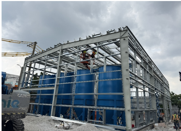
Photo 4: View facing northwest. CAC bolting up new steel building components.
