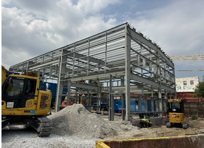
Photo 1: View facing southwest. View of imported DGA as CAC preps trench north of building for backfill.
