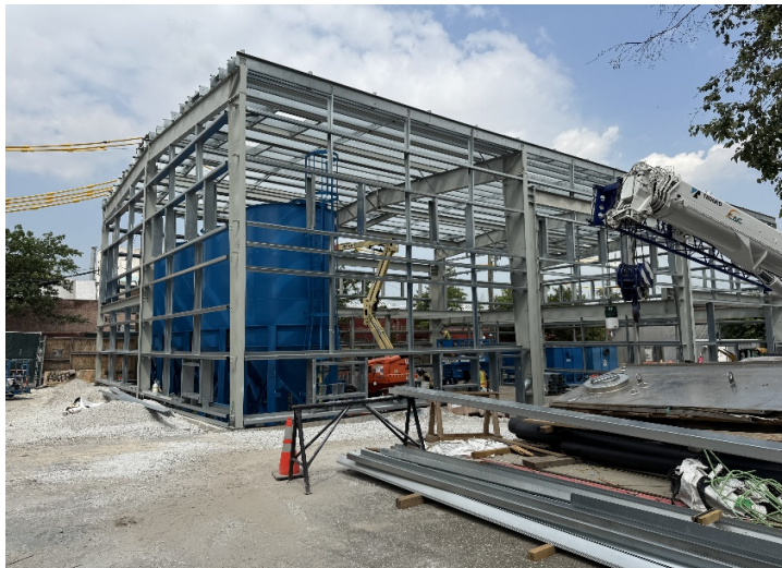
Photo 2: View facing northwest. CAC bolting up new steel building components.
