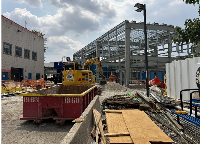
Photo 3: View facing southwest. CAC backfilling trench north of building footprint.
