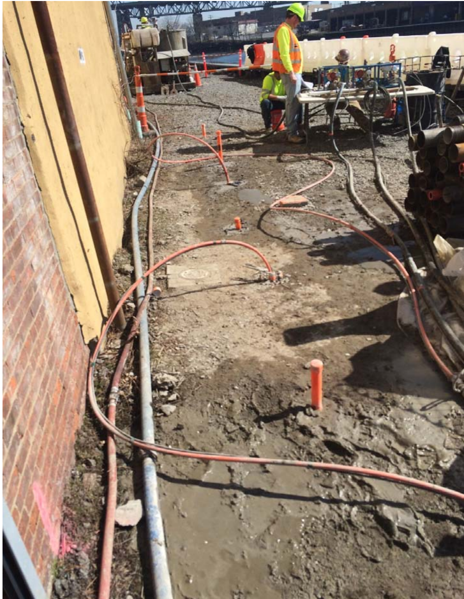
Photo 12: Hoses injecting grout in TAM-13 and TAM-15, March 9, 2016
