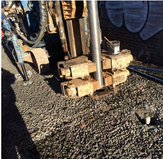
Photo 6: Drilling for TAM pipe installation, March 3, 2016
