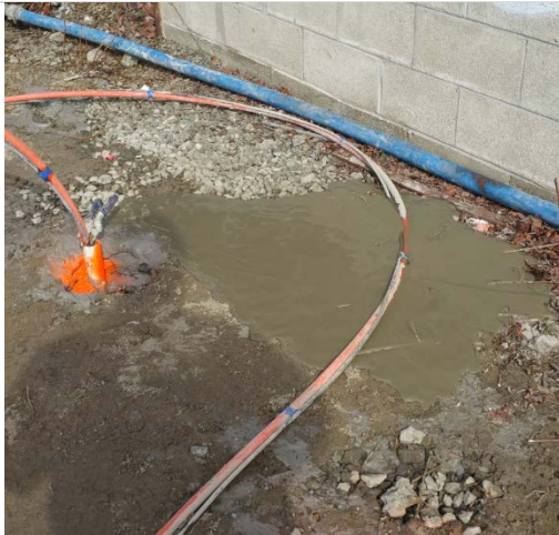
3/09/16 - Grout return to surface during injection.
