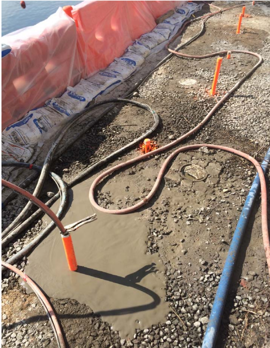
Photo 10: Looking west, hoses injecting grout in TAM-12, March 8, 2016
