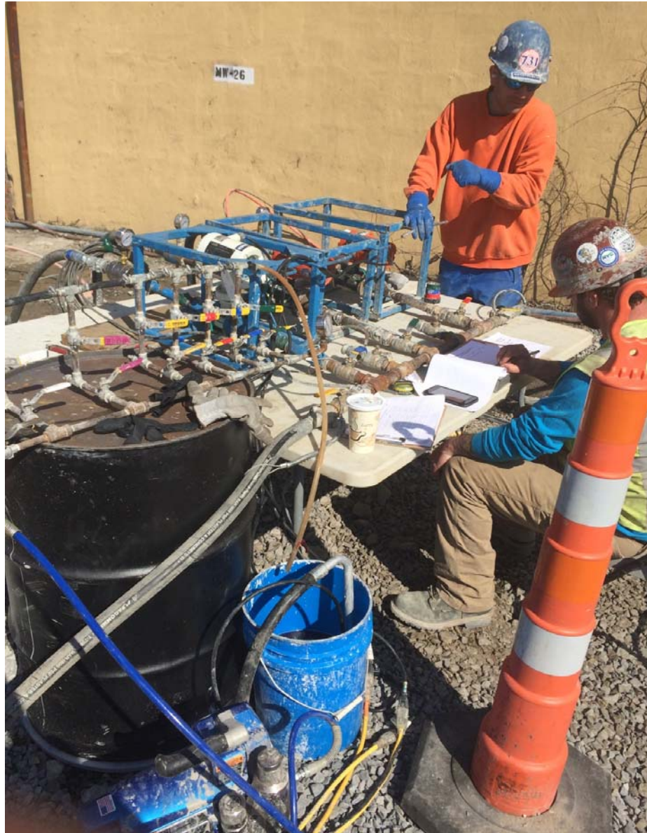
Photo 11: Grout manifold and monitoring set up, March 9, 2016
