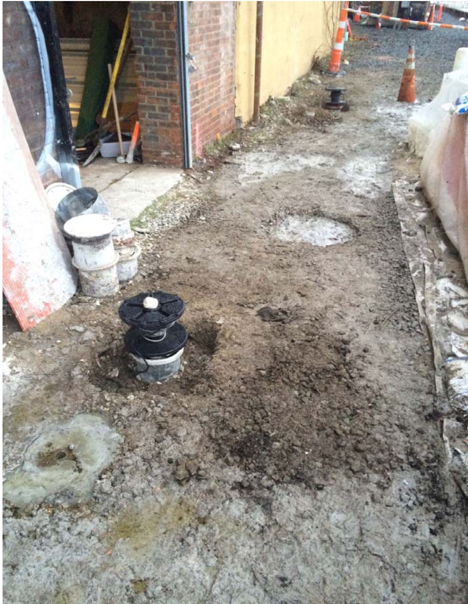
Photo 16: Looking east, image of abandoned wells and newly installed piezometers, March 14, 2016
