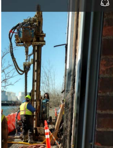
3/2/16- PVC pipe installation into borehole
