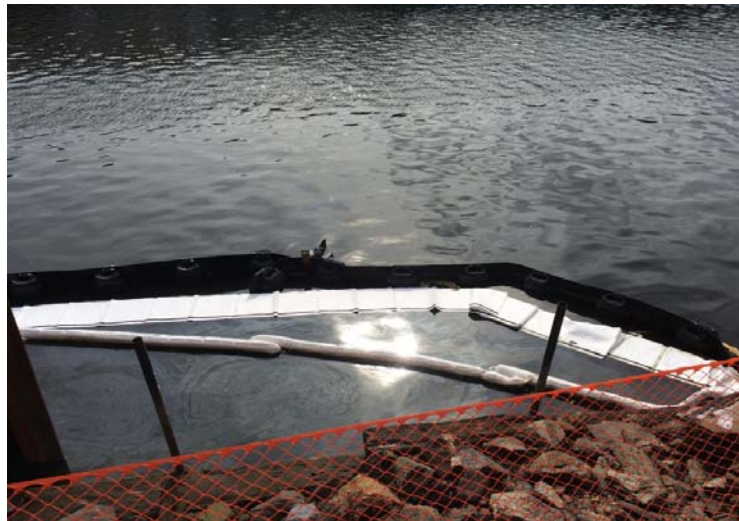
Photo 9: Looking south, view of Newtown Creek with absorbent boom, absorbent pads and PVC hard boom around work area, March 4, 2016
