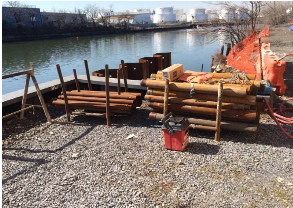
Photo 2: Looking southwest, drill casings for TAM pipe installation, March 1, 2016
