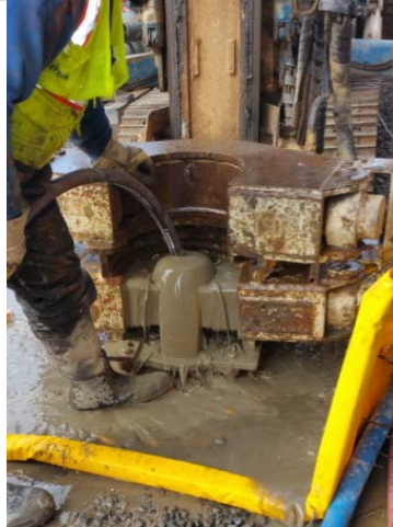
3/2/16- Grouting borehole.
