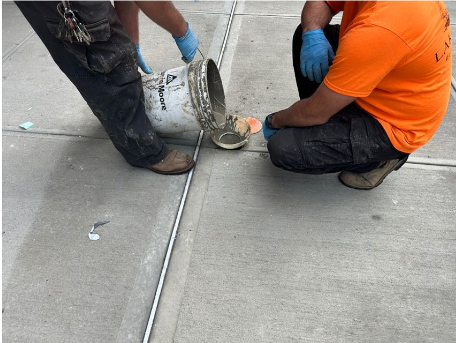
Photo 1: View of Lakewood Environmental Services Corp. (Lakewood) decommissioning monitoring well MW-4, facing southeast. (Taken on 5/8/2024).
