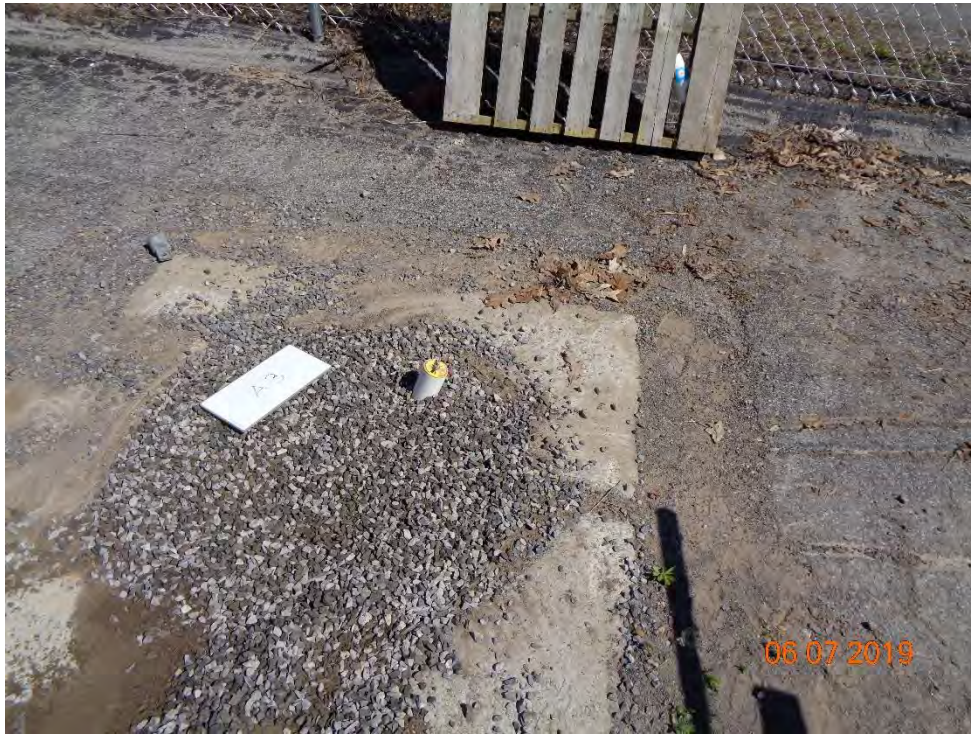
Photo 75 - View of A3 after refilling manhole with stone
