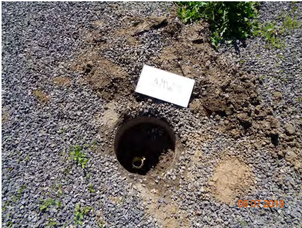
Photo 76 - View of AMW8 prior to extending and backfilling
