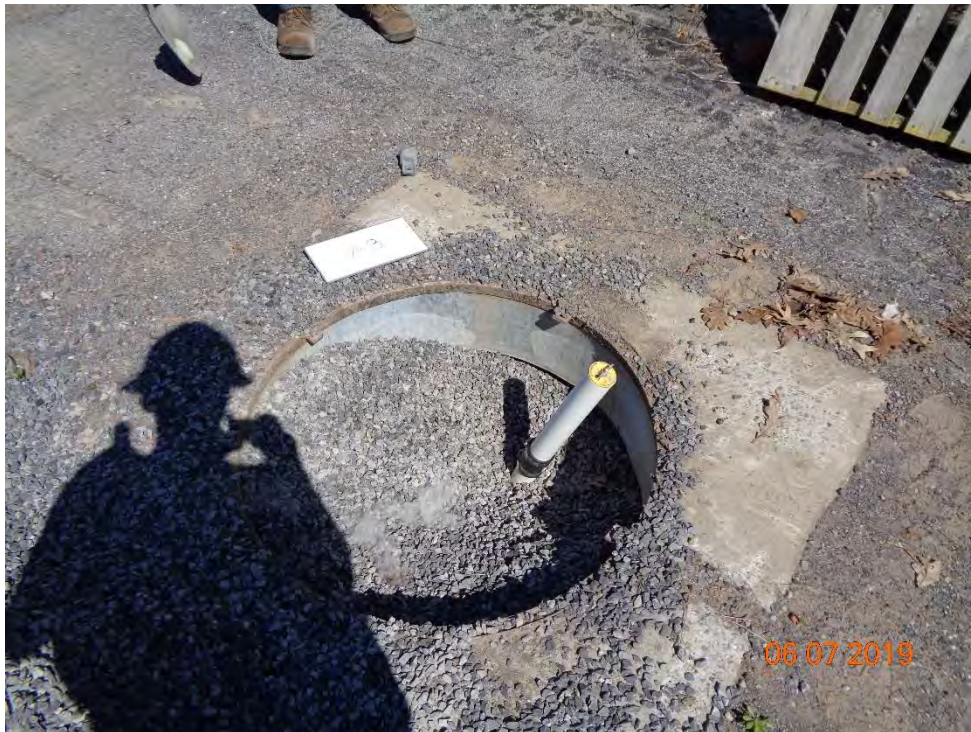
Photo 74 - View of A3 after extending and prior to refilling manhole
