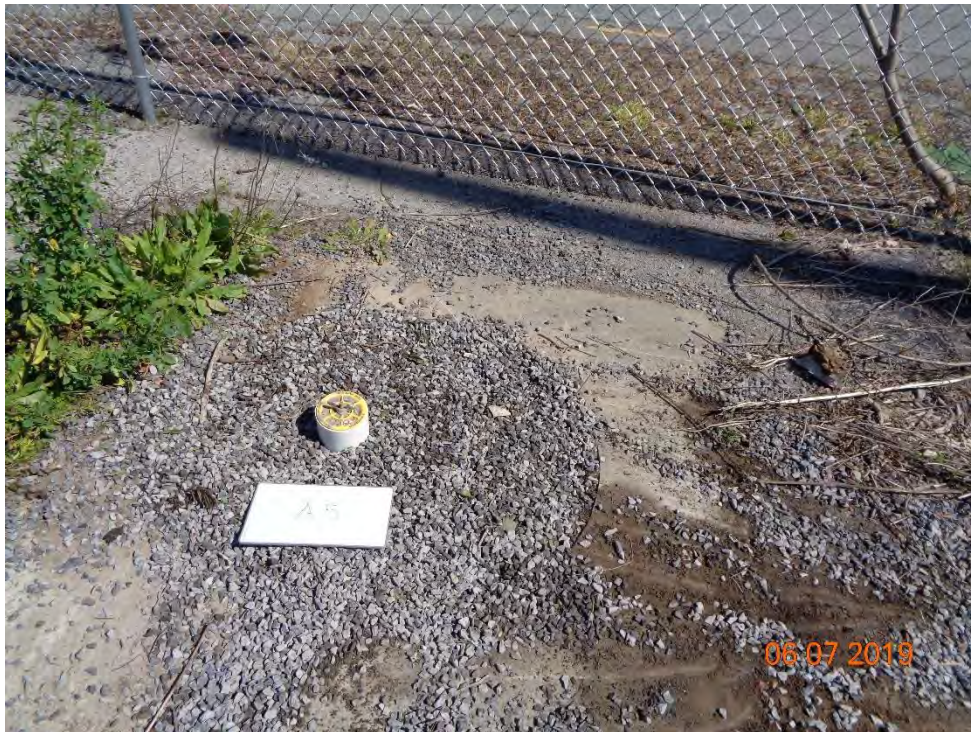
Photo 72 - View of A5 after refilling manhole with stone
