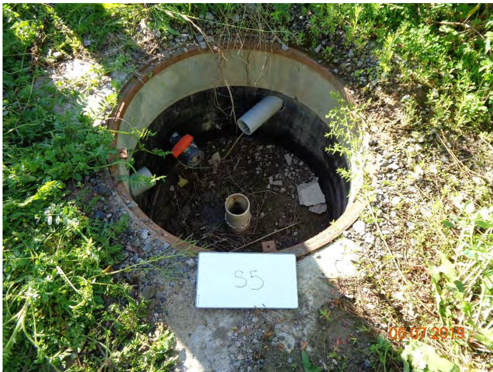
Photo 62 - View of S5 prior to extending and backfilling manhole
