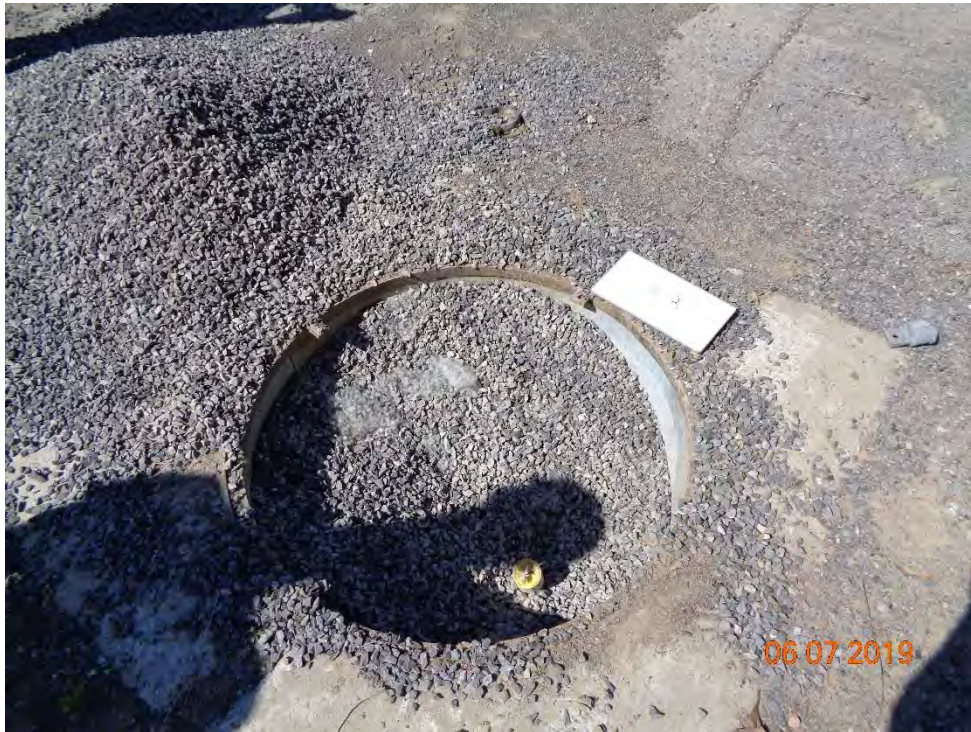
Photo 73 - View of A3 prior to extending and refilling manhole
