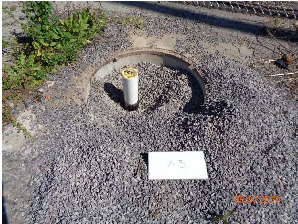
Photo 71 - View of A5 after extending and prior to refilling manhole
