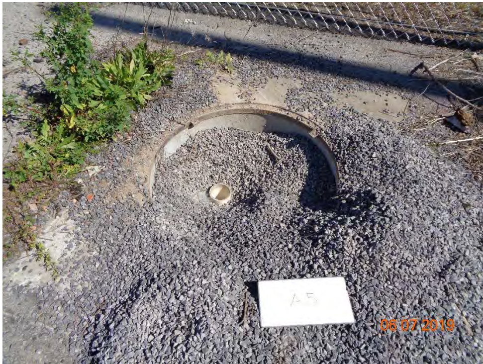
Photo 70 - View of A5 prior to extending and refilling manhole
