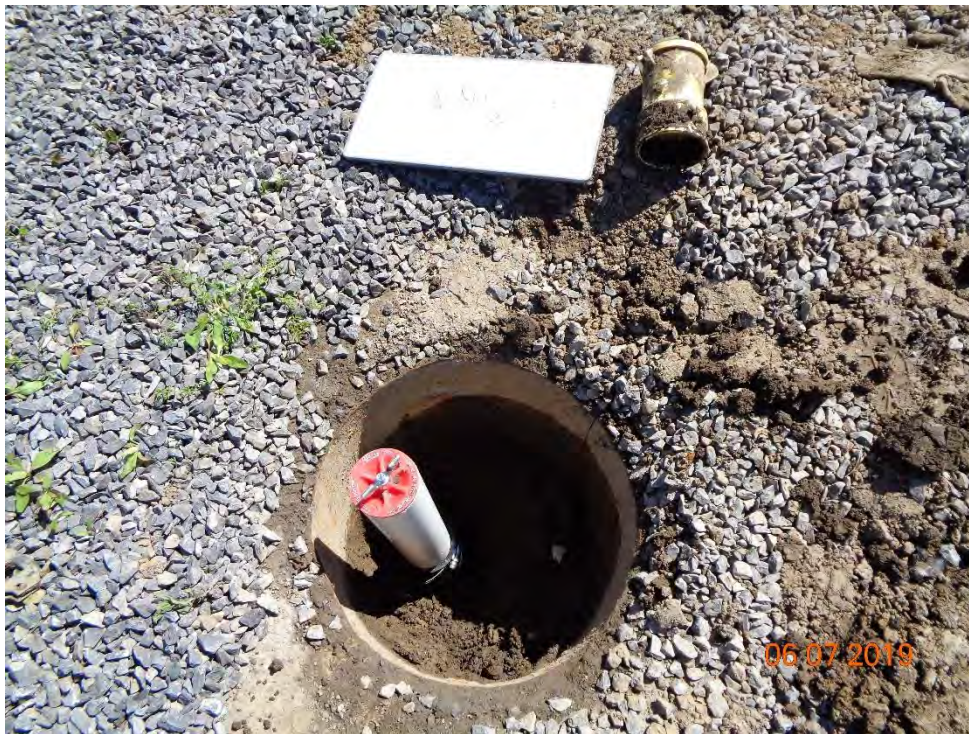
Photo 77 - View of AMW8 after extending and prior to backfilling (note slip cap piece removed from well casing prior to extending)
