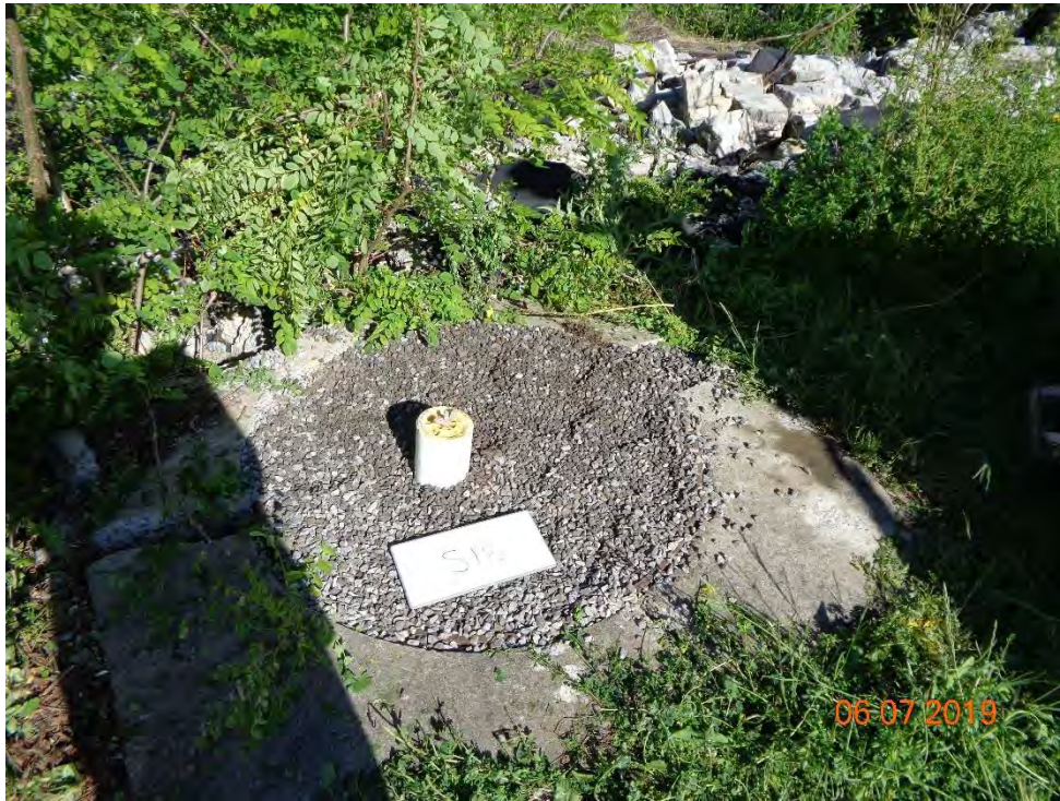
Photo 67 - View of S18 after backfilling manhole with stone
