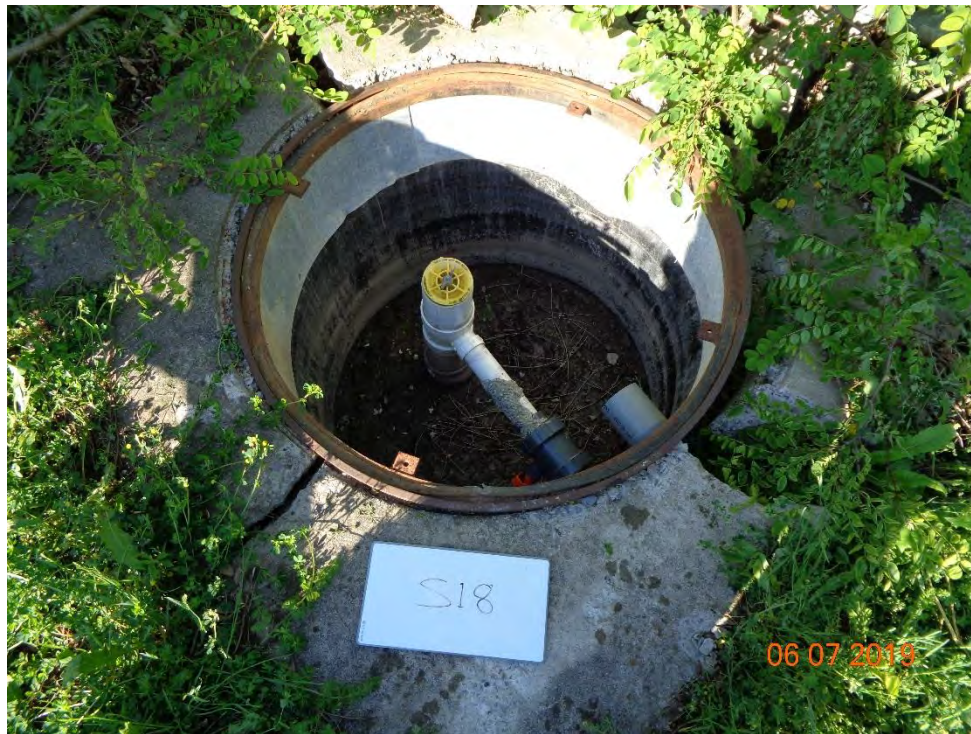
Photo 65 - View of S18 prior to extending and backfilling manhole
