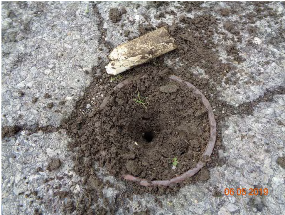
Photo 37 - View of Northern Terminal CT4, close-up of broken casing
