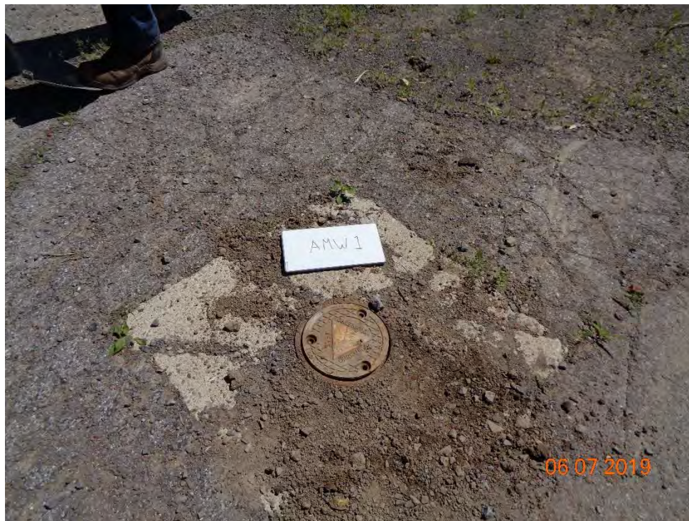
Photo 80 - View of AMW1 after placing salvaged cover from dislodged casing of PZ104D
