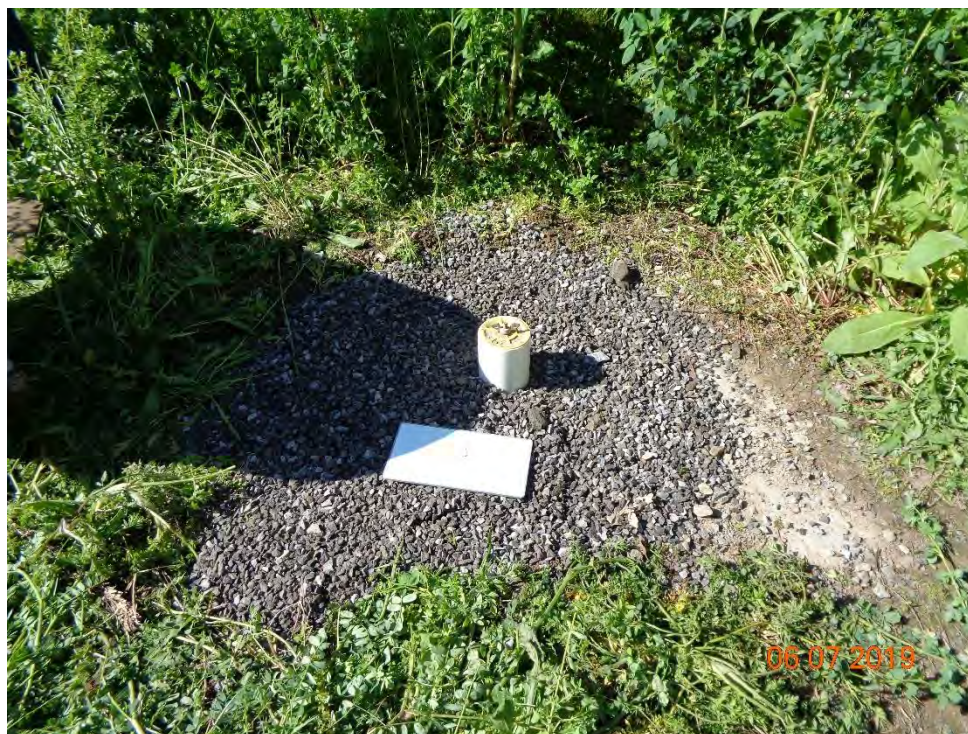
Photo 64 - View of S5 after backfilling manhole with stone
