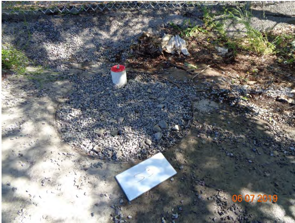
Photo 69 - View of S3 after refilling manhole with stone
