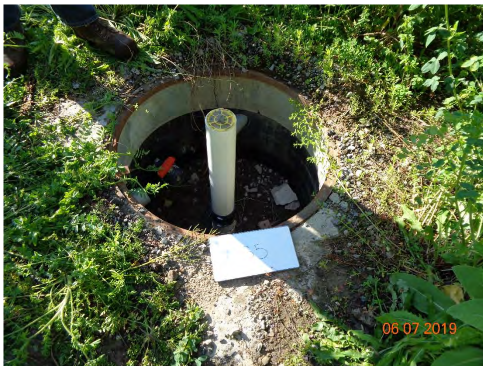
Photo 63 - View of S5 after extending and prior to backfilling manhole
