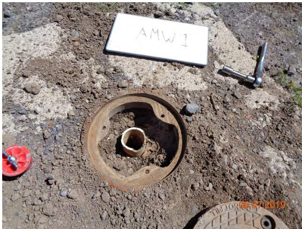
Photo 79 - View of AMW1 after cutting down broken PVC casing
