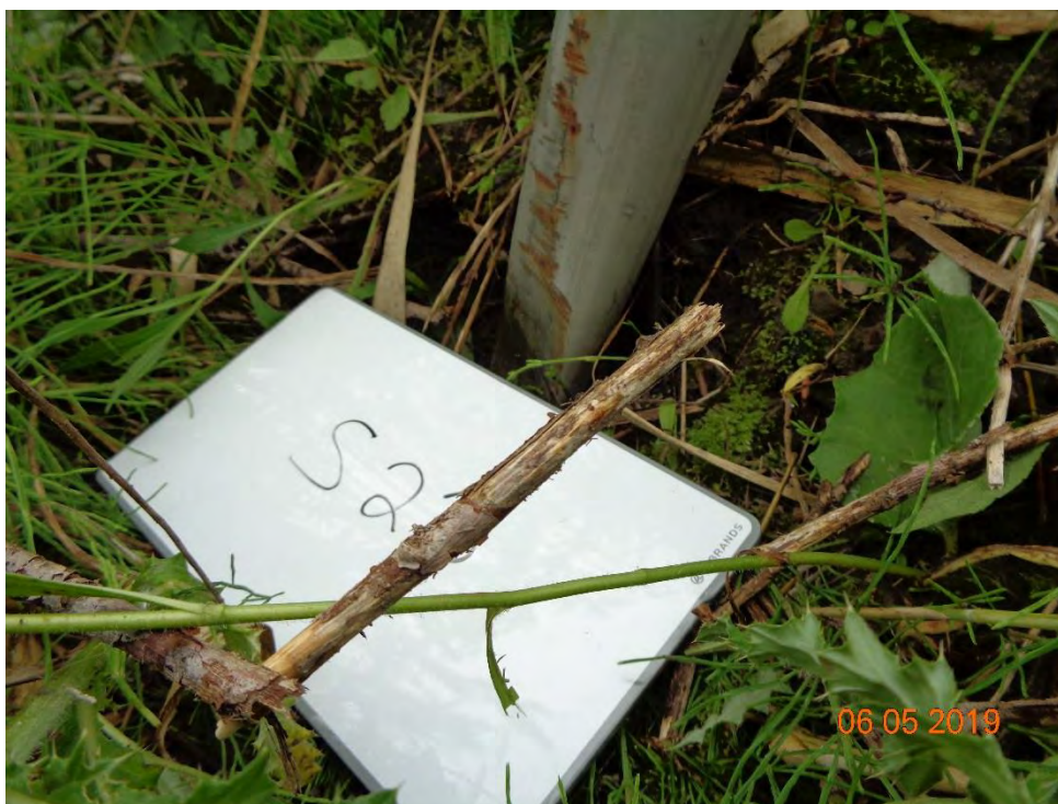
Photo 47 - View of S23, close-up of crushed casing
