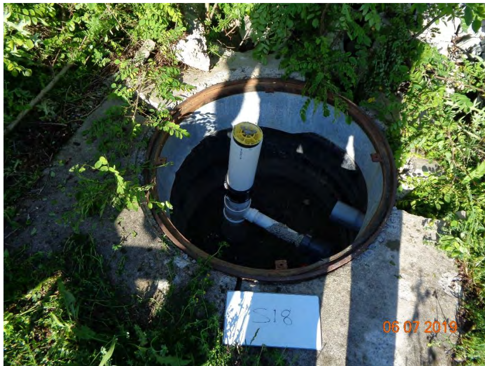
Photo 66 - View of S18 after extending and prior to backfilling manhole
