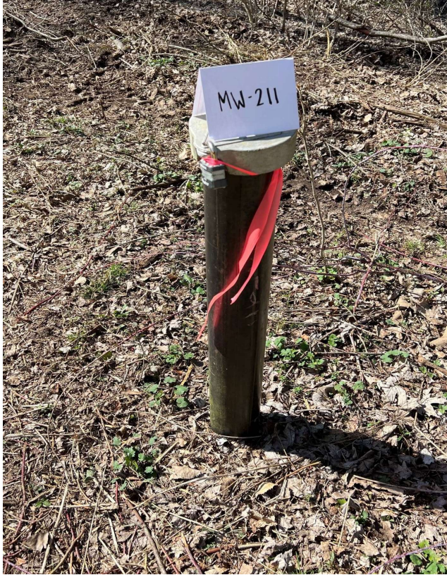
Photograph No. 27: MW-211 Pre abandonment 04/12/2023
