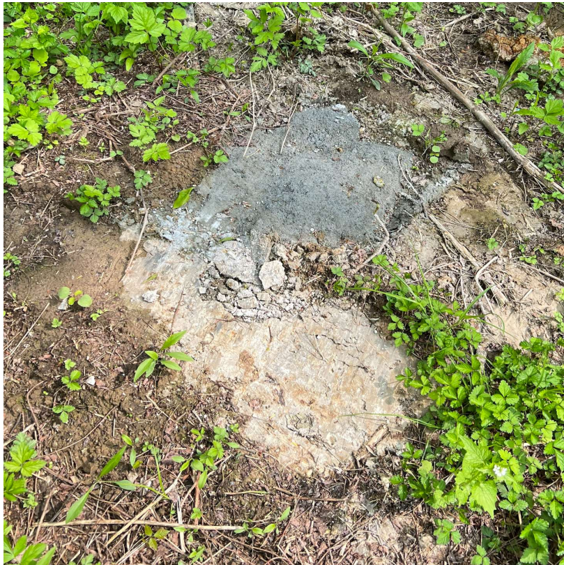
Photograph No. 16: MW-203 Post abandonment 05/09/2023
