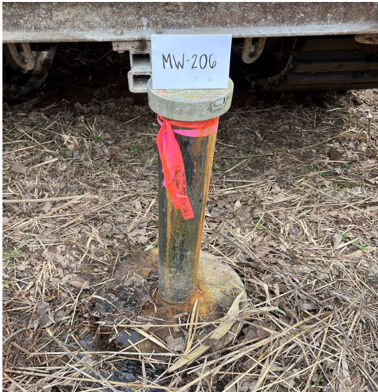
Photograph No. 19: MW-206 Pre abandonment 04/11/2023
