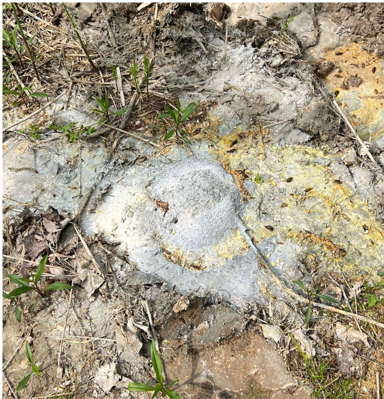
Photograph No. 20: MW-206 Post abandonment 05/09/2023
