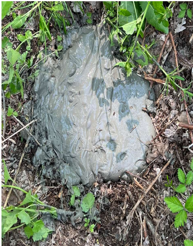
Photograph No. 28: MW-211 Post abandonment 05/09/2023
