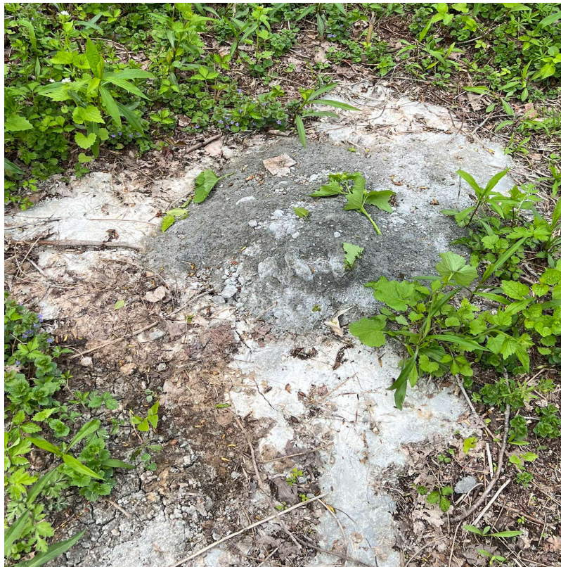
Photograph No. 14: MW-202 Post abandonment 05/09/2023
