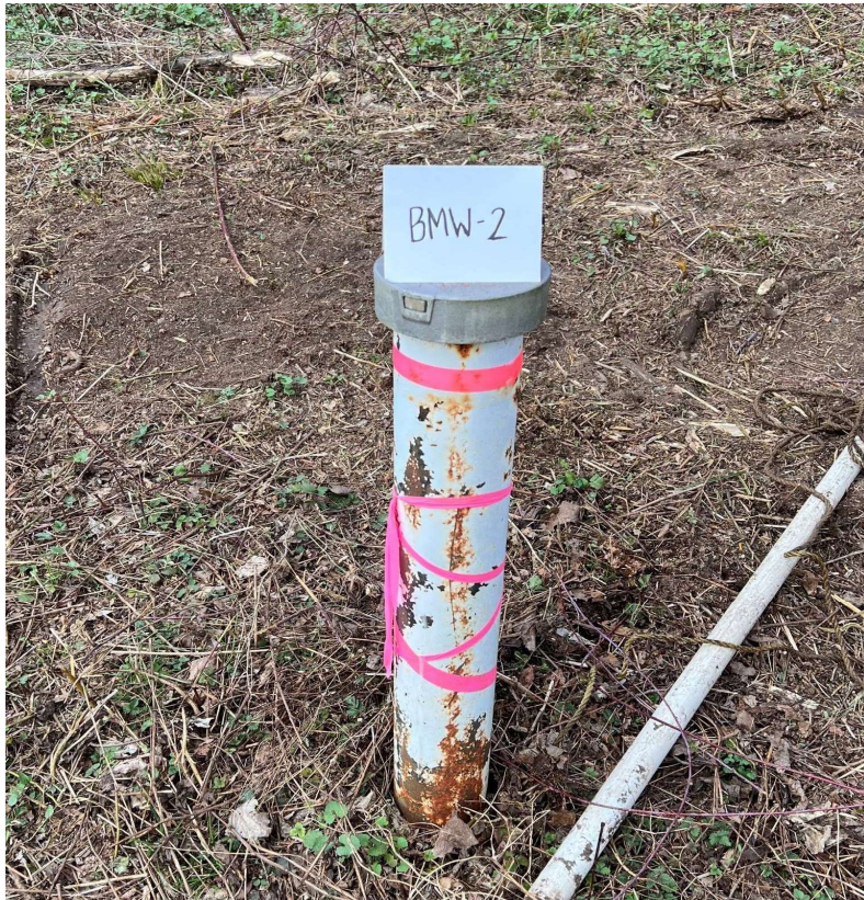
Photograph No. 1: BMW2 Pre abandonment 04/12/2023
