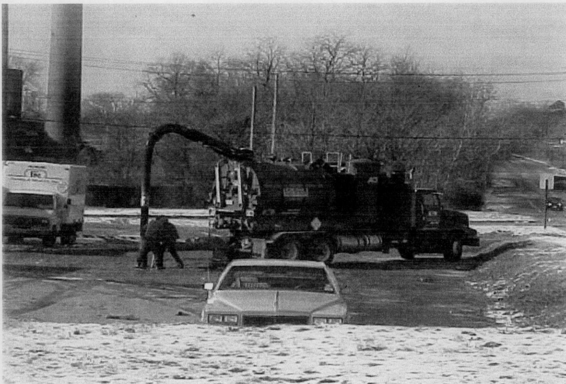
3. View of the vactor truck utilized during remediation.
