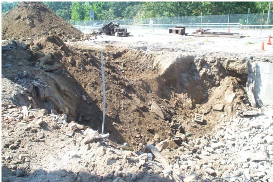
4. Excavation of PCE-contaminated soil at former repair bays (looking southwest)
