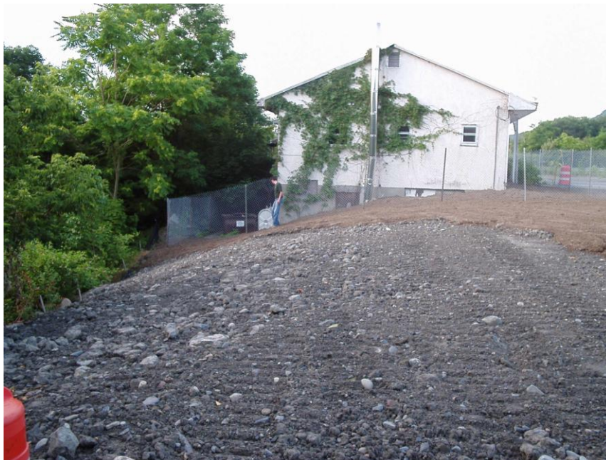
10. Installation of final soil barrier layer at eastern portion of Site
