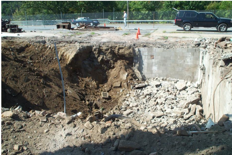
3. Excavation of PCE-contaminated soil at former repair bays (looking west)
