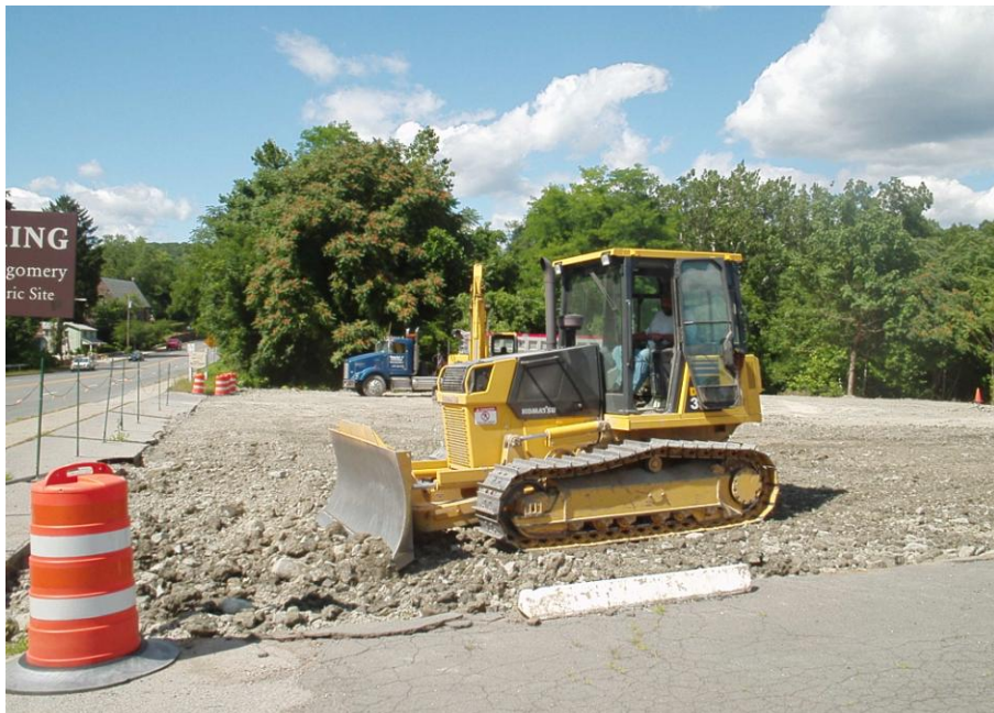
9. Installation of final soil barrier layer at western portion of Site
