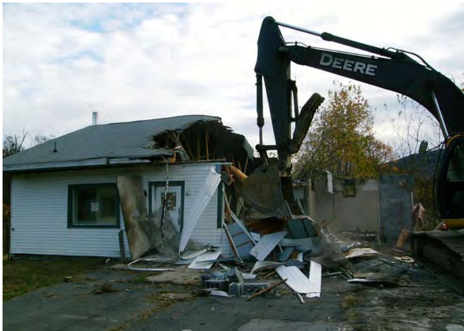
2. Demolition of the northern portion of the building.
