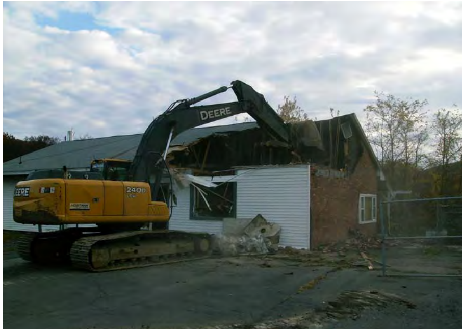
1. Initial building demolition activities.
