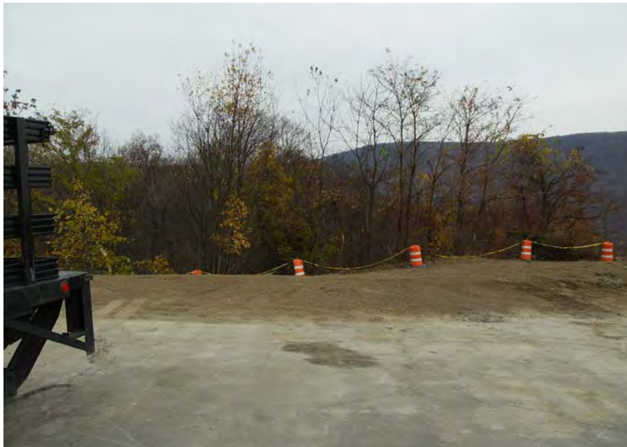
7. Area of former on-site building following Site restoration.
