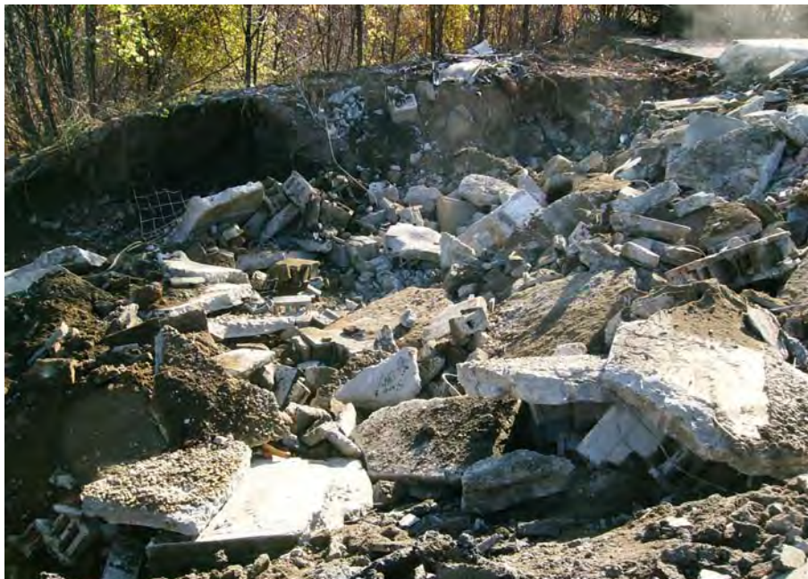
6. Demolition debris consisting of concrete block and foundation.
