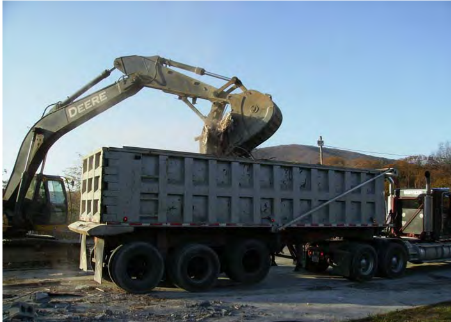
5. Loading of demolition debris for off-site disposal.
