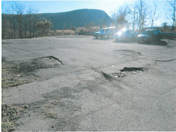
Looking South East
