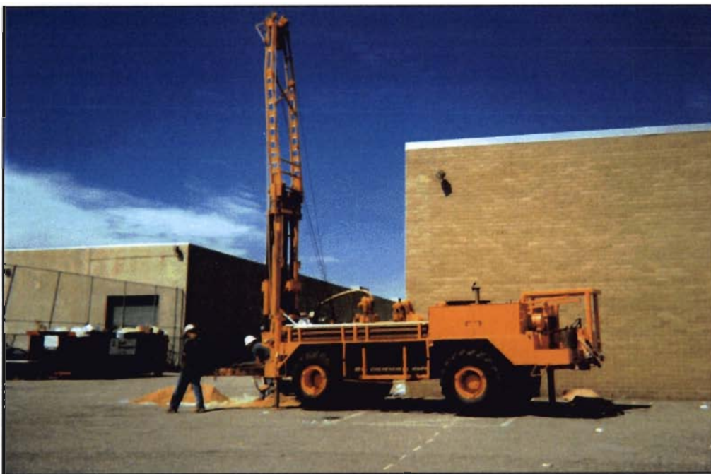
Hollow-stem auger drill rig used for the temporary well points.
