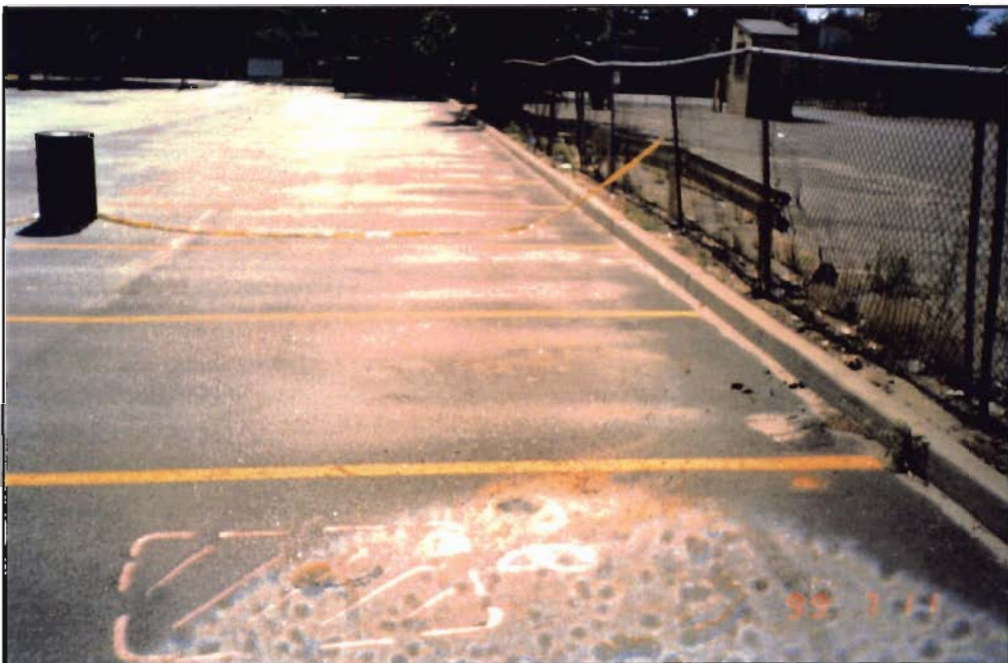
SB-008 was used to evaluate subsurface conditions adjacent to a historic catch basin and down gradient of a historic leaching pool.
