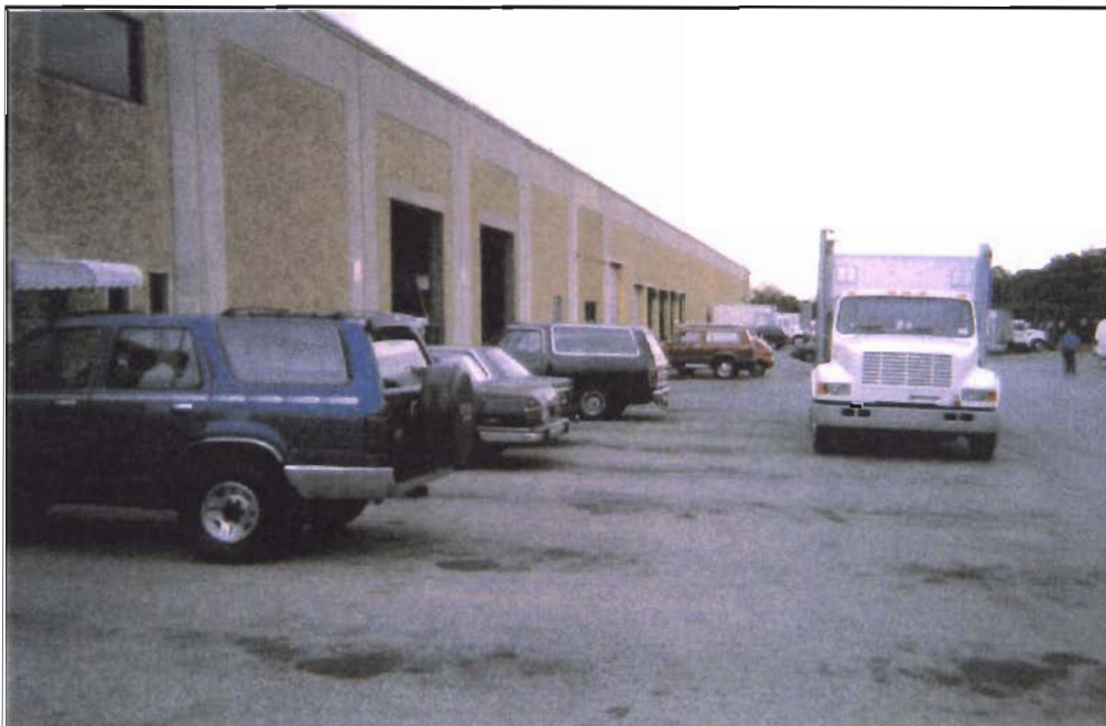
Several truck bays are located on the south side of Magazine Distributors.
