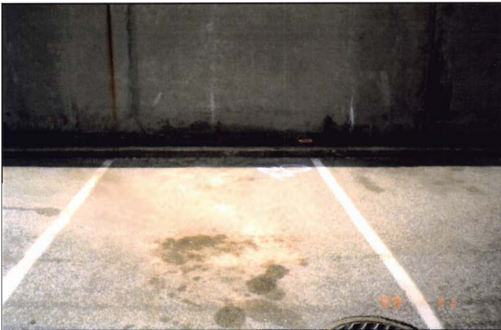
SB-022 was used to evaluate subsurface conditions near a historic inlet/leaching pool.
