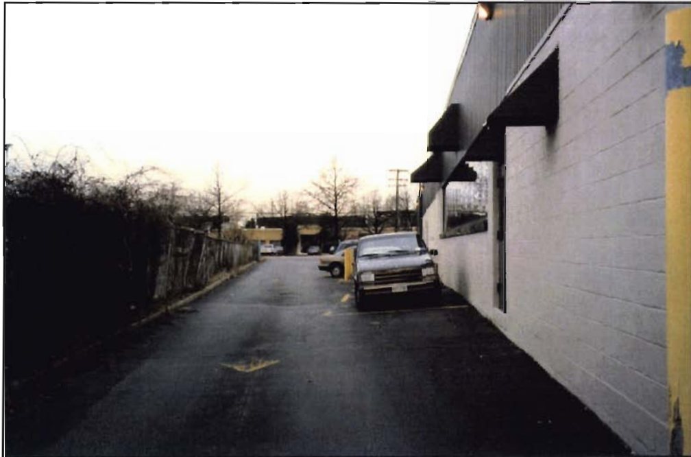
South side of Air Techniques.
