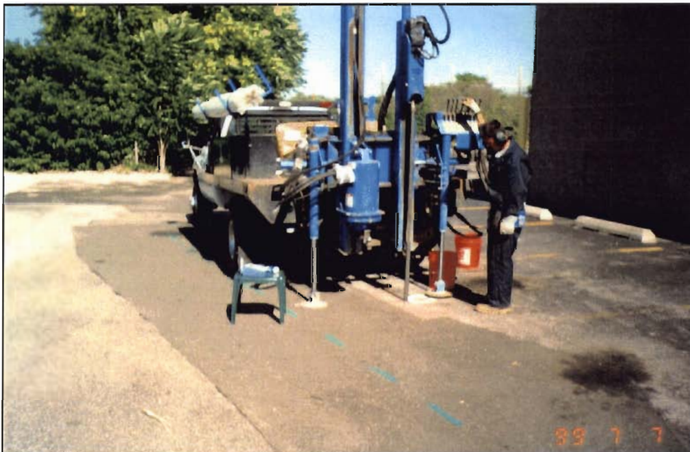
The Hurricane Drill Rig.
