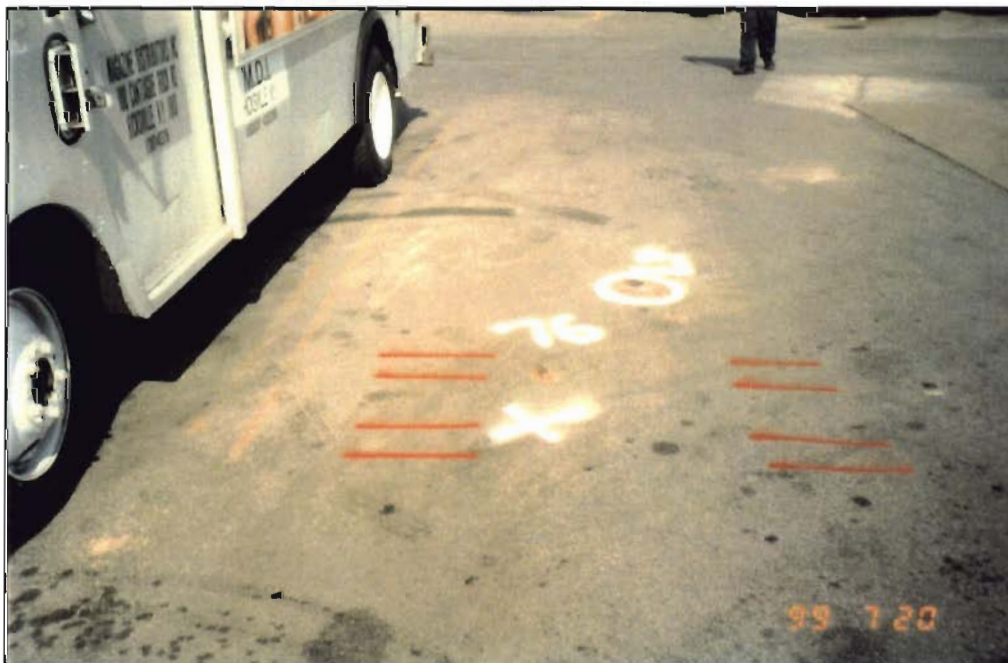
SB-076 was used to evaluate subsurface conditions associated with a historic leaching pool (Magazine Distributors).
