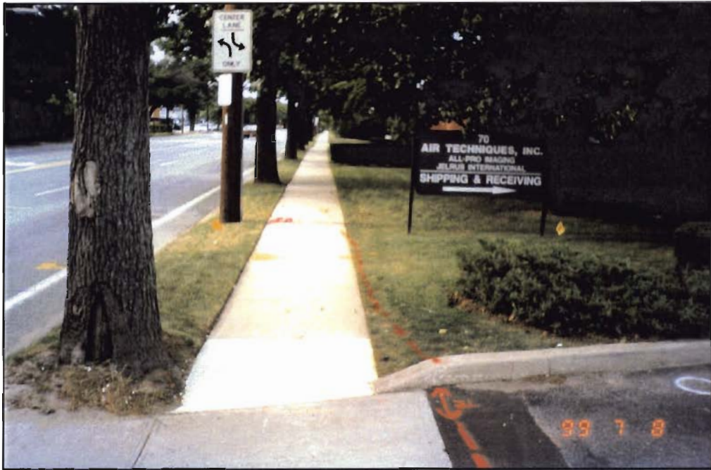
Picture illustrating the utility markouts in front of Air Techniques.
