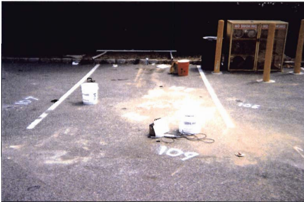
SB-105 through Sb-109 were used to evaluate subsurface conditions associated with elevated radioactivity and VOCs found at approximately 9 feet below grade during the installation of TW-02.
