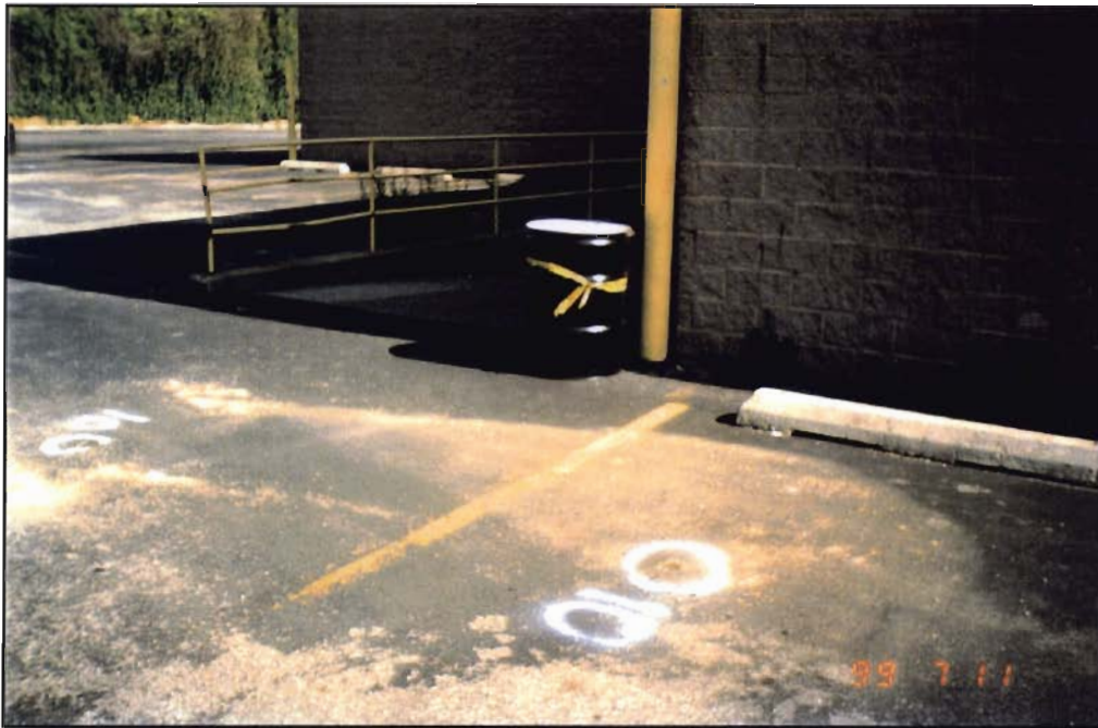
SB-010A & B were used to evaluate subsurface conditions associated with former Recharge Basin #4. Refusal was encountered in boring 10A therefore boring 10B was advanced (Air Techniques, Inc.).
