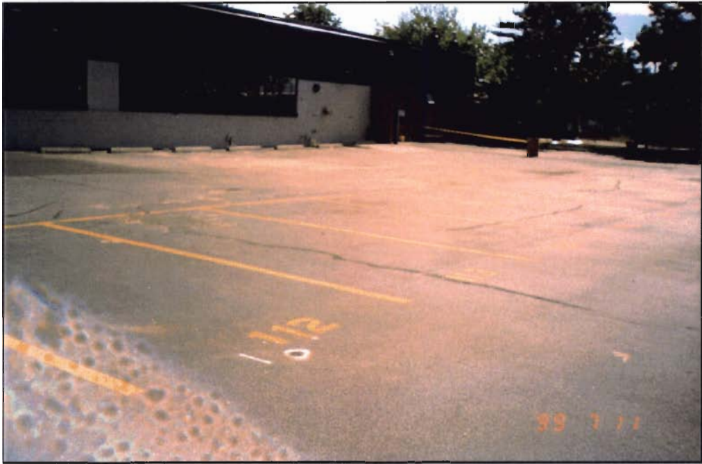
SB-001 was installed on the north side of the Air Techniques Building to penetrate the footprint of the former the Special Nuclear Material Storage #1 Building.
