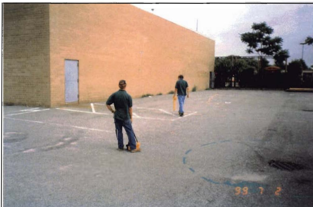
NAEVA personnel marking the underground utilities and other objects at the rear of Gilbert Displays.
