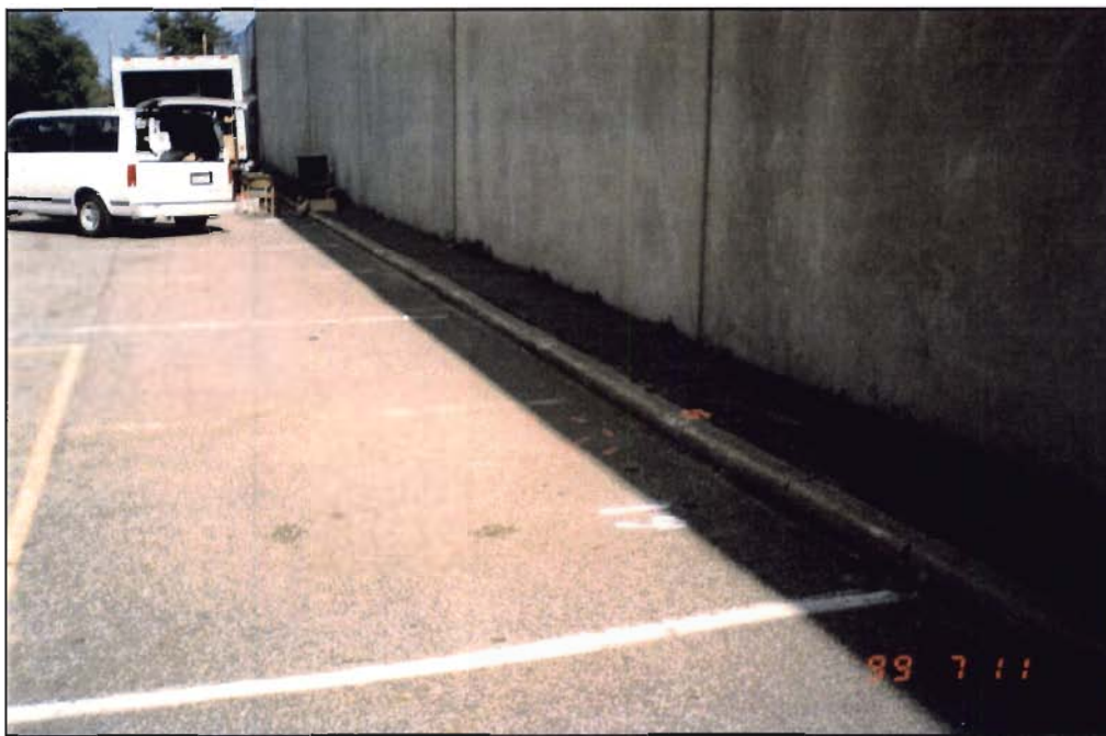
SB-019 was used to evaluate subsurface conditions adjacent to a historic leaching pool.
