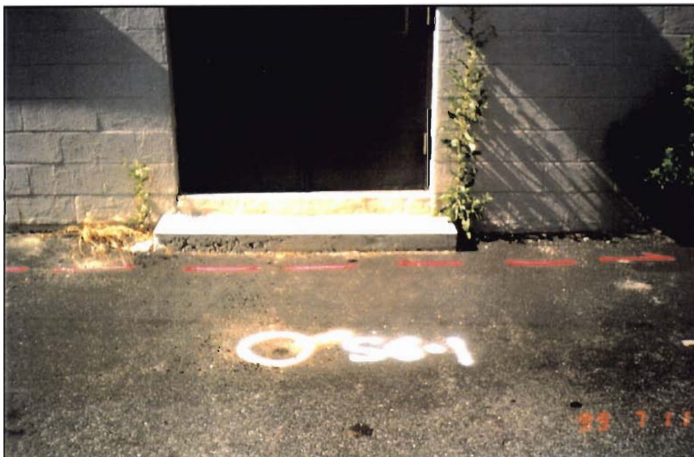
SG-01 was installed at the request of NYSDEC to evaluate the area for BTEX compounds.
