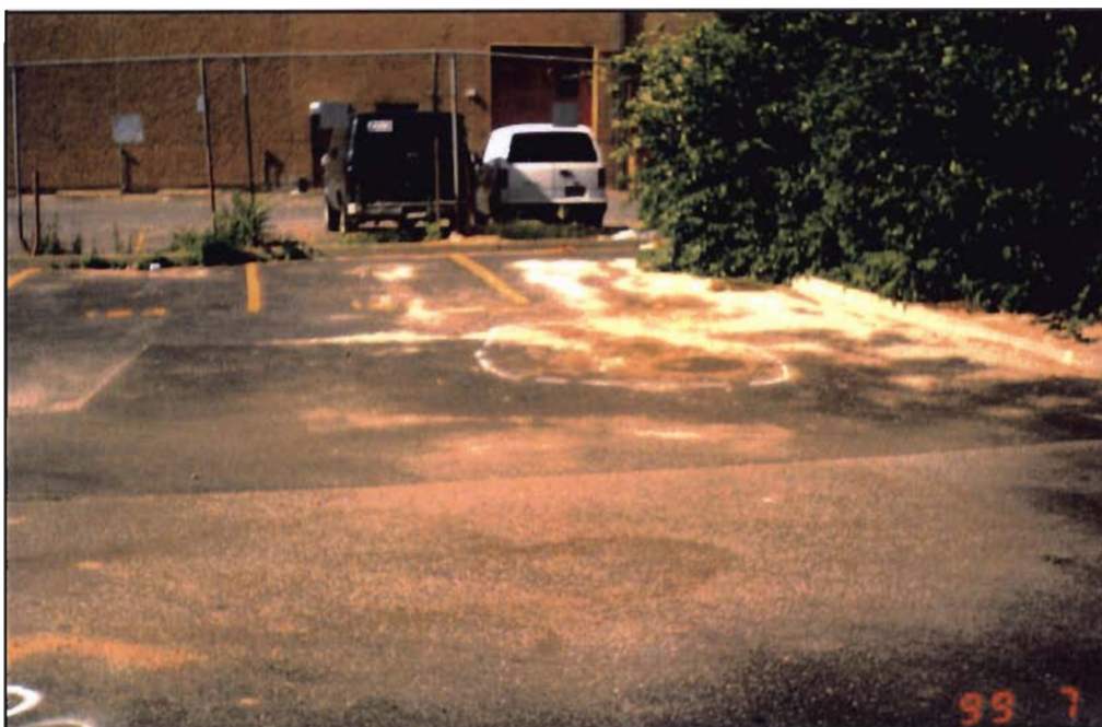
Many of the borings were located within close proximity (i.e. SB-009 and SB-010).
