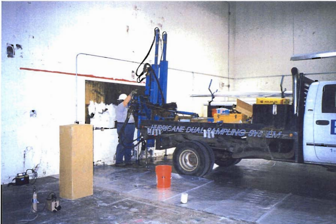
Hurricane Geoprobe Rig (inside the former Gilbert Displays Building).
