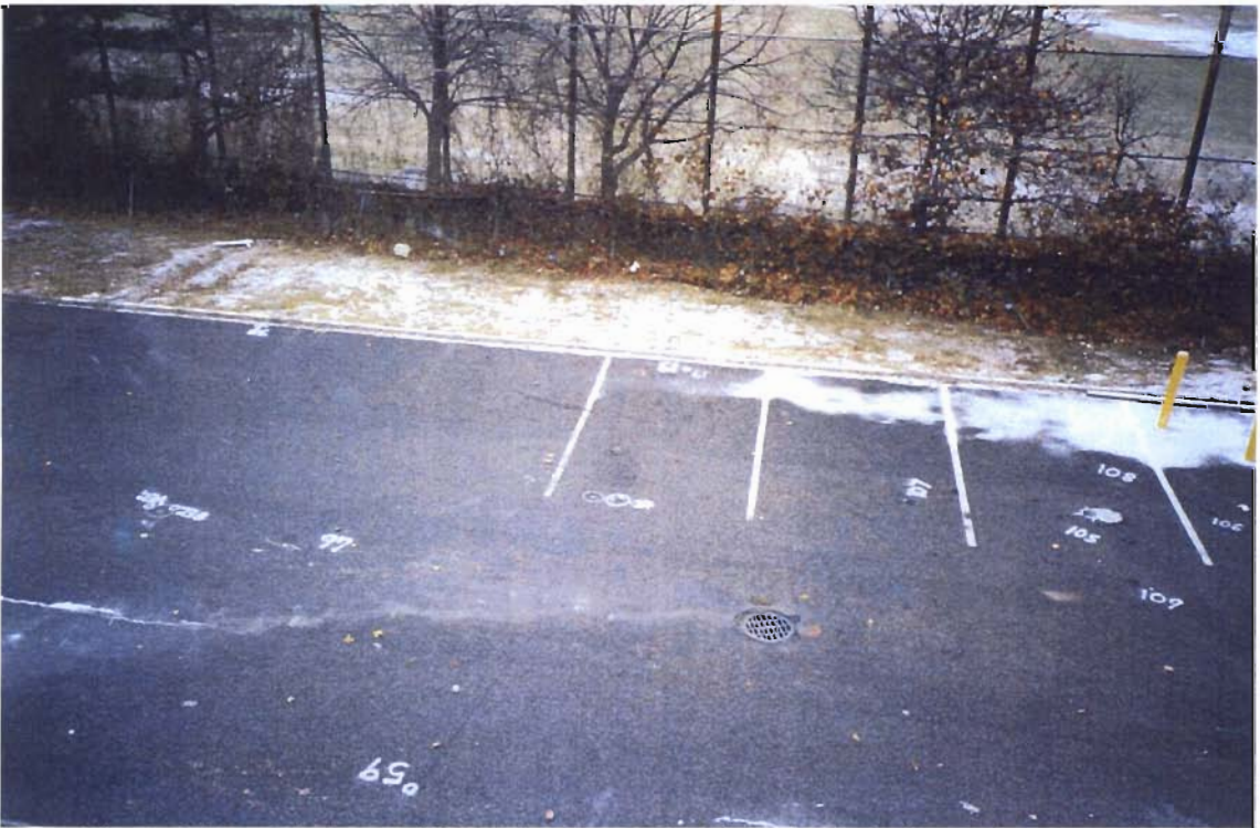
Rear of former Gilbert Displays Building (view from roof) Orientation is further south compared to the previous picture.
