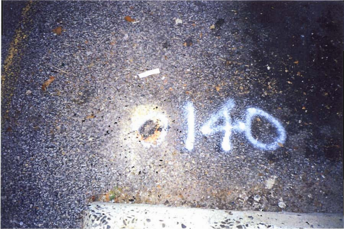
Soil boring SB-140 was installed near the historic transformer pad at Magazine Distributors.
