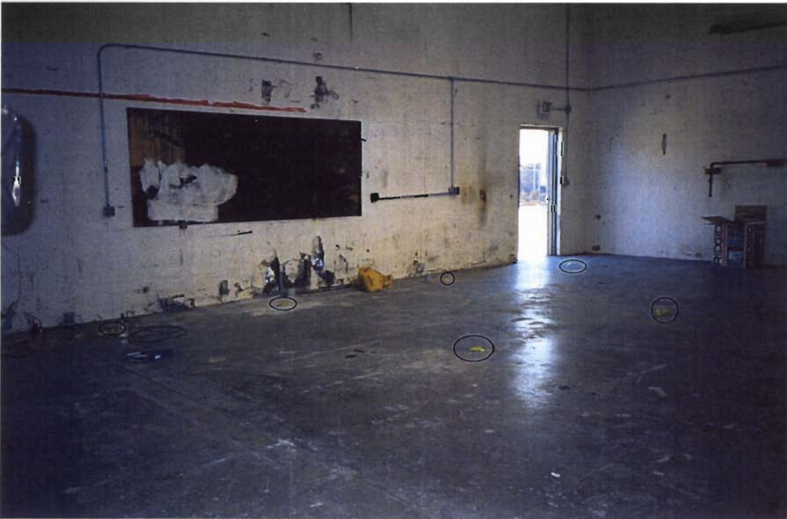
Inside of former Gilbert Displays Building. Soil boring SB-119, SB-120, SB-121, SB-124, SB-125, and SB-126 were installed in this area.
