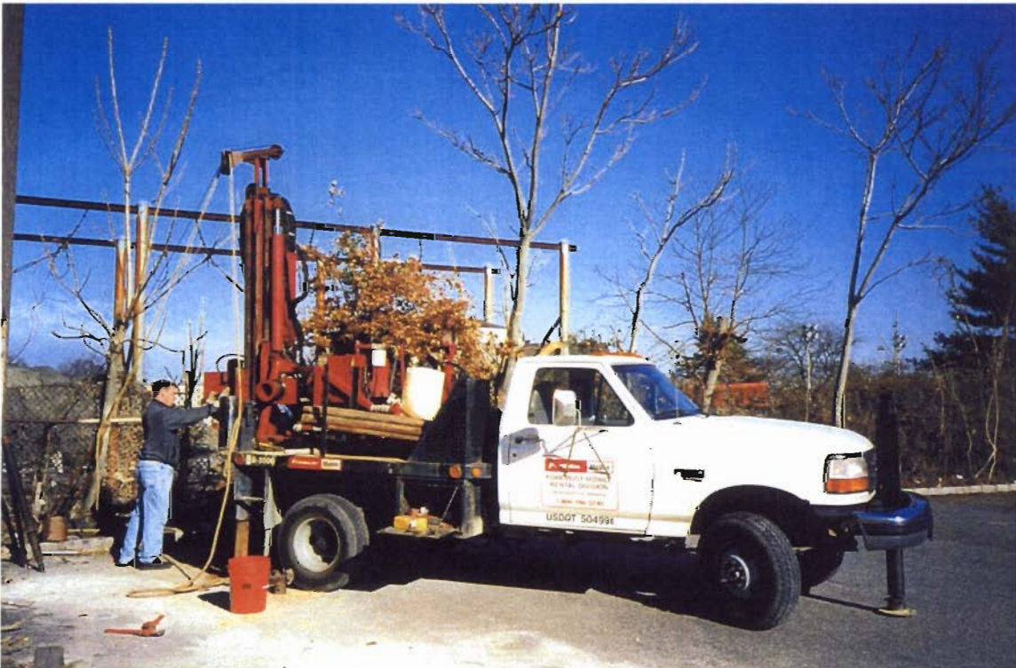
Geotechnical drill rig. Two geotechnical borings were advanced adjacent to the former Gilbert Displays Building. View of GT-1.
