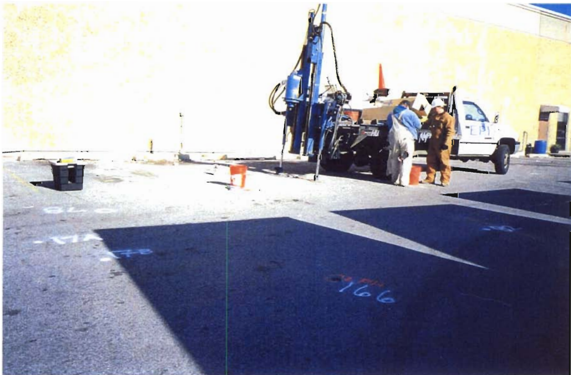
Soil boring SB-166 was advanced to investigate an historical leaching pool south of Magazine Distributors. Note air monitoring equipment housed in tote.
