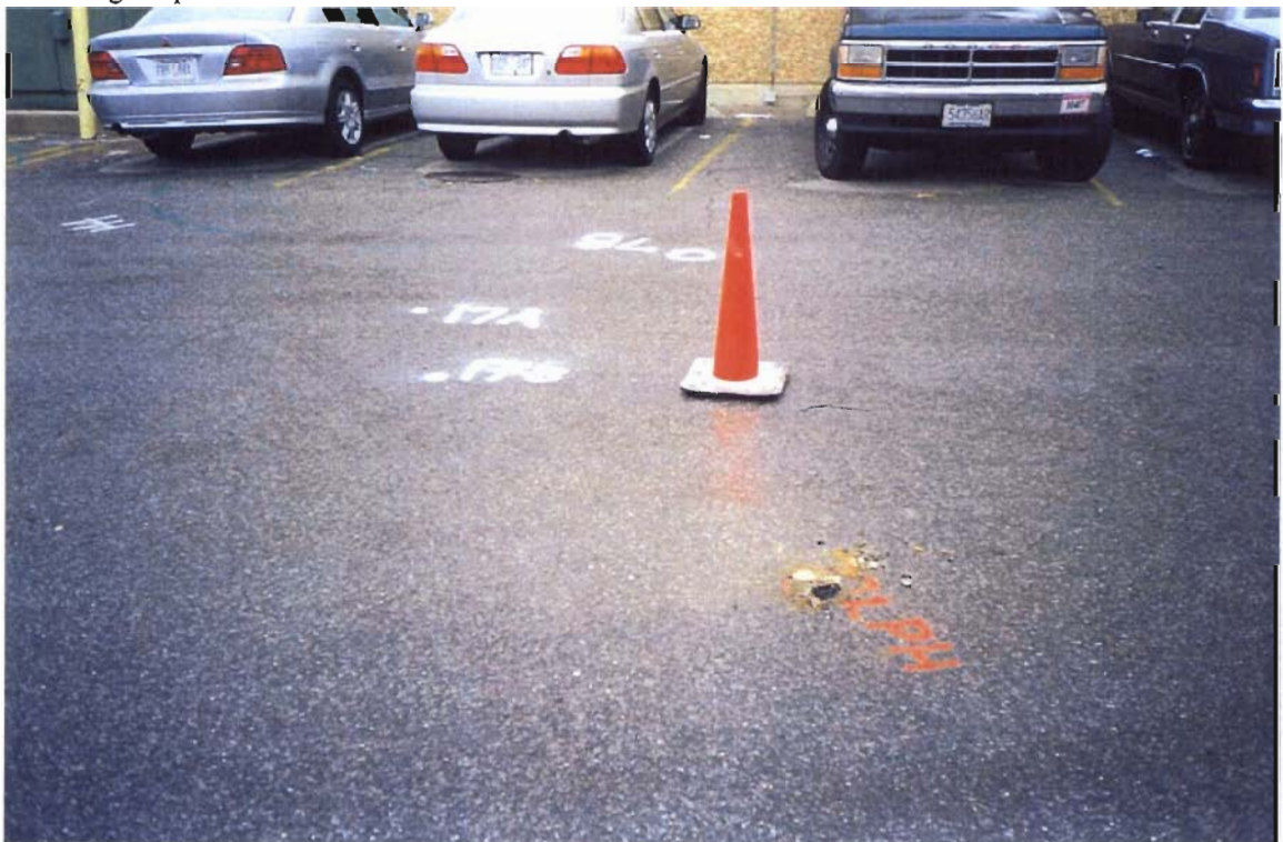
Soil boring SB-145 was placed south of Magazine Distributors to investigate an historic leaching pool.
