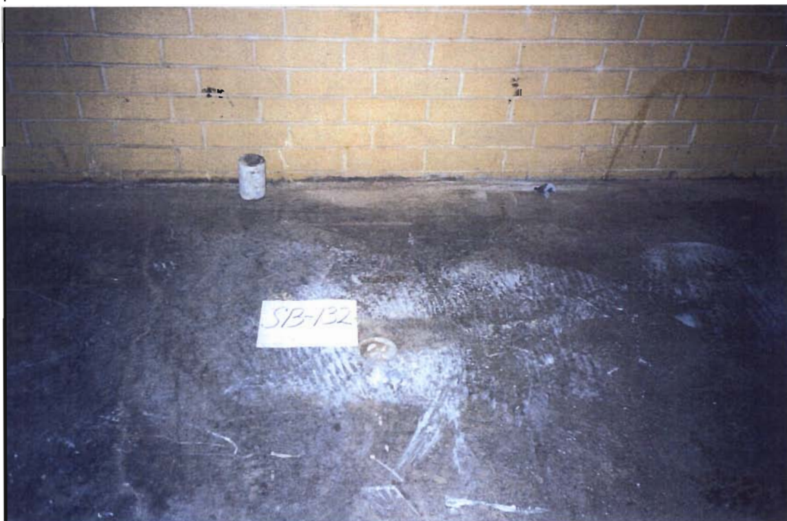
Soil boring SB-132 was added to the scope to determine whether the increase in surface radiation was a result of the proximity to the brick wall.
