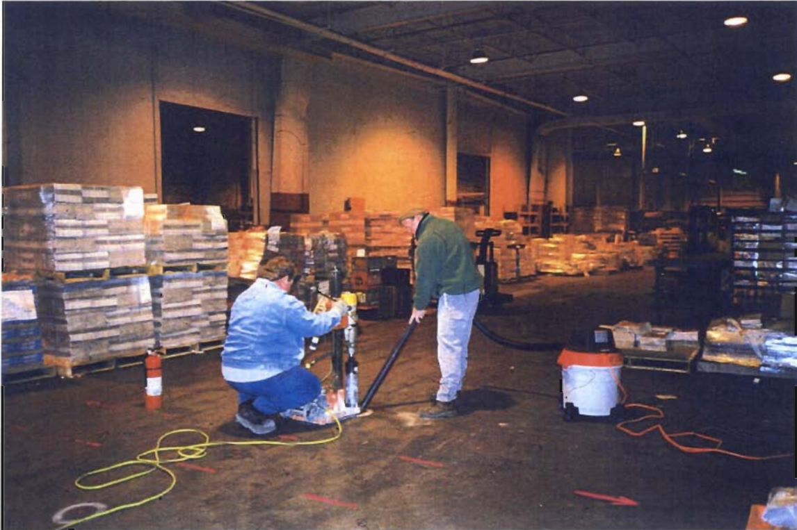
Coring the floor at Magazine Distributors.
