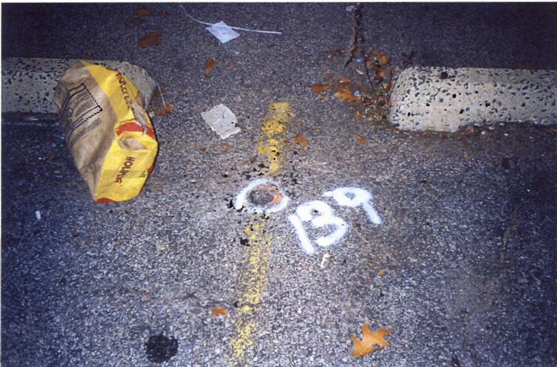
Soil boring SB-139 was installed near the historic transformer pad on Magazine Distributors.
