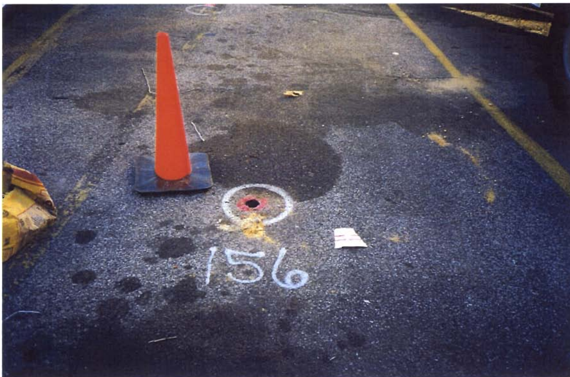
Soil boring SB-156 was advanced to further define SB-064 (southeast of the former reservoir).
