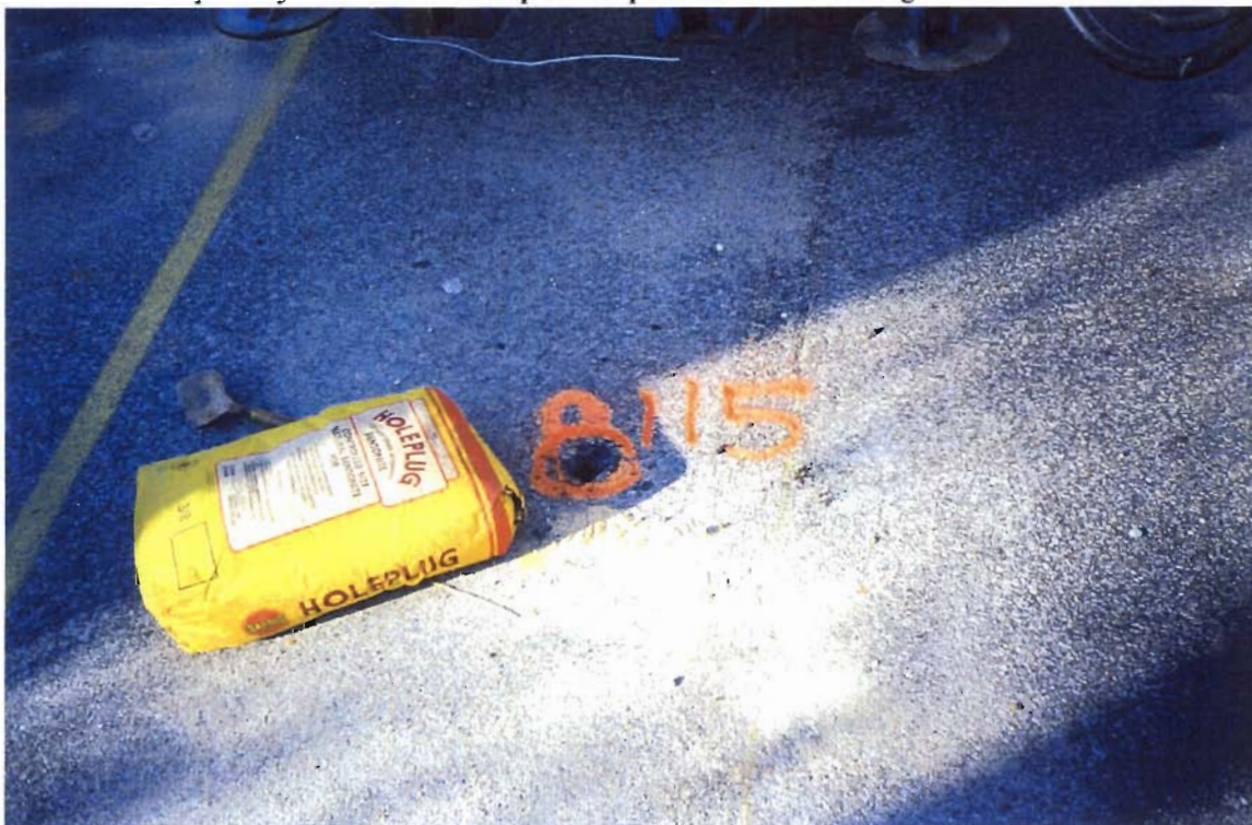
Soil boring SB-115 was advanced to evaluate the potential presence of process residuals at Magazine Distributors.
