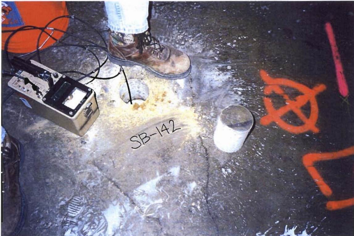
Soil boring SB-142 was located inside Magazine Distributors to investigate an historic leaching pool.
