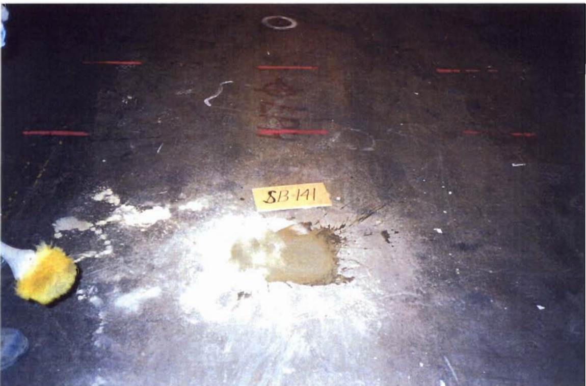
Soil boring SB-141 was installed inside Magazine Distributors to investigate an historic leaching pool.
