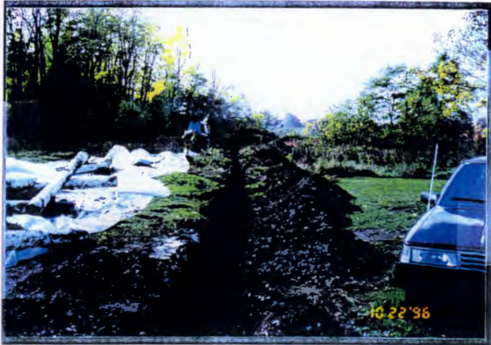
Drain line excavation facing discharge point excavation
