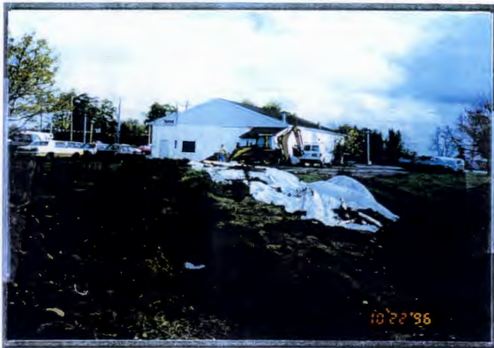
Drain line excavation facing building structure
