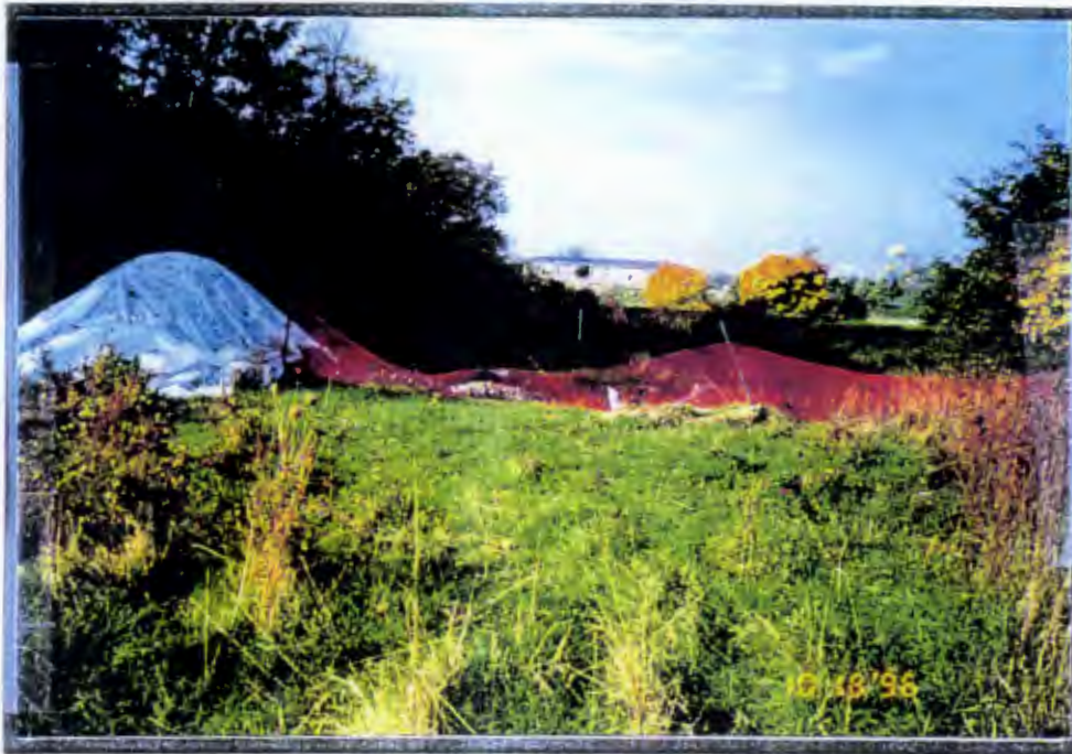
Soil excavated from drain line discharge area awaiting disposal
