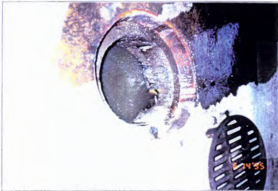
Floor drain in service bay
