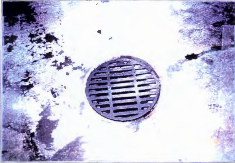
Floor drain in service bay
