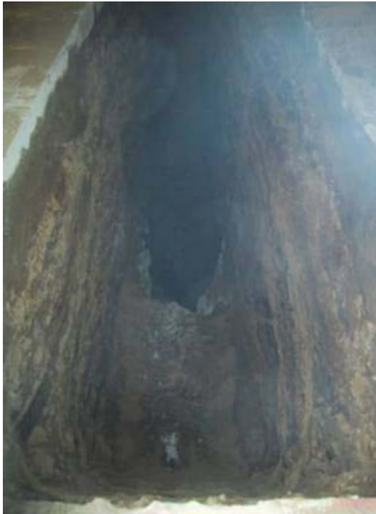
Photograph 1: Concrete slab at 7 to 7.5 feet bgs in TP-12, located at eastern edge of former 350,000 ft 3 relief holder footprint.
