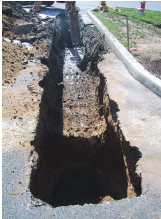
Photograph 11: Concrete pad at 5.5 to 6.5 feet bgs in TP-20, located at northern edge of former 3 million ft 3 gas holder footprint.
