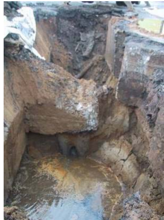
Photograph 14: Concrete and brick walls in TP-23, located within footprint of former generator house.
