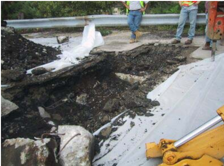
Photograph 19: Concrete partition at western end of TP-26, located within footprint of former pump house.
