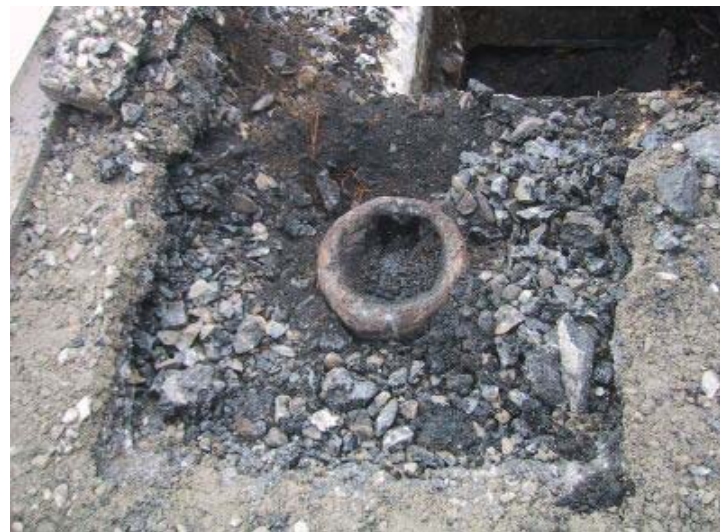
Photograph 18: Vertical pipe at approximately 0.5 feet bgs in TP-26, located within footprint of former pump house.
