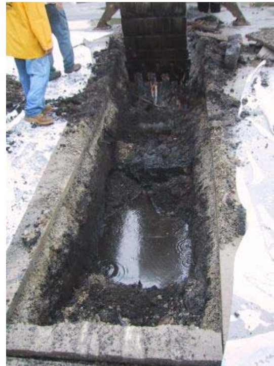
Photograph 16: Black-stained material and NAPL on groundwater at 1 to 4 feet bgs in TP-25, located within footprint of former underground brick tar tank.
