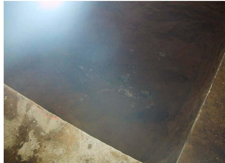
Photograph 2: Concrete slab at 7 to 8 feet bgs in TP-12B, located in center of former 350,000 ft 3 relief holder footprint.
