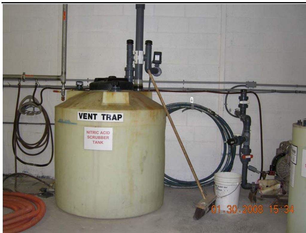
Photo 20 Nitric acid scrubber. [Scrubbers not in operation during sampling event.]
