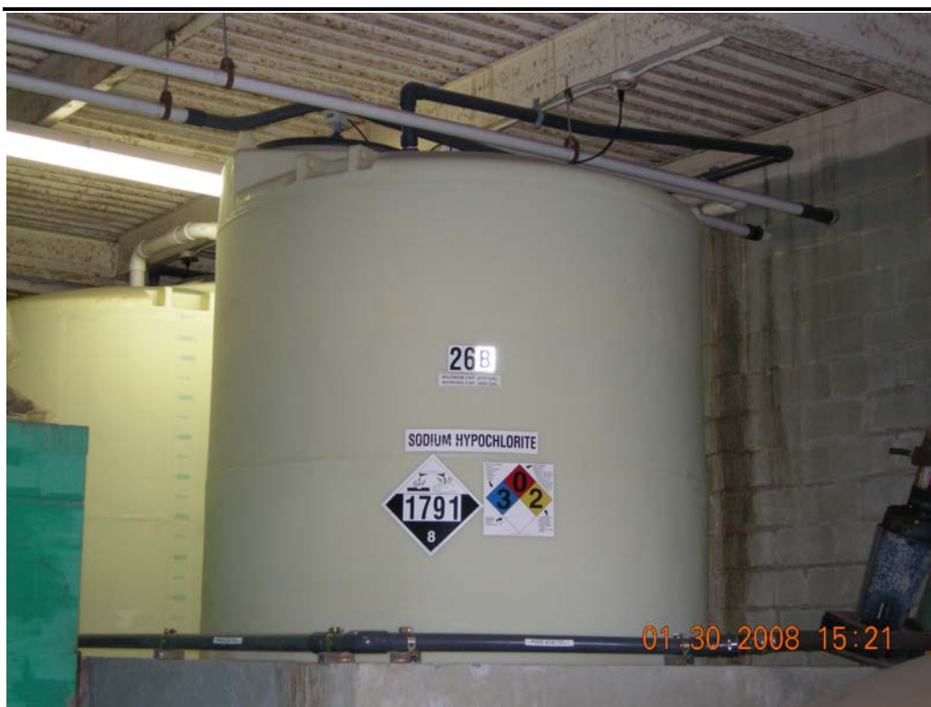
Photo 18 Bulk sodium hypochlorite tank.
