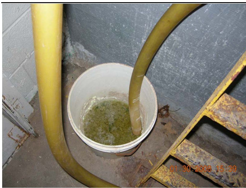
Photo 24 Bleach line capture bucket.
