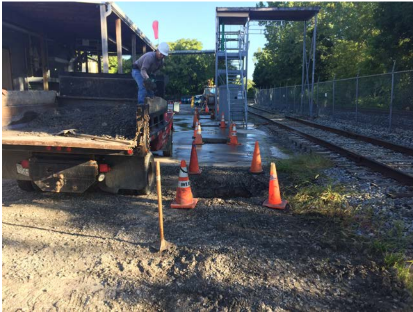
Excavations for Canopy Foundations
