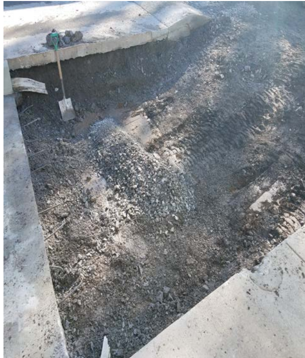
South Excavation for Truck Scale
