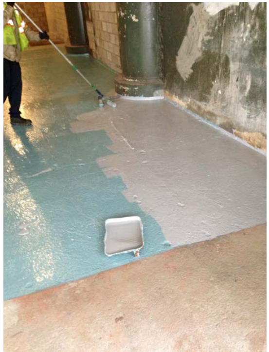
Applying second coat of epoxy
