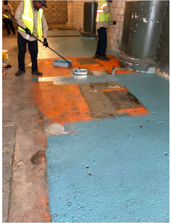
Applying first epoxy coat
