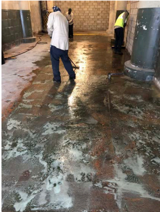
Initial concrete wash
