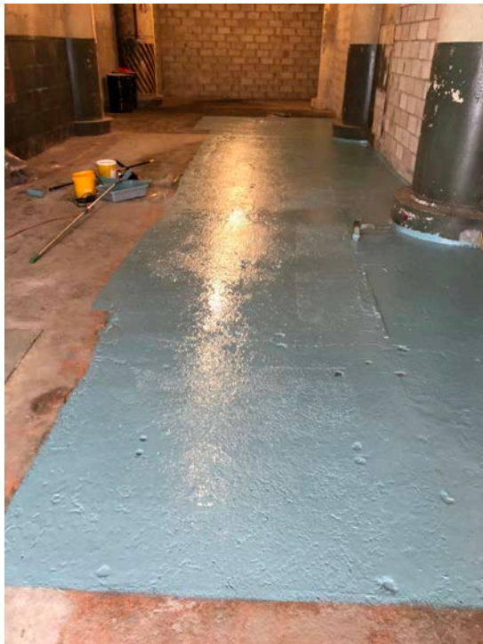
First coat of epoxy
