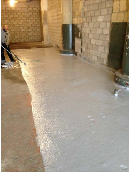
Second coat of epoxy
