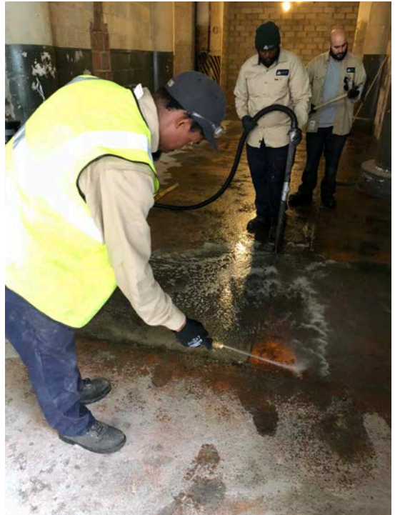
Initial concrete rinse
