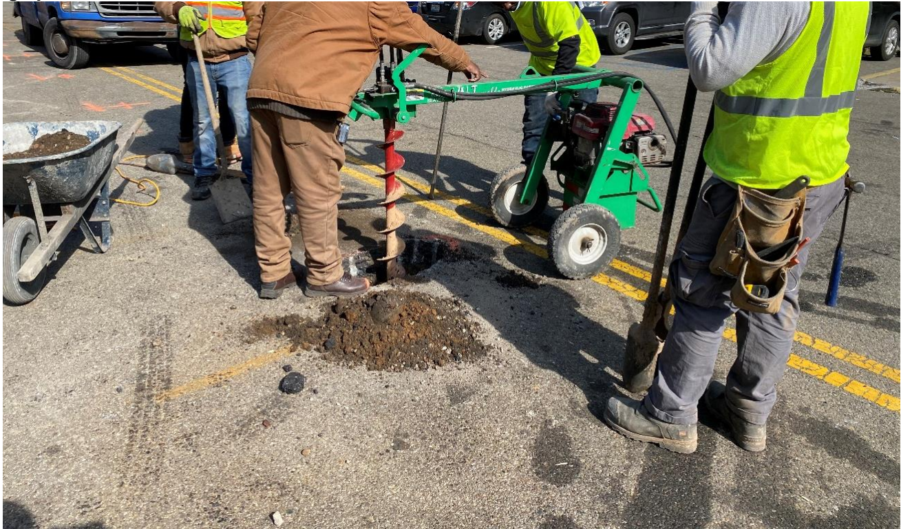
Photo 1: View of Forrester excavating holes for fence post installation (facing northwest)
