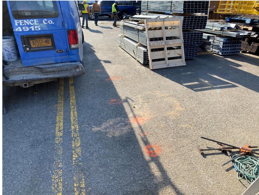
Photo 1: Markout of post-hole locations (facing northwest)– 3/10/2021
