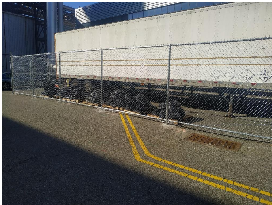
Photo 8: Installed fence with concrete filled post-holes and restored site cap (facing southwest) – 3/11/2021
