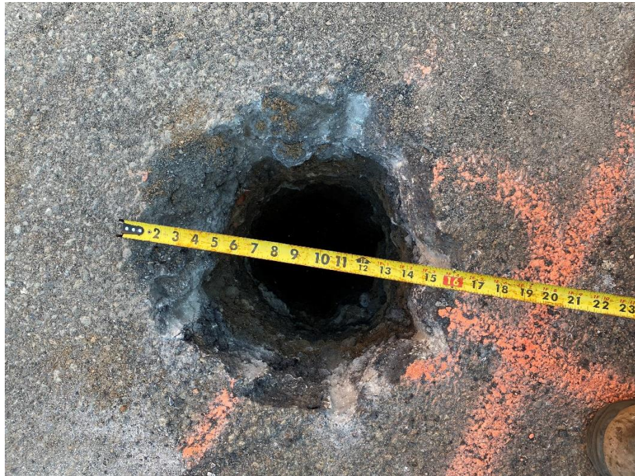
Photo 4: Typical post-hole excavation – 3/10/2021
