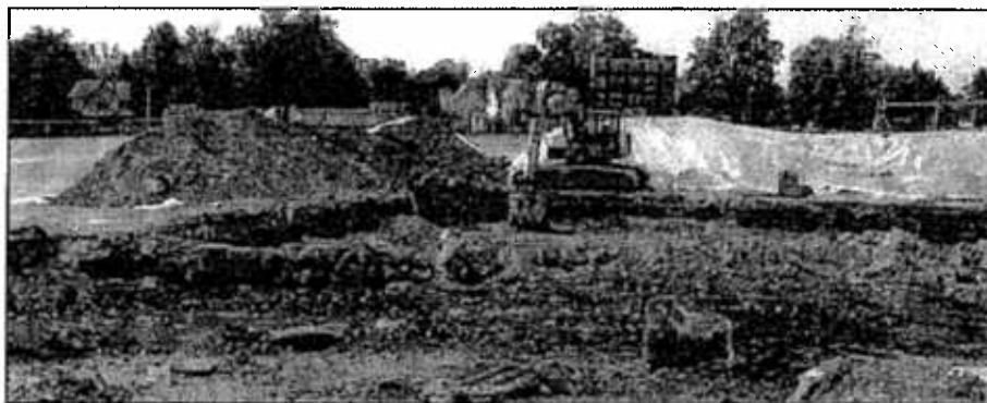
Picture 3-1 Asphalt Removal
