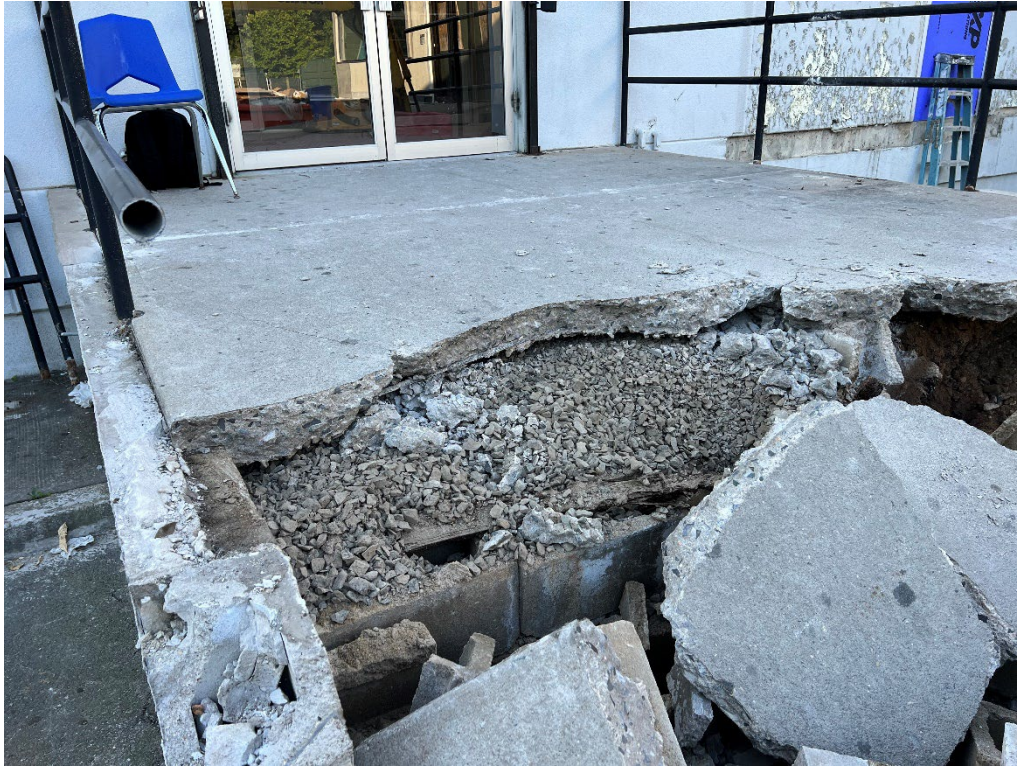
Photo 3: View of the crushed stone encountered in the void space beneath the stairs
