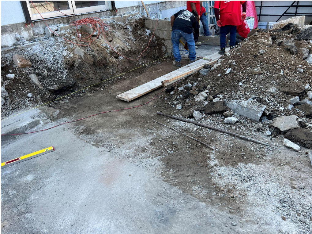
Photo 5: View of asphalt surface beneath the former stairs
