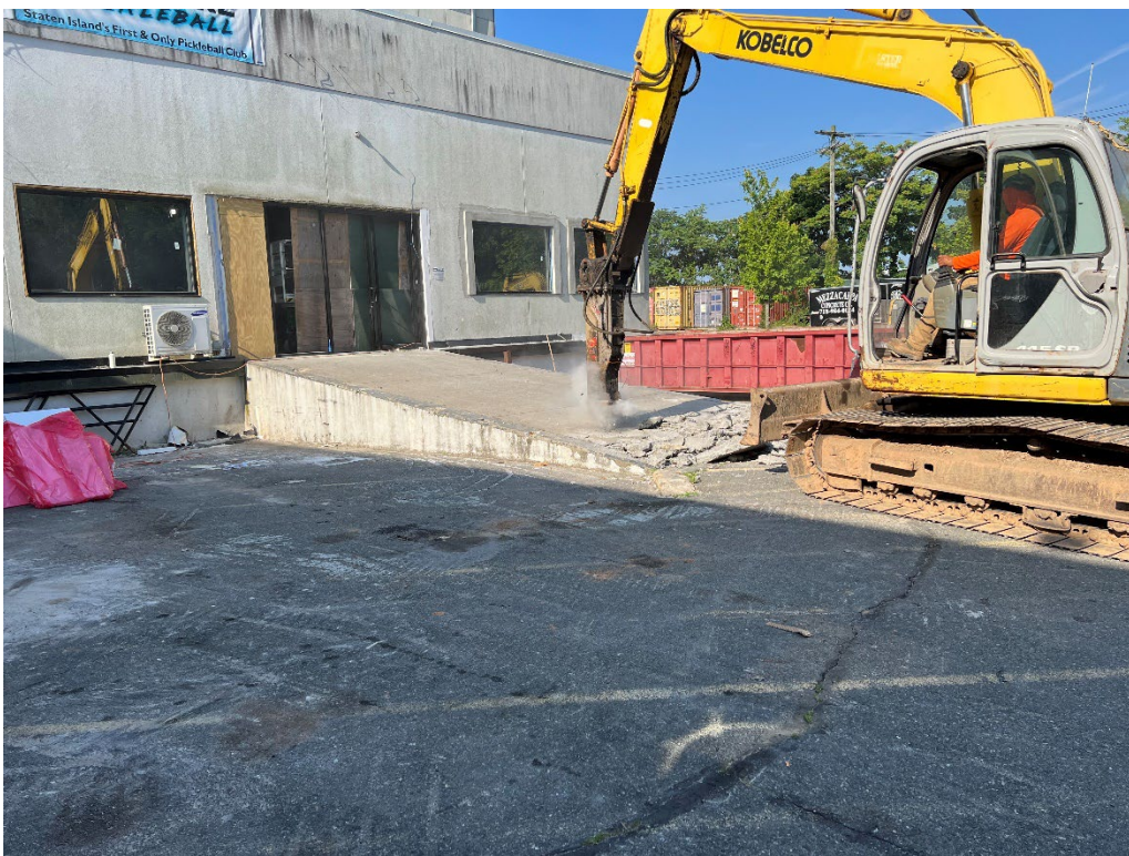
Photo 6: View of concrete ramp being demolished
