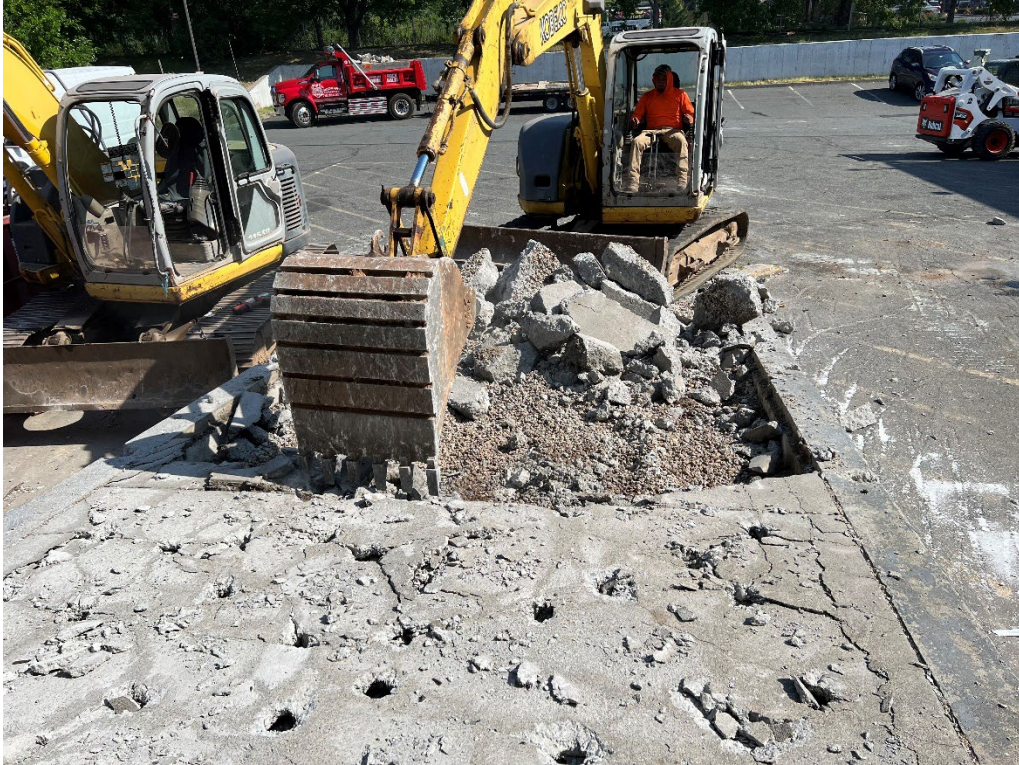
Photo 7: View of pea gravel encountered in the void space beneath the concrete ramp
