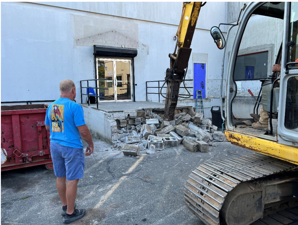
Photo 2: View of the concrete stairway being demolished
