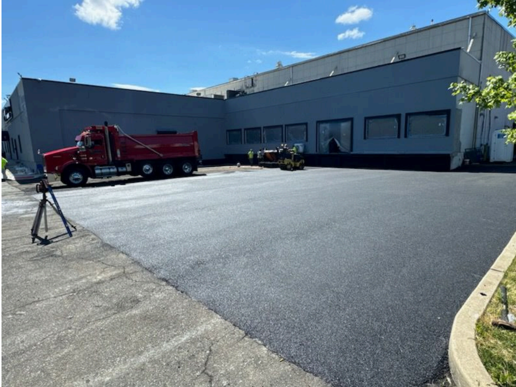
Photo 9: View of asphalt being placed on the pre-construction capping system(s)
