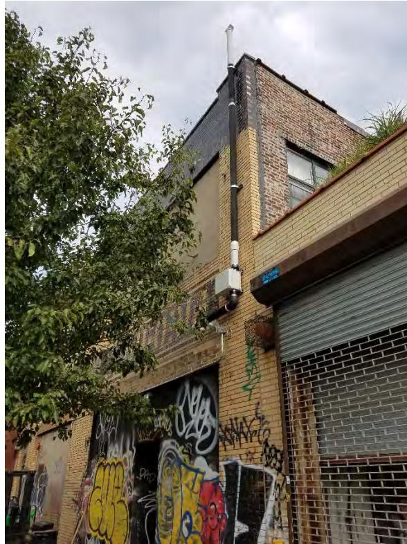
08/08/16: View of SSD System blower and discharge piping
