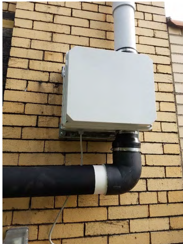
08/08/16: SSD System blower mounted to exterior building wall
