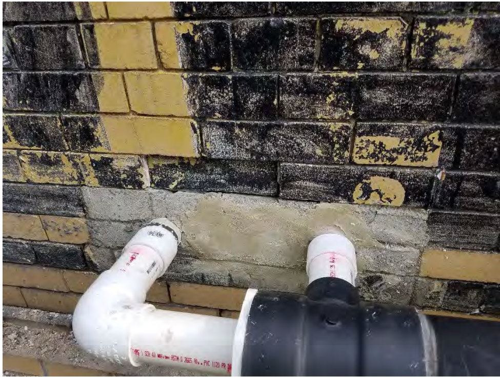
08/08/16: SSDS System piping penetration of exterior building wall
