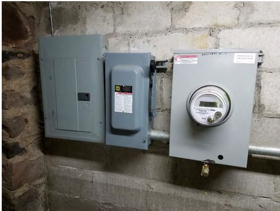
08/08/16: Installation of new disconnect switch and electrical distribution panel
