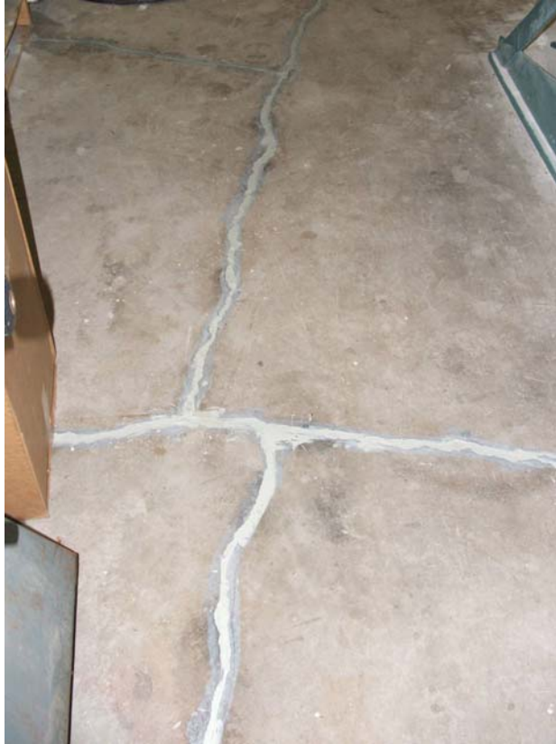
Typical Crack Sealing (using urethane caulk)
