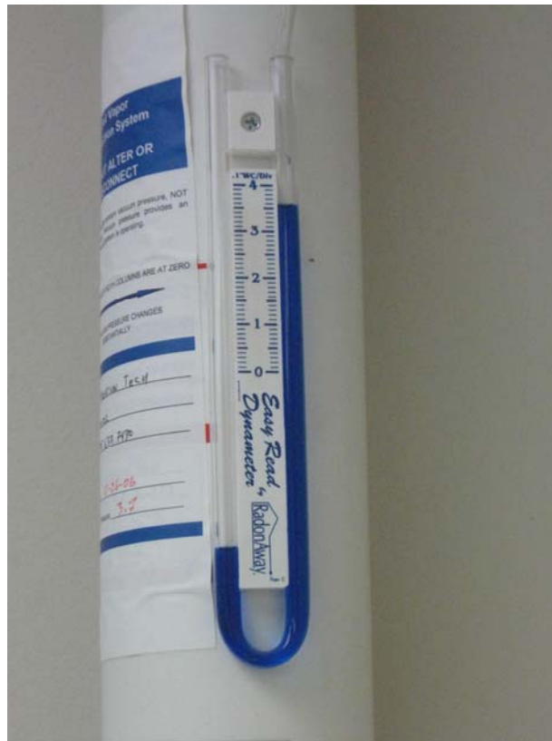
SSD – Typical Stack to Roof with Warning Device and Label
