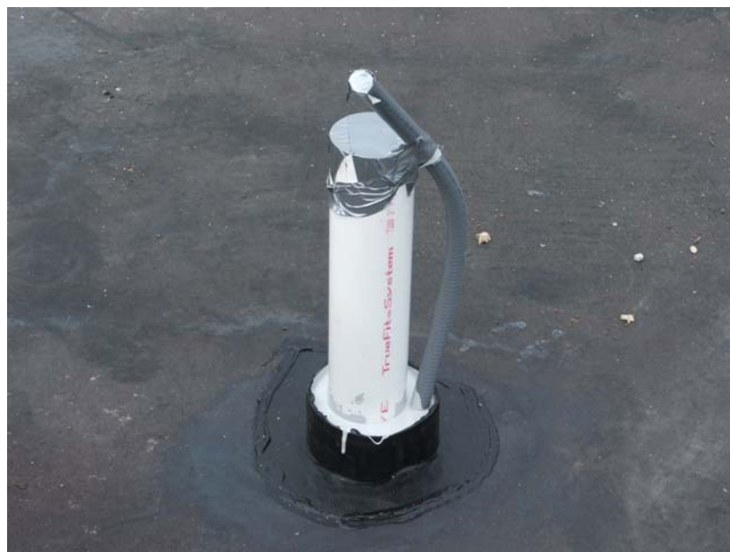
Roof – Typical Roof Penetration
