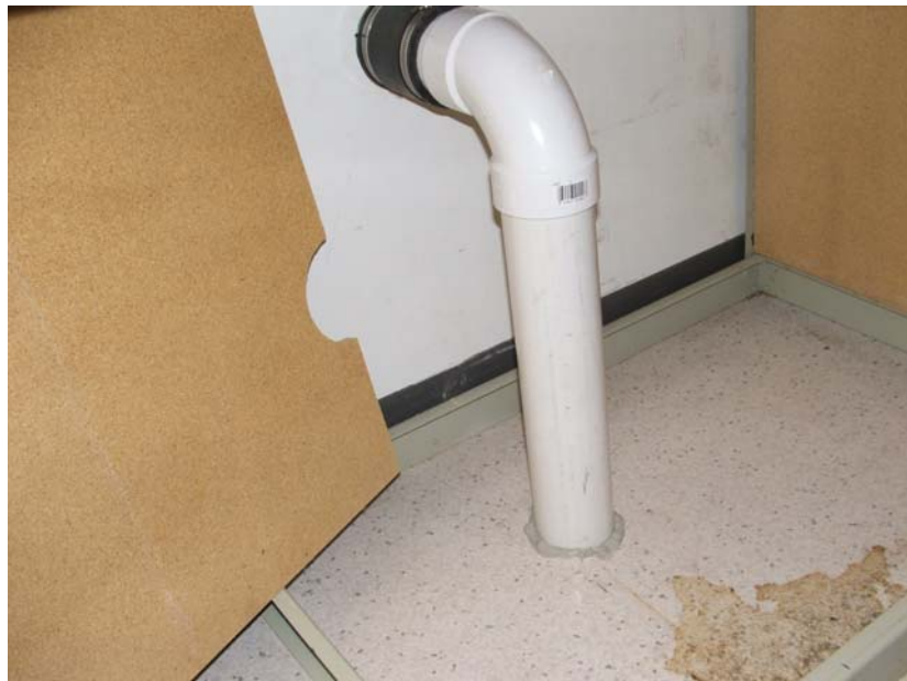
SSD – Typical Penetration (sealed with urethane caulk)
