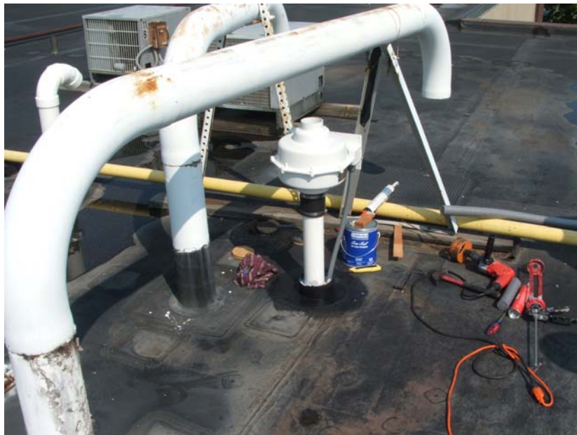
Roof – Typical SSD Exhaust
