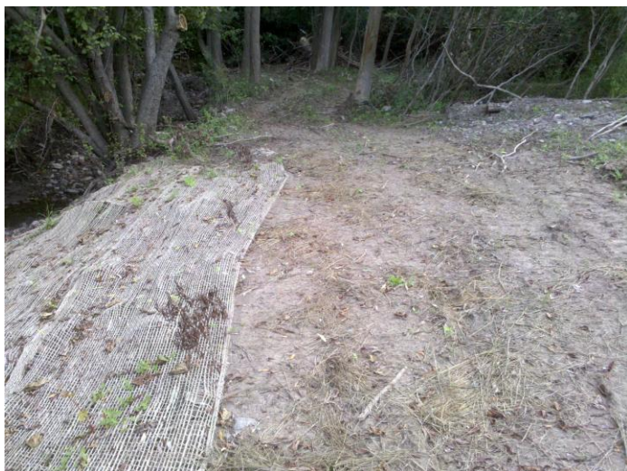
View of Outfall #2 work area and jute approximately 1 month after remedial activities.
