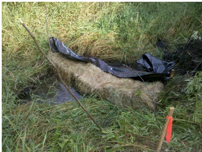
View of Outfall #1 downgradient sediment dam.
