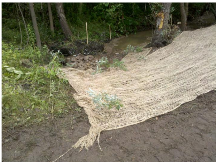
View of jute mesh on bank of Outfall #2 held in place with black locust live stakes.
