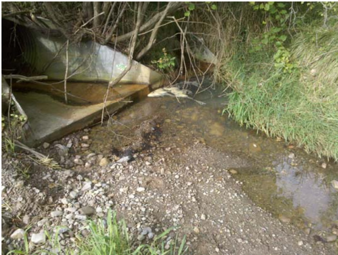
View of Outfall #2.
