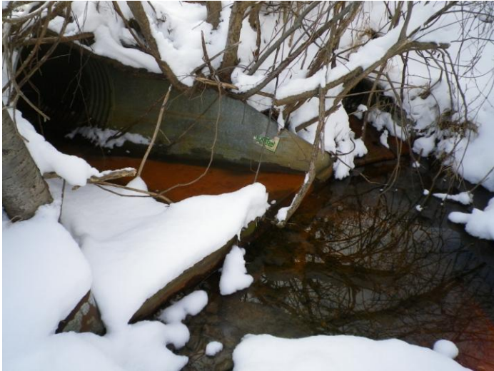
View of Outfall #1.
