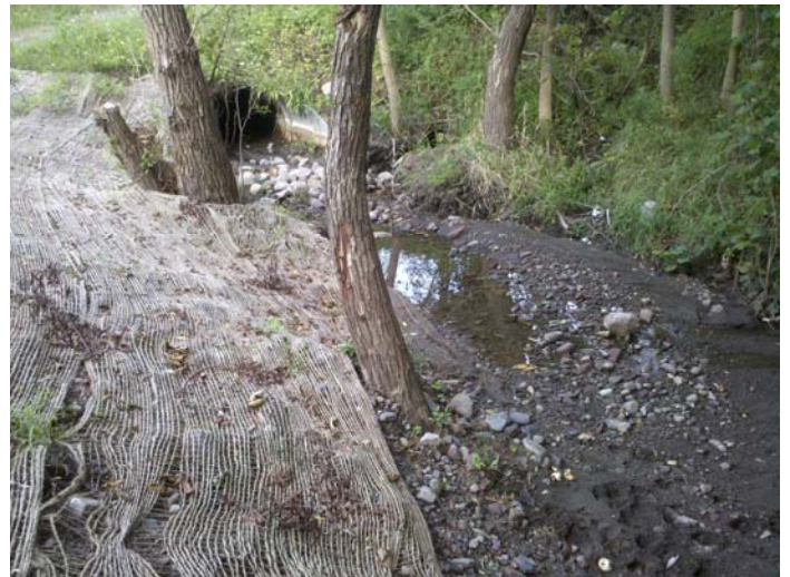
View of upper extent of Outfall #2.
