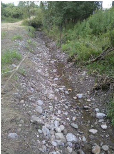
View upgradient of Outfall #2.
