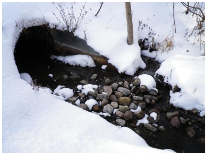
View of Outfall #2.
