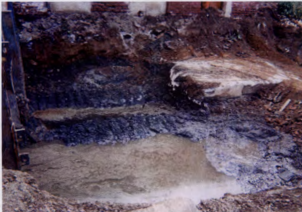
Figure 2 – Soil excavated to bedrock in western portion of the excavation. A concrete encased 550 gallon tank was encountered.
