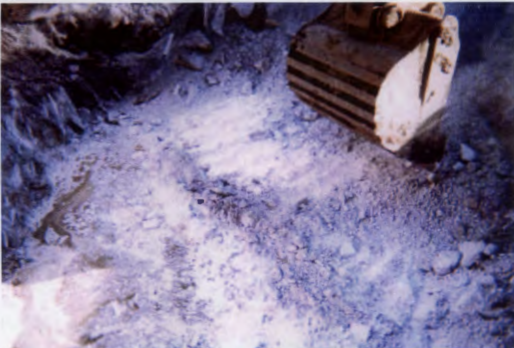
Figure 10 – ORC application within the excavation.
