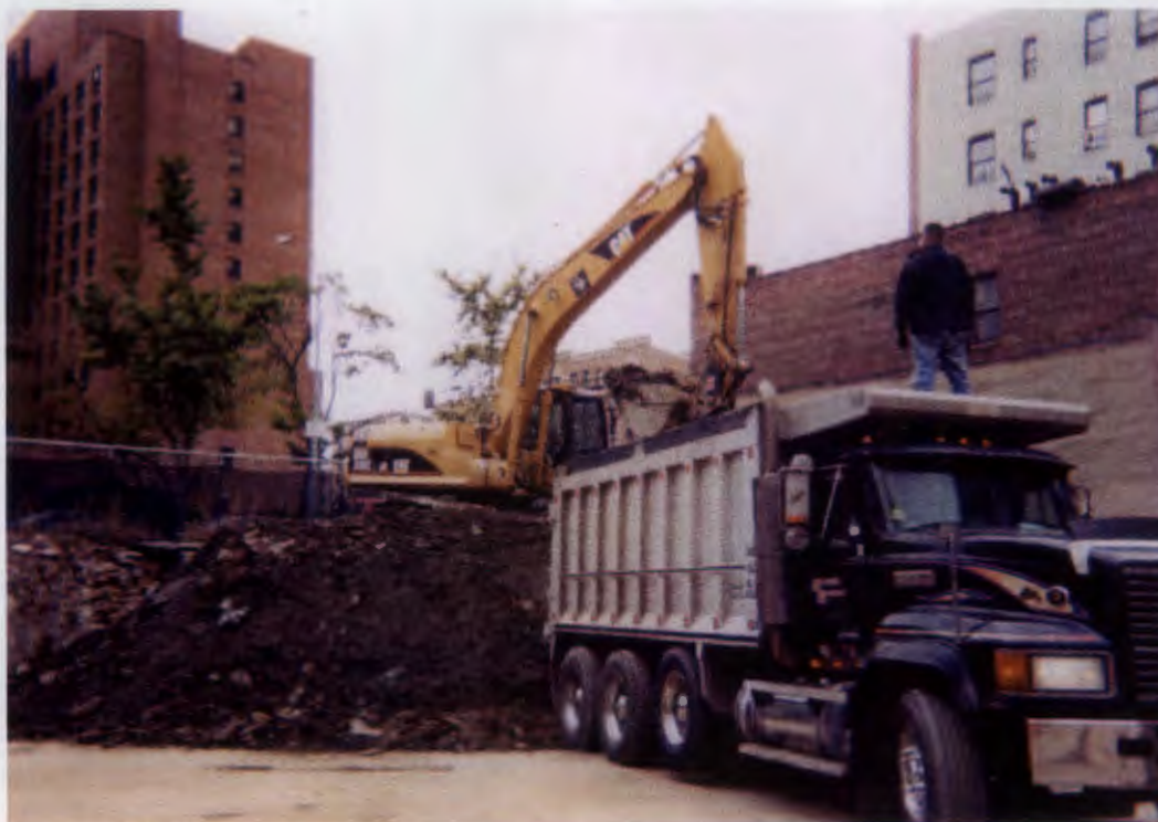
Figure 18 – Soil was loaded out by dump truck for disposal.
