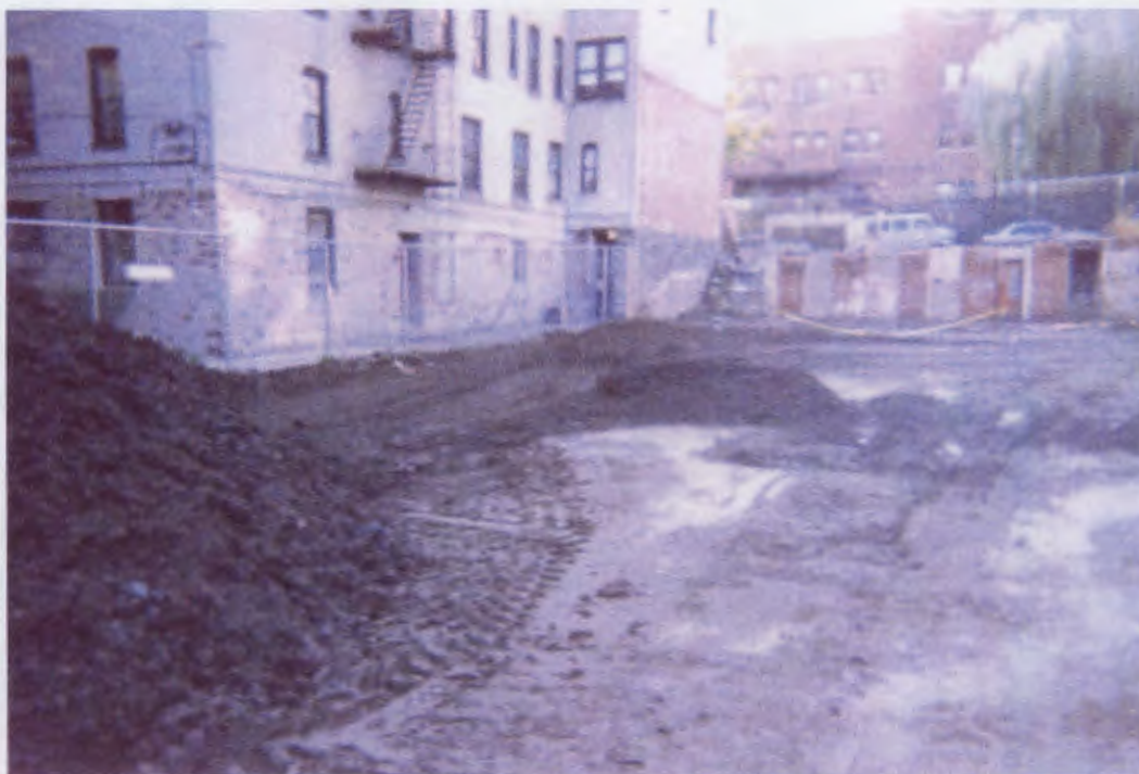
Figure 14 – Central portion of the site backfilled.
