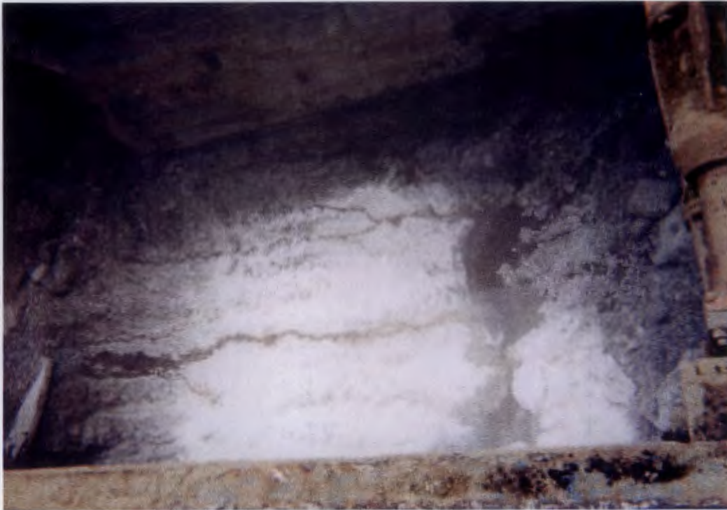
Figure 5 – ORC application within the excavation shown on Figure 3.
