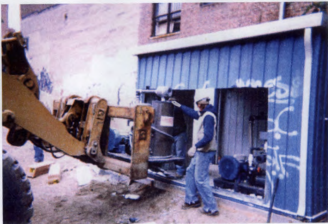
Figure 19 – The SVE system was dismantled and removed from the site.
