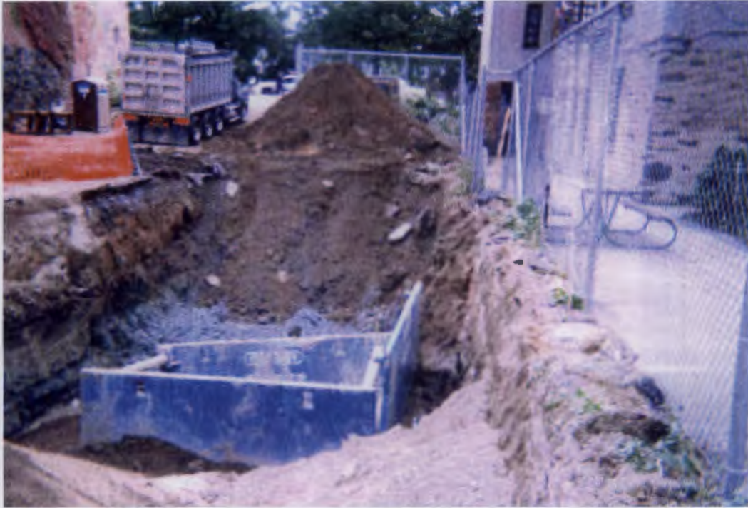
Figure 7 – Excavation along the south property line. Impacted soil was noted at approximately eight feet below grade.
