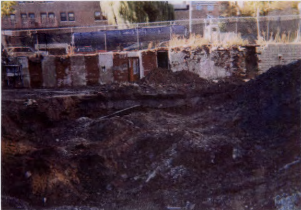
Figure 15 – Excavation was extended to the north to remove impacted soils.
