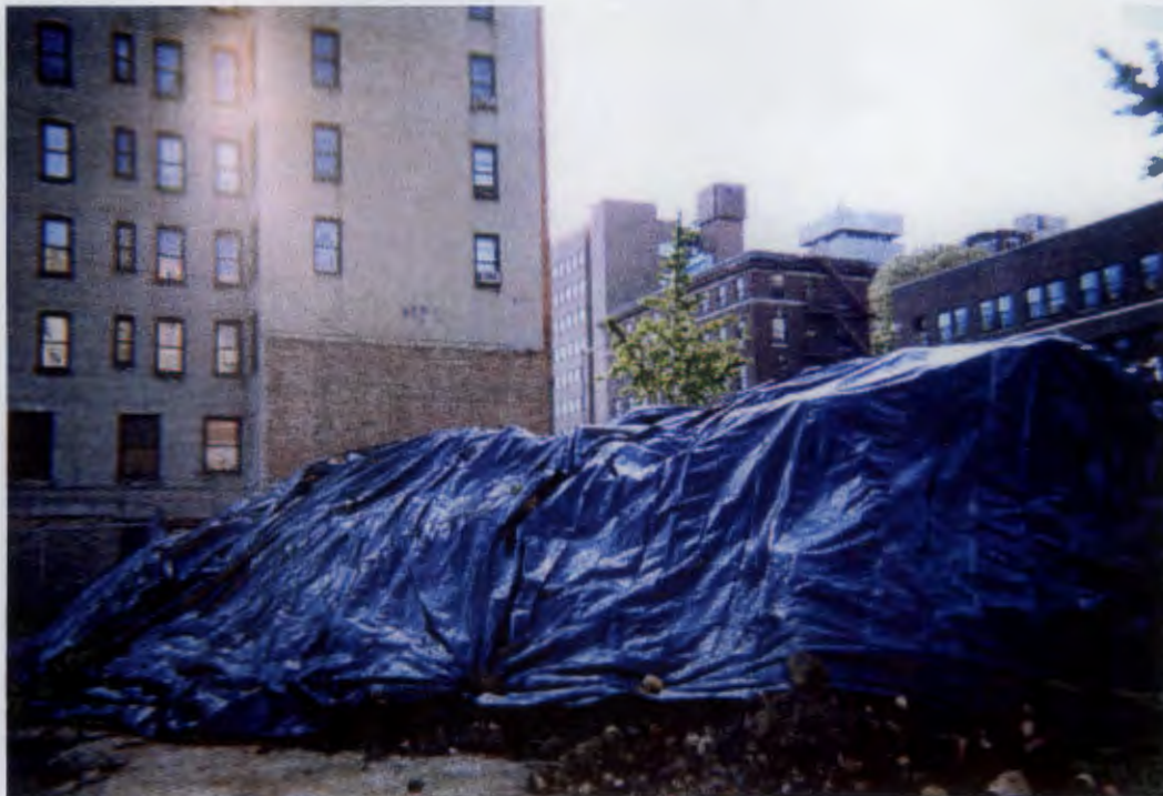
Figure 17 – During the excavation phase, the stockpile was covered each night.
