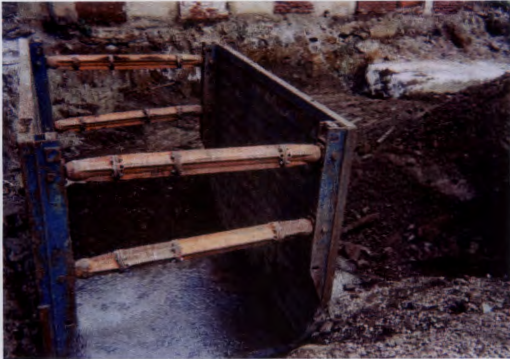
Figure 9 – Overnight groundwater would seep into the open excavation.
