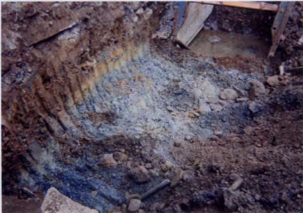
Figure 8 – Impacted soils encountered in the central portion of the excavation.
