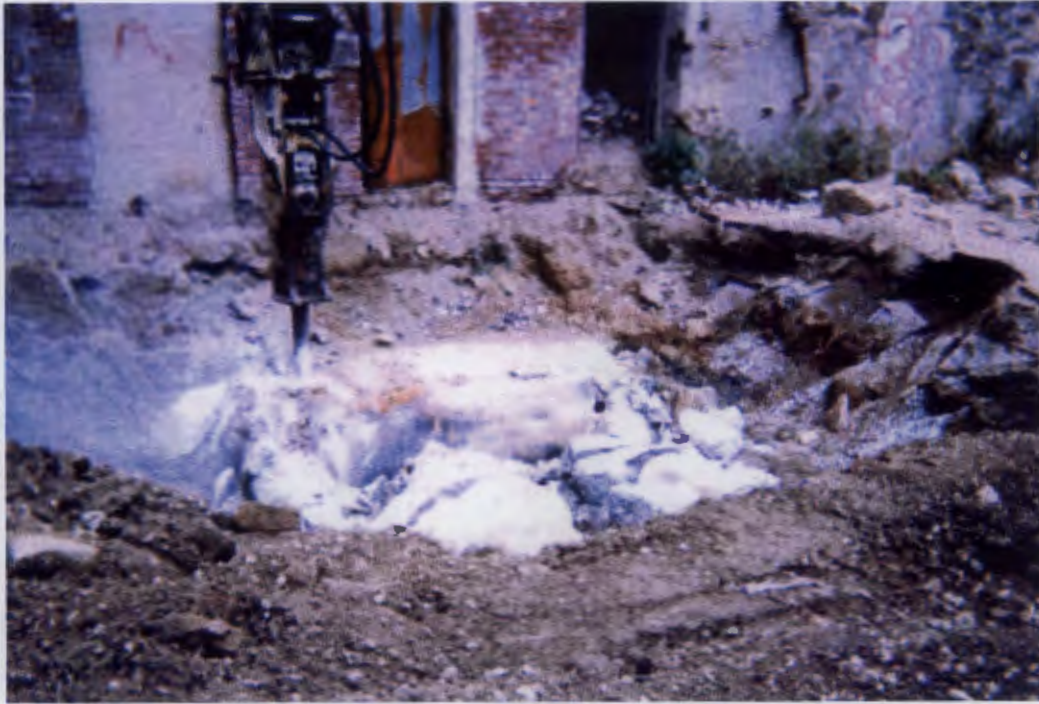
Figure 3 – Concrete vault around the tank was removed to access the tank.
