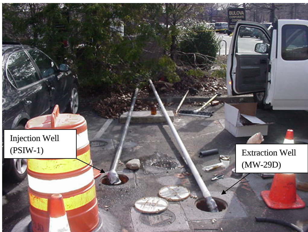
Photo 2: Extraction and Injection points (Phase 2, extraction from MW-29D, Injection into PSIW-1.
