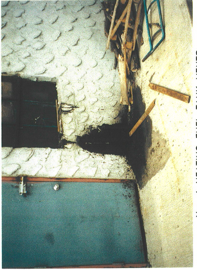
No. 4 HEATING FUEL TANK VENTS, EVIDENCE OF OVERFILLING
