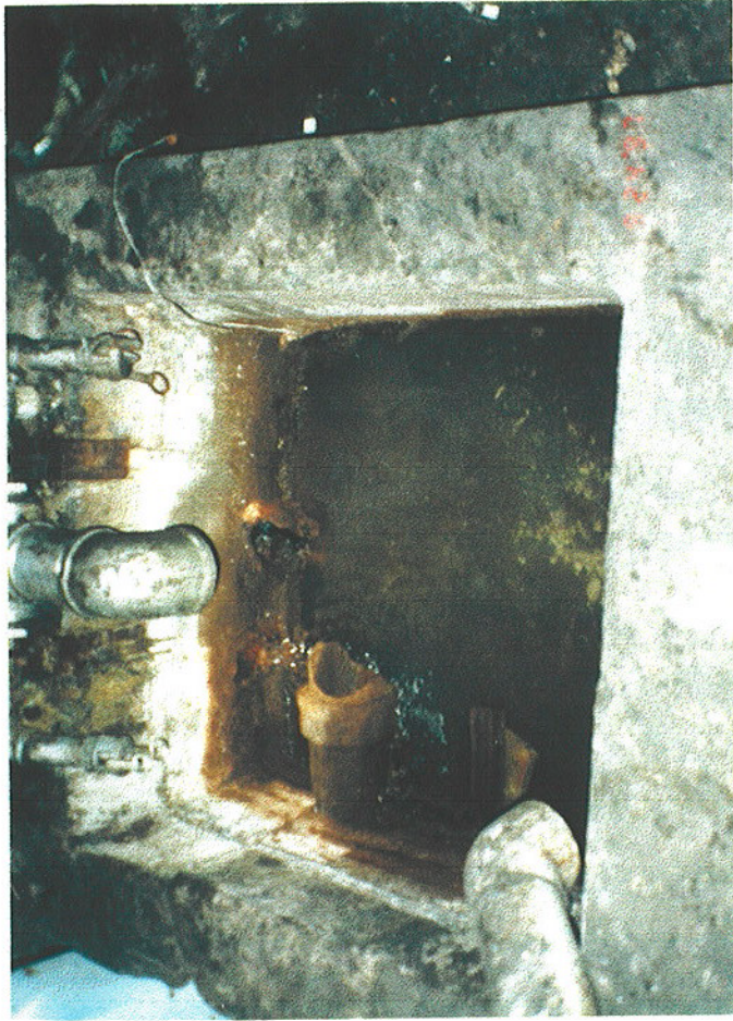
COLLECTION PIT FOR COOLING WATER, BUILDING A (SULFATIONS)
