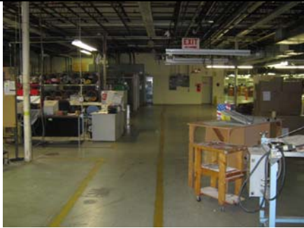
Photo 1 is a typical view of the interior production area of the Champion Products Facility.
