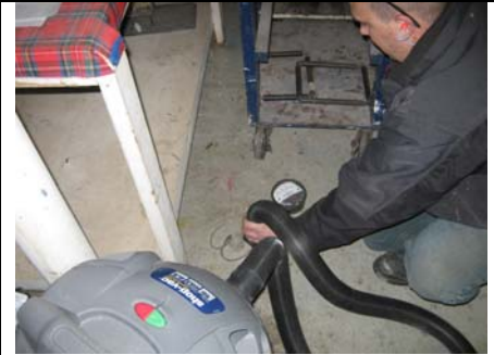
Photo 3 is a typical view of vacuum testing with a shop vac and magnahelic pressure gauge.
