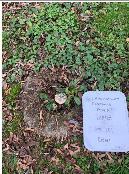
Photo 6: MW-201 before decommissioning – 11/28/22
