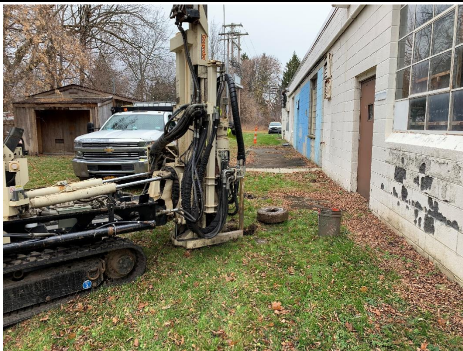
Photo 8: View of monitoring well decommissioning activities
