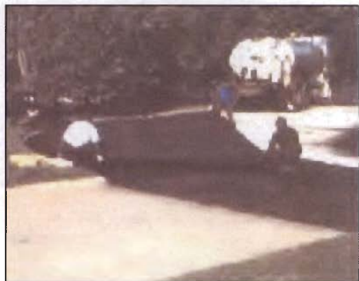
Figure 8 PETROMAT PLACEMENT AROUND CURVES
