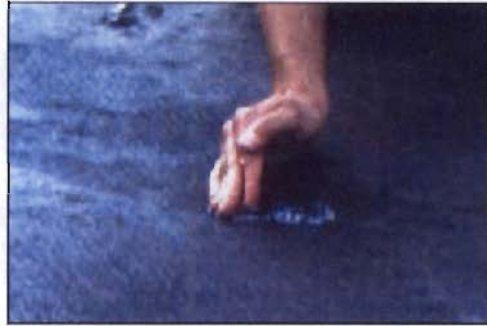
Photograph of a site that is too wet for overlay placement.
