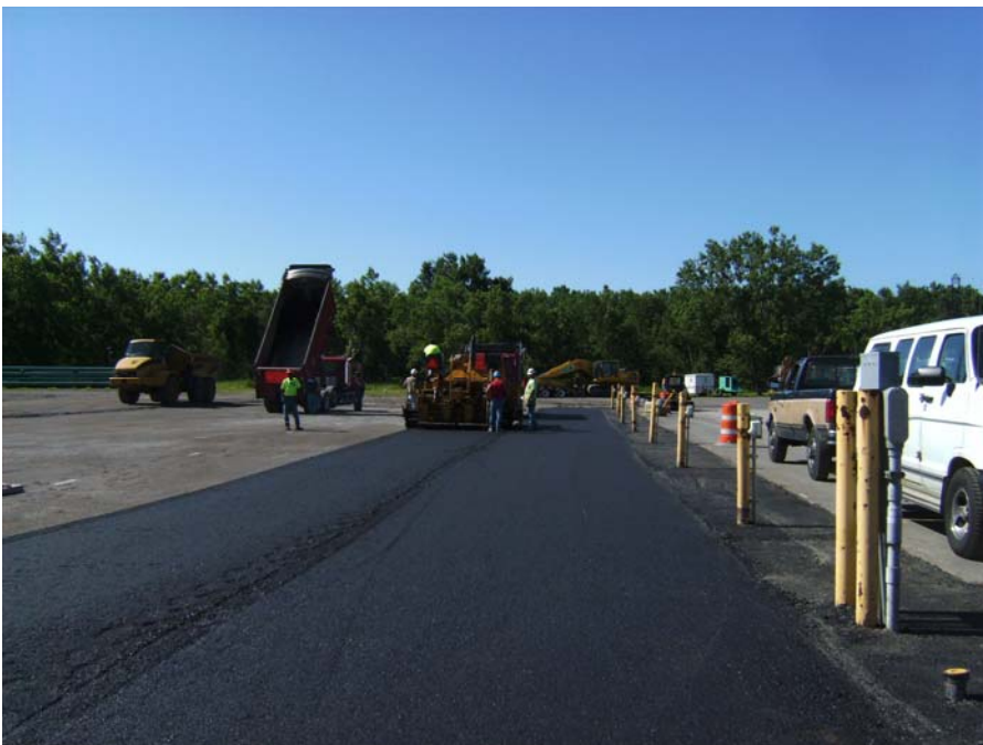
July 10, 2008 Installation of asphalt binder material.
