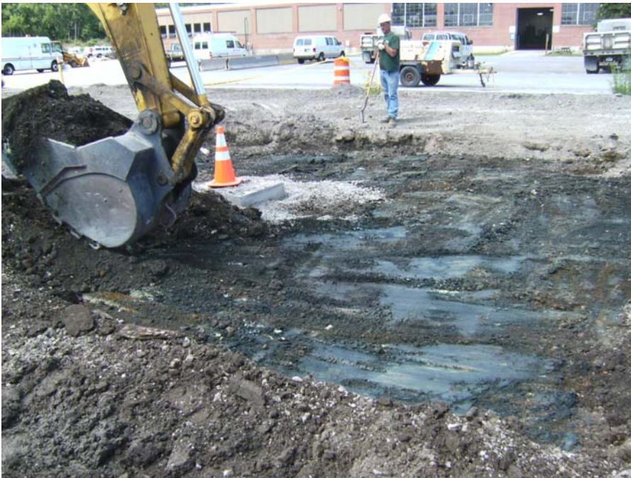
Removal of impacted soils in footprint of Building 8 Asphalt Cap.
