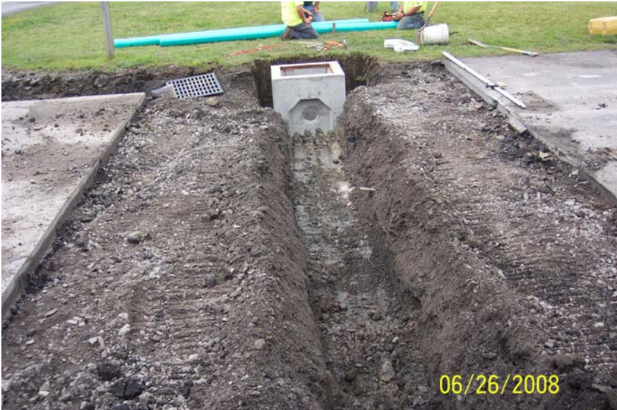
June 26, 2008 Installation of catch basin north of installed Building 8 Asphalt Cap.
