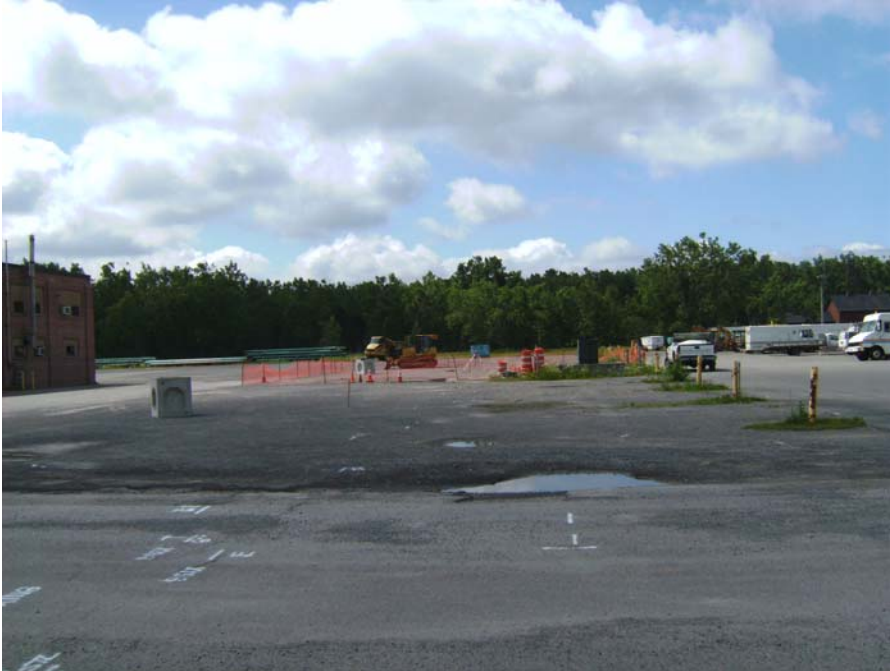
June 24, 2008 Building 8 area prior to construction activities.
