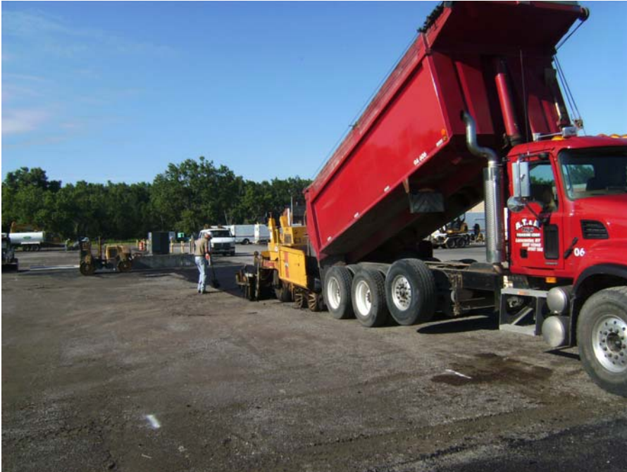
July 10, 2008 Installation of asphalt binder material.
