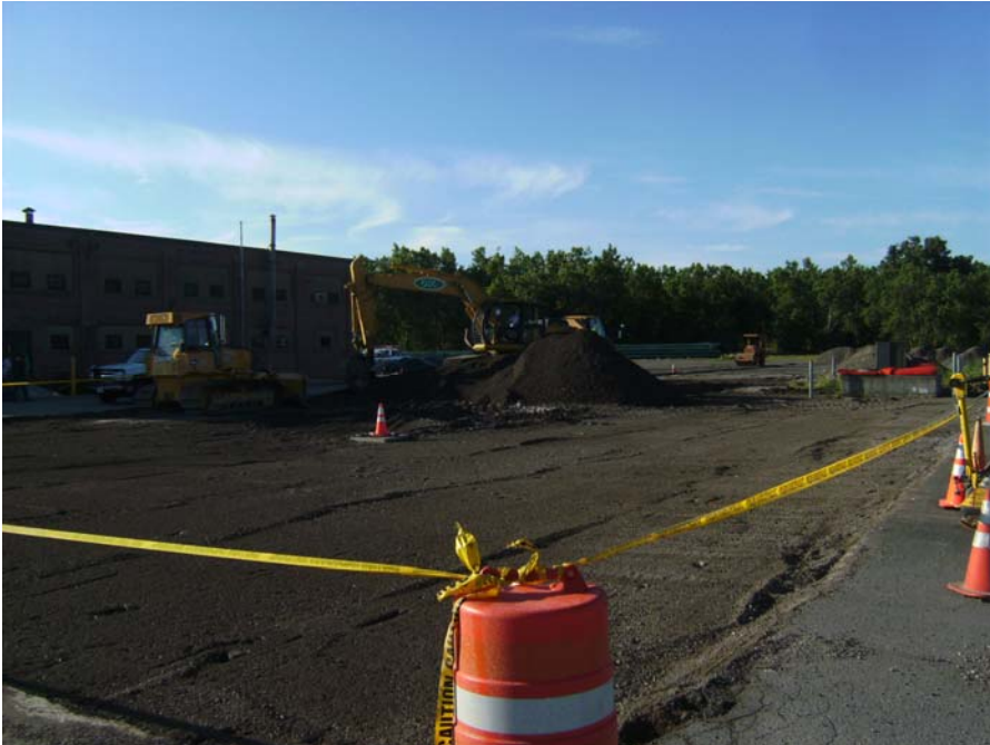
July 2, 2008 Grading and reallocation of subsurface material.
