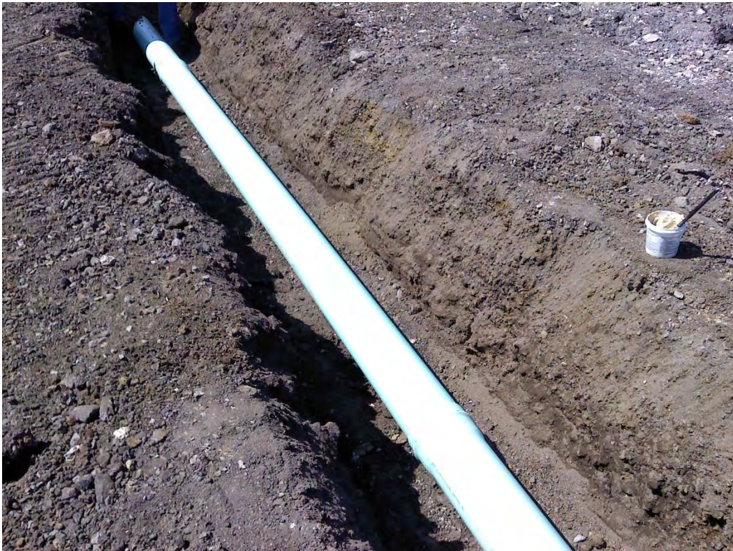
Drain pipe installed in trench.
