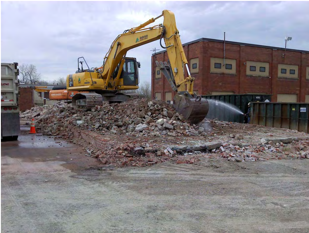
Water spray was used for dust control during building demolition.
