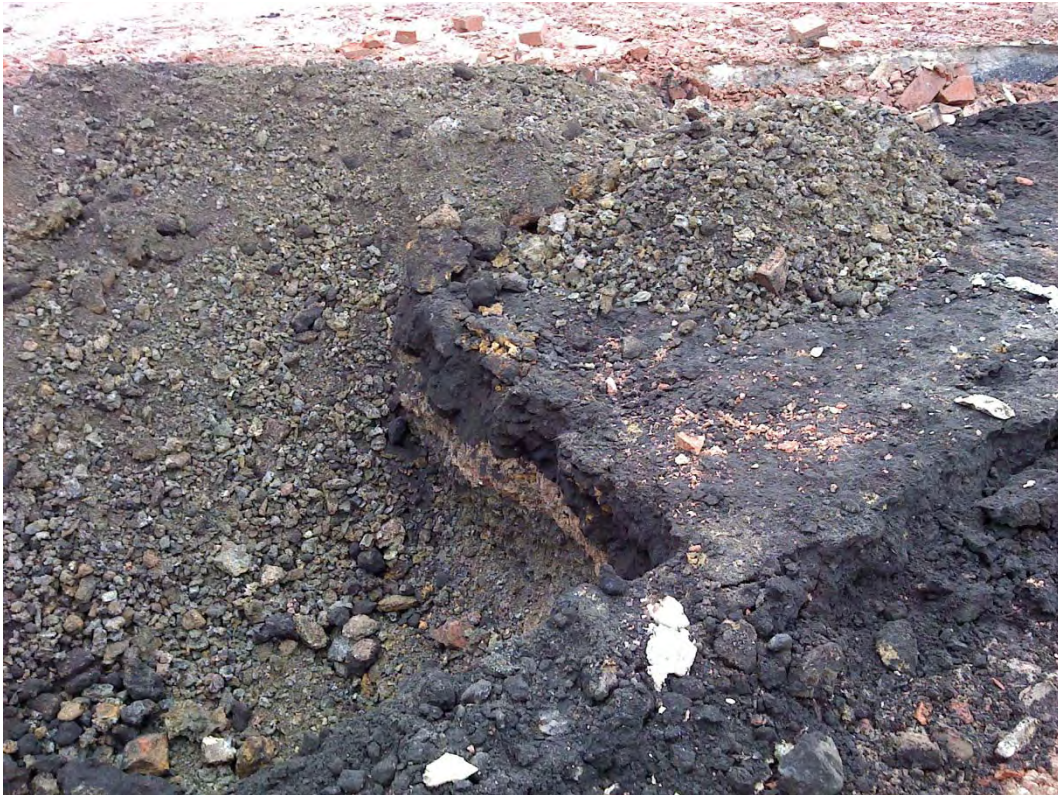
Coal slag bedding was about 6" to 8" thick.
