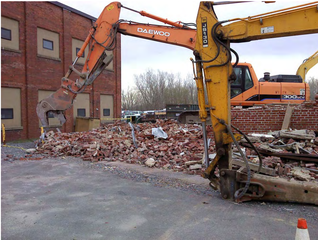
Demolition of Mineral Springs Building #8.
