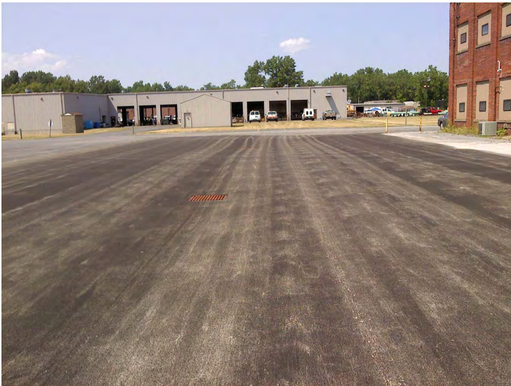
Looking north at new asphalt pavement.
