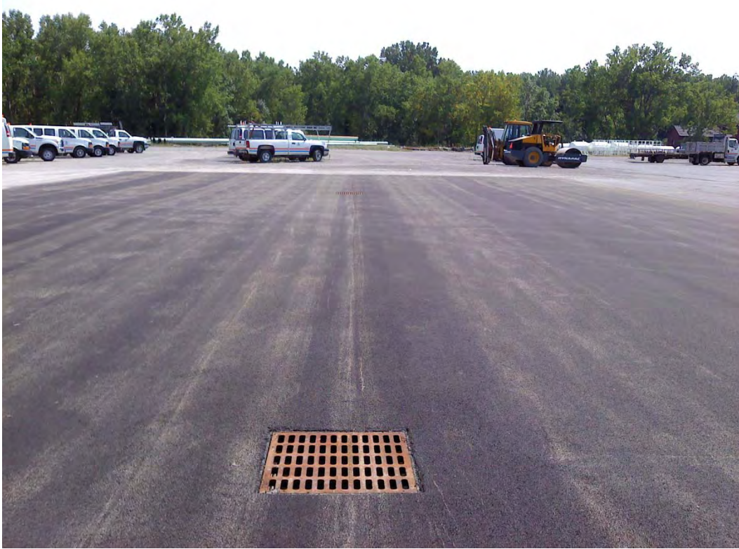
Looking south at new asphalt pavement.
