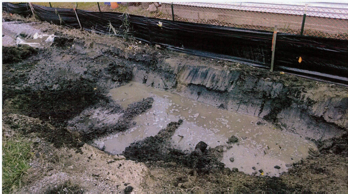
Photo 2: November 6, 2013. Facing West. Visual impact excavation along western property boundary.
