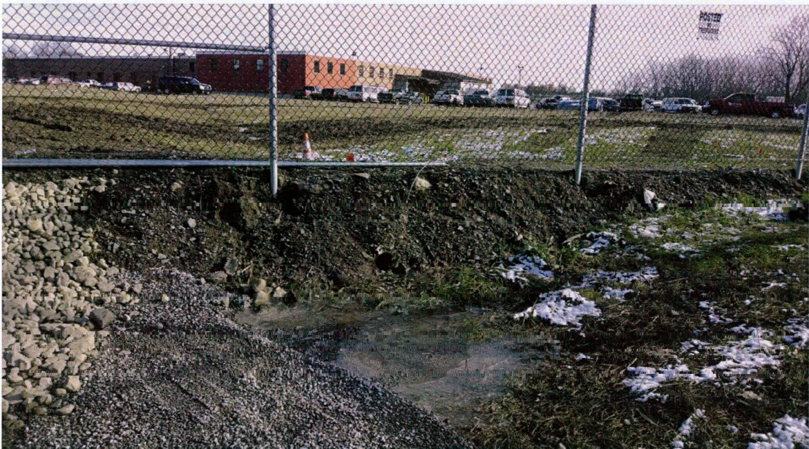
Photo 16: November 13, 2013. Facing Northeast. Known impacts area as identified in historic figure. Located north of transmission tower excavation. Note fill material used to grade fence sufficiently covers a portion of the area.
