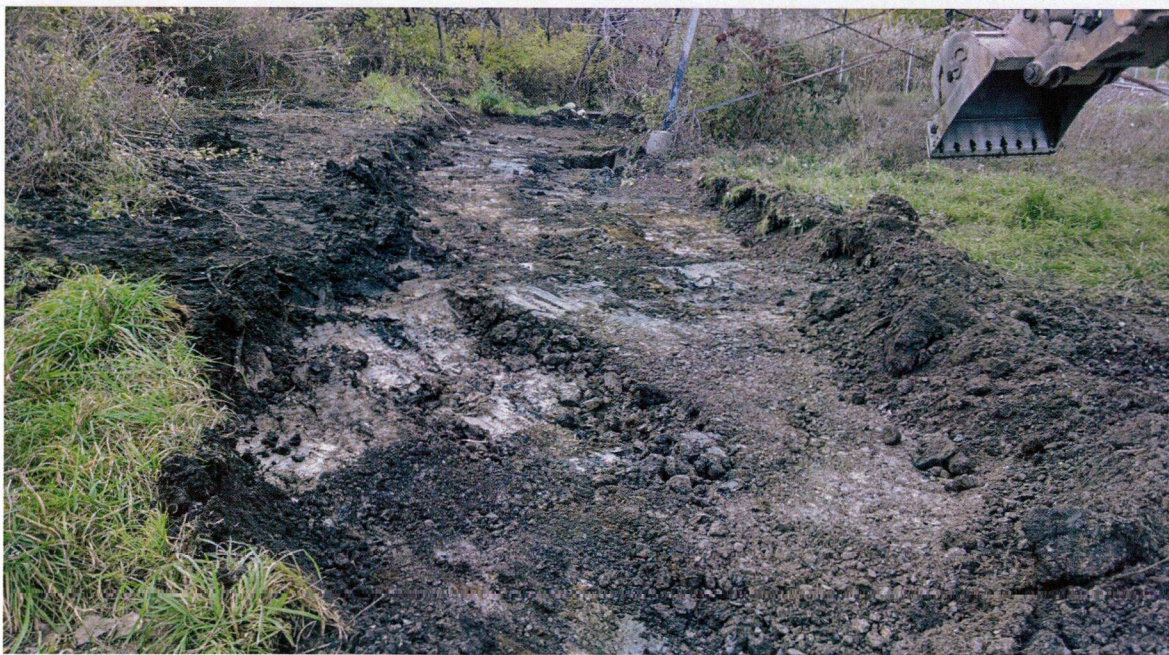
Photo 12: November 6, 2013. Facing west. Transmission tower excavation bottom.
