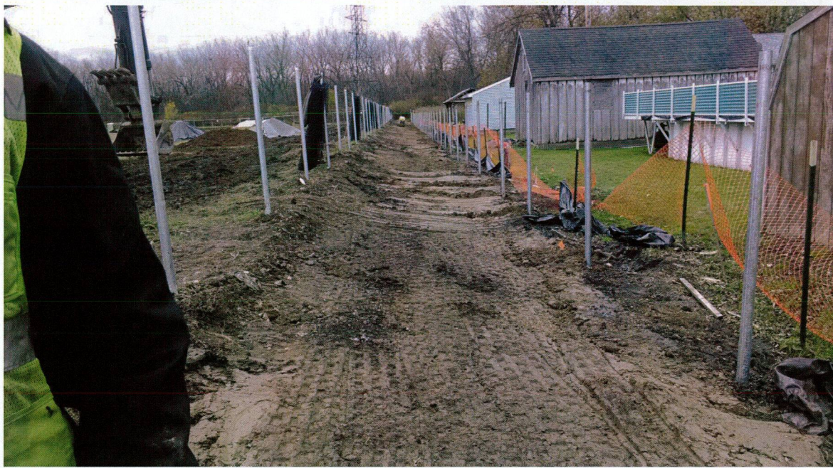
Photo 7: November 8, 2013. Facing South. Drainage ditch filled with clay and compacted with padfoot roller.
