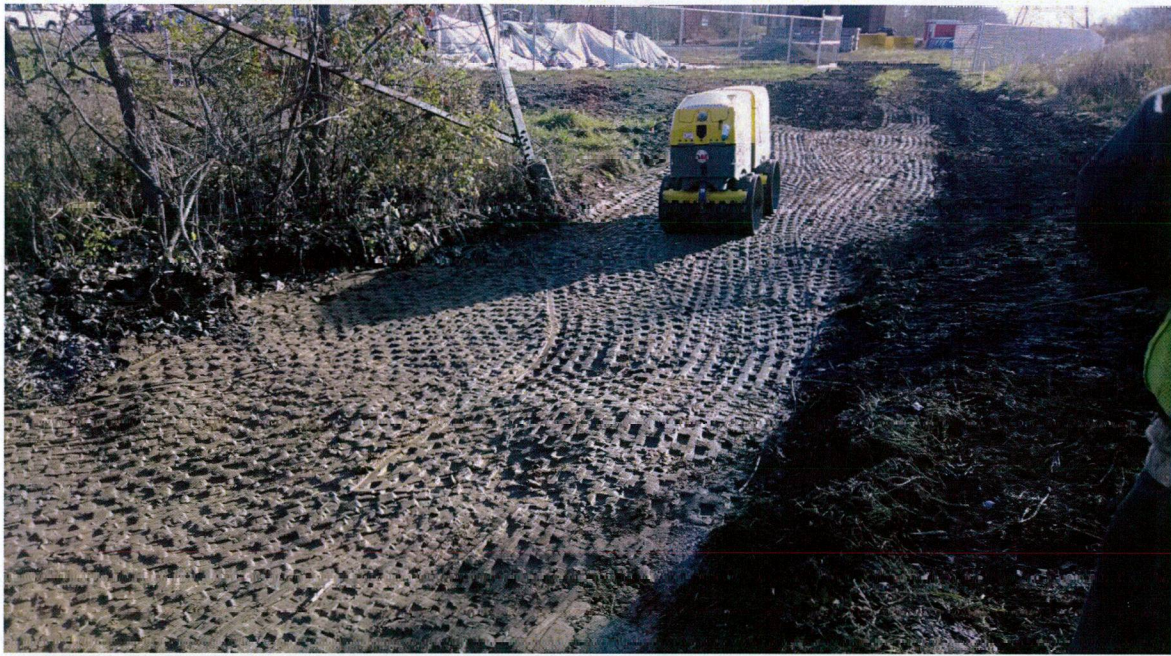
Photo 15: November 8, 2013. Facing East. Transmission tower excavation backfilled with clay and compacted with padfoot roller.
