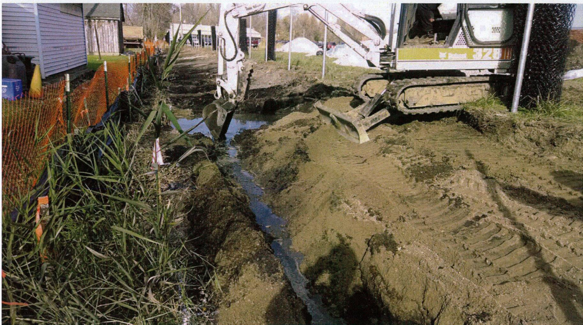
Photo 4: November 5, 2013. Facing North. Drainage ditch excavation. Note water level in excavation from Photo 4.
