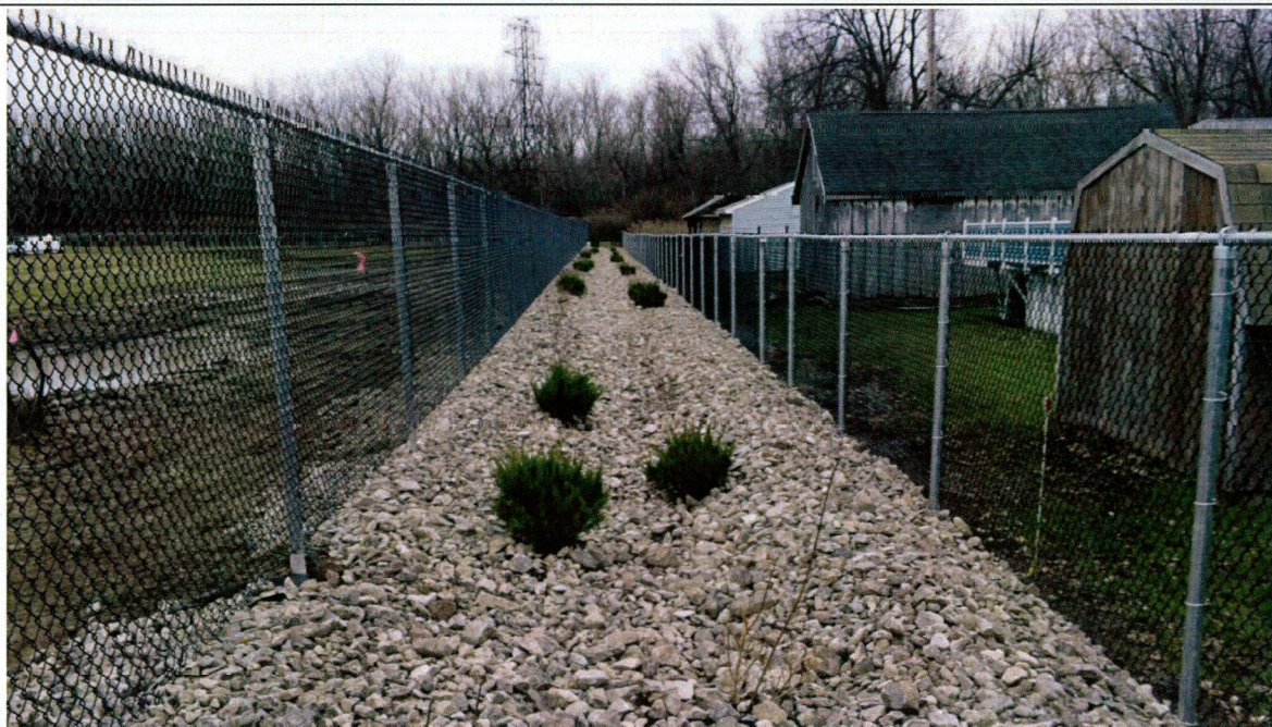
Photo 10: November 19, 2013. Facing South. Completed berm area with both fences installed.
