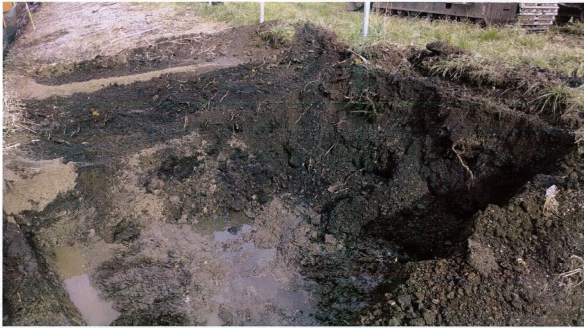
Photo 3: November 4, 2013. Facing Northeast. Visual impact excavation, along western property boundary, starting to fill with water. Water eventually filled excavation to ground surface (see Photo 5).
