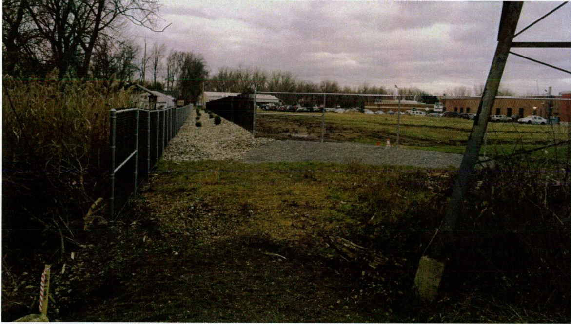
Photo 11: November 19, 2013. Facing North. Completed berm area with both fences installed.
