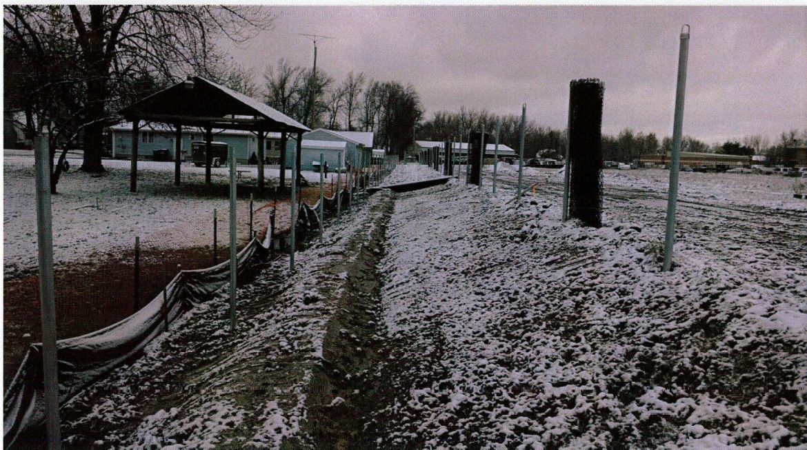
Photo 8: November 12, 2013. Facing north. Berm constructed with clay. Geotextile (Mirafi® 600X woven polypropylene) and gravel are spread on northern end of berm. Note roll of geotextile fabric placed on berm.
