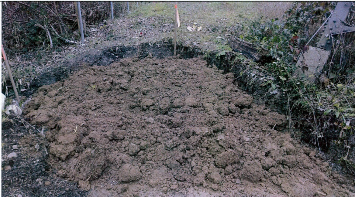
Photo 14: November 7, 2013. Facing North. Clay material backfilled into excavation west of tower. Note photo taken before clay was compacted.
