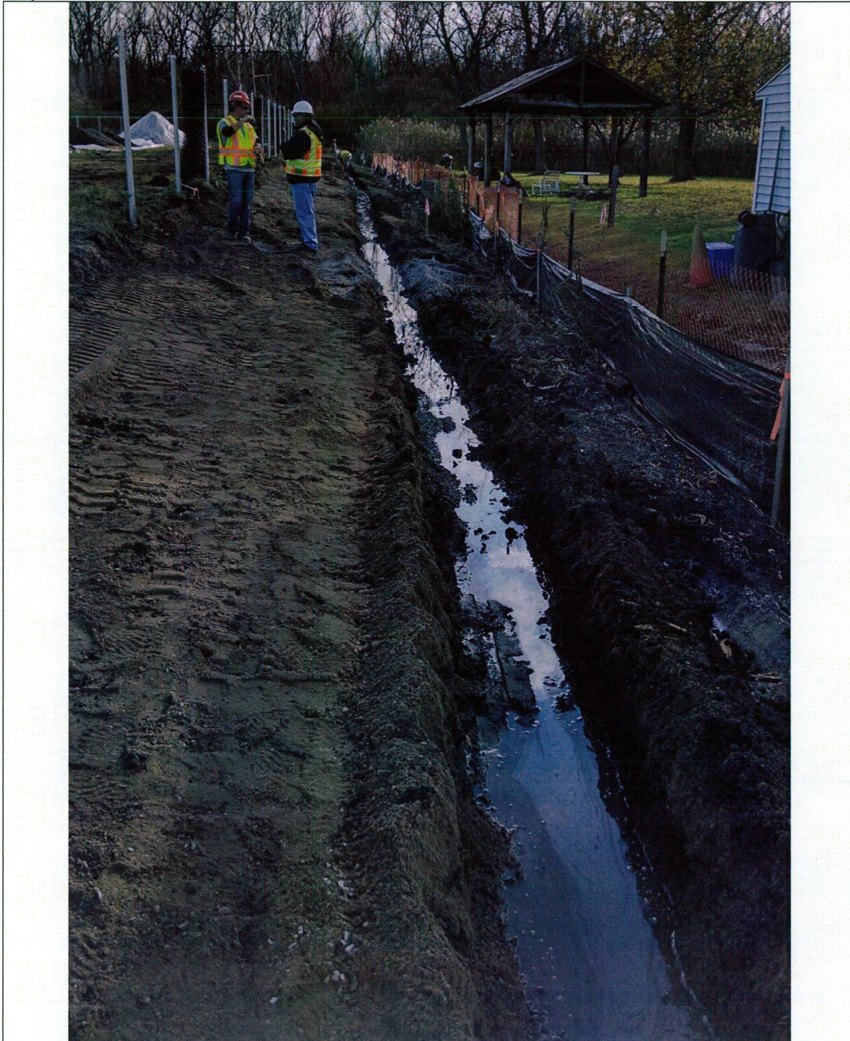
Photo 6: November 5, 2013. Facing South. Excavated drainage ditch. Water infiltrated into ditch.
