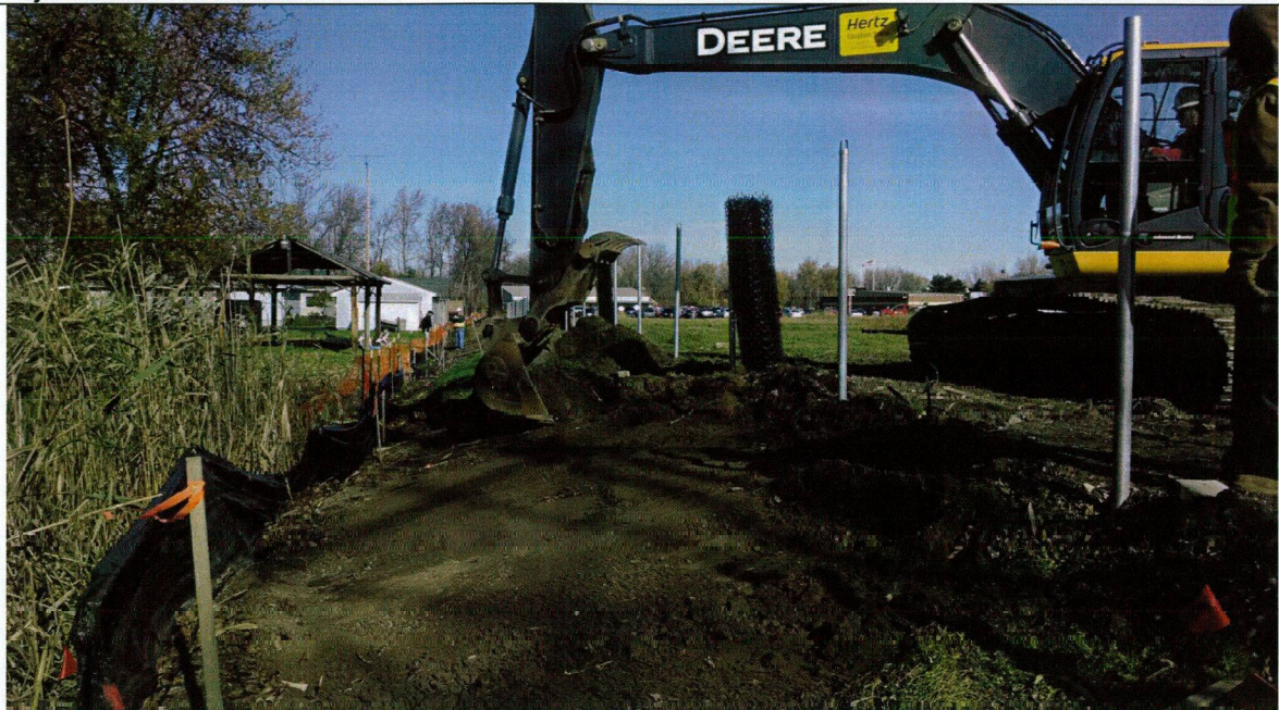
Photo 1: November 4, 2013. Facing North. Clearing western property boundary. Note black silt fence in place along downslope area. Silt fence is approximately located on property boundary.
