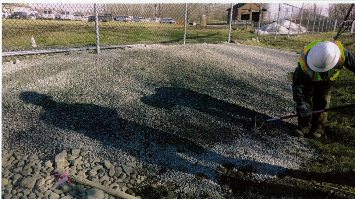
Photo 18: November 14, 2013. Facing Northeast. Additional gravel cover area complete.
