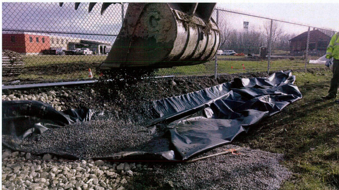
Photo 18: November 14, 2013. Facing Northeast. Known impacts area covered with geotextile fabric. Gravel cover in progress.
