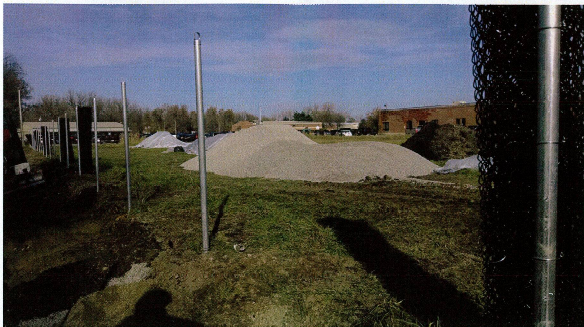
Photo 5: November 5, 2013. Facing Northeast. Gravel and drainage stone stockpile for backfill and cover. Plastic-covered stockpiles contain impacted materials.
