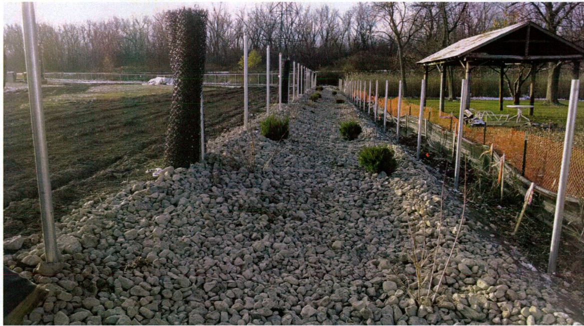
Photo 9: November 13, 2013. Facing South. Berm completed with most of ornamental stone placed. Plants planted according to planting plan.
