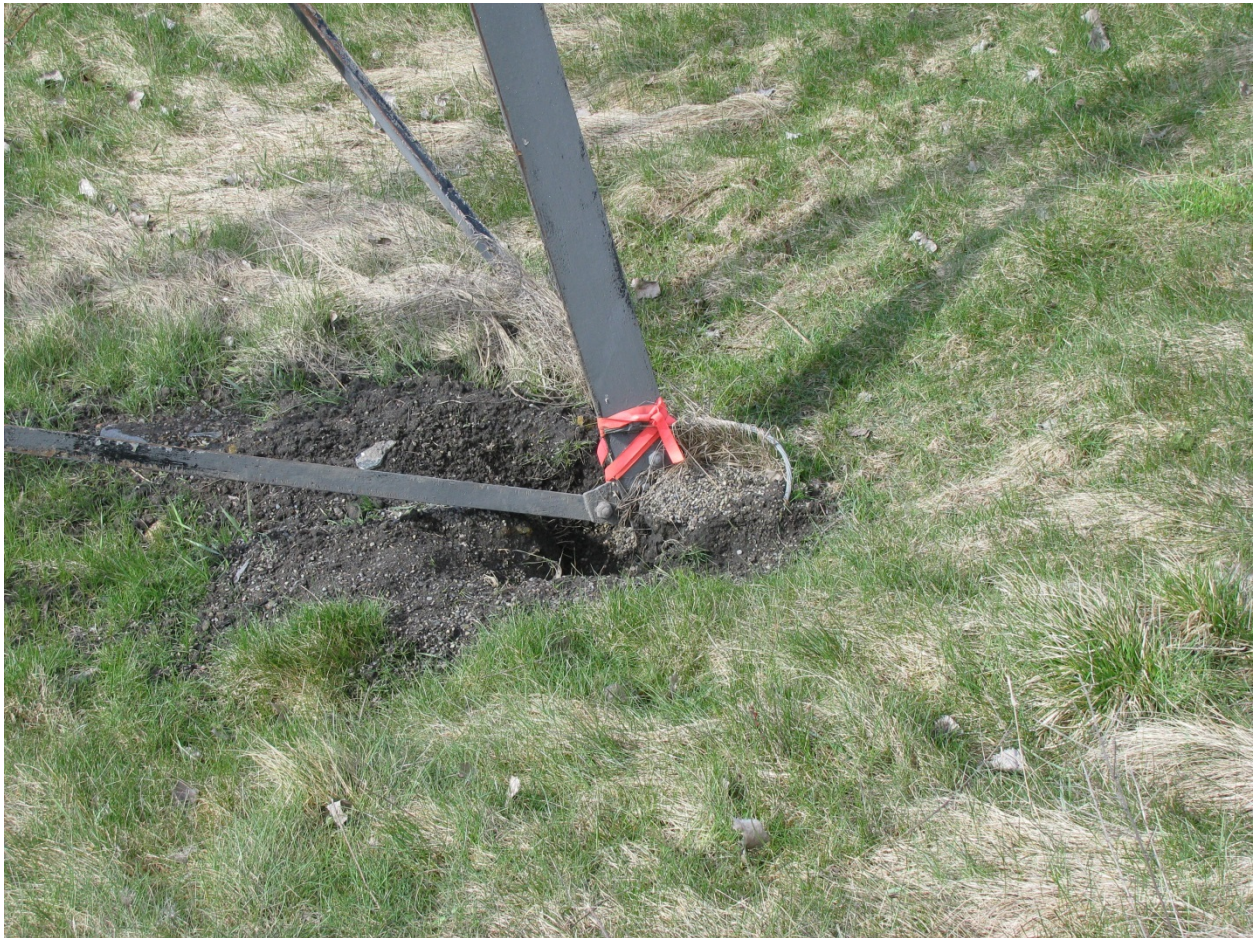
Animal burrow noted at the foot of the overhead transmission tower in the Clay Cap area.
