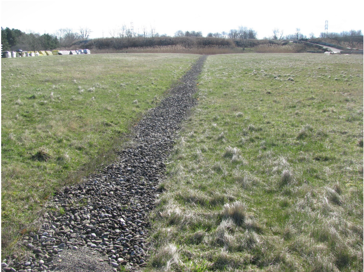
Looking east at French drain in Eastern Swale HDPE Cap (ESHC). Repairs made last year have been successful.
