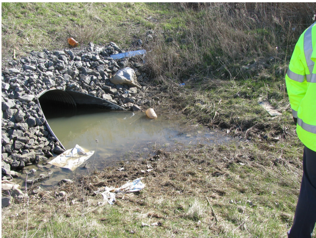
Looking east at small area of standing water at the outlet to the north culvert to the mid-section of the Eastern Drainage Ditch (EDD).
