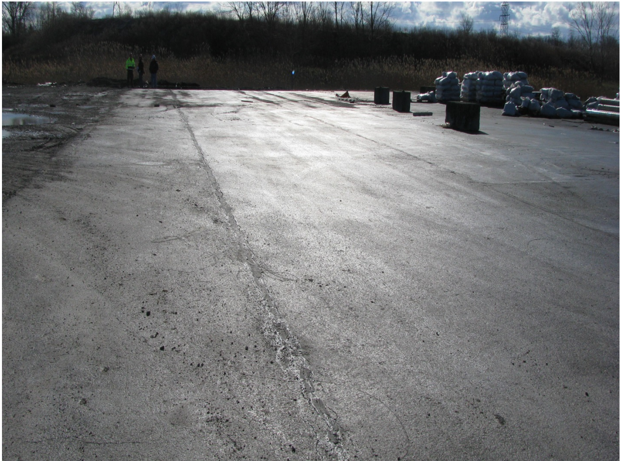
Looking east at Eastern Swale North Asphalt Cap (ESNAC), showing repairs made last year (2015).
