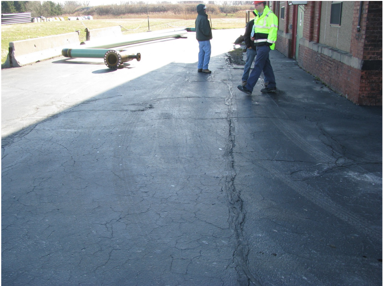
Looking east at the Building 10 Asphalt Cap (B10AC). Cracks in distance not fully penetrating the asphalt cap.
