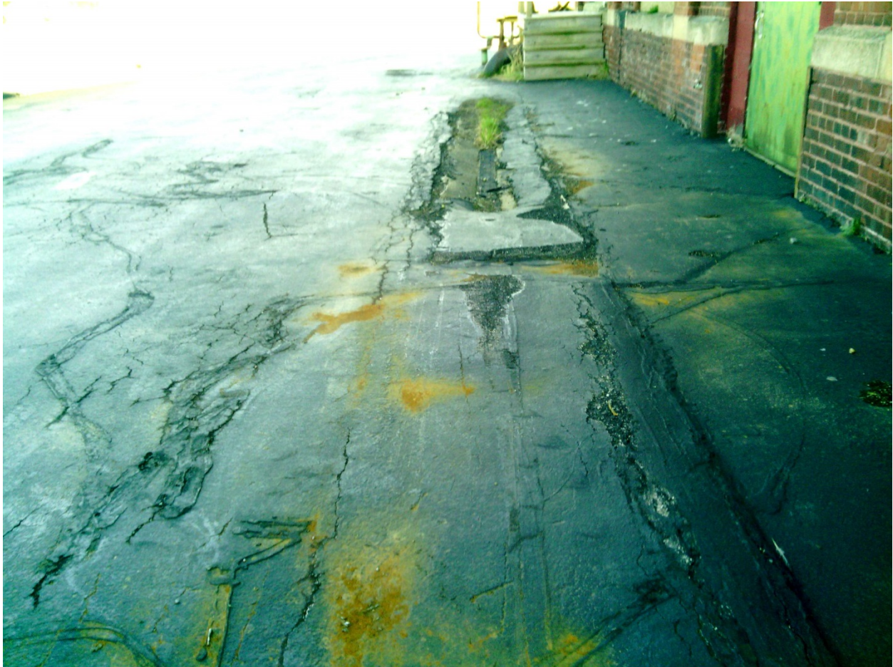
Look east at portion of the Building 10 Asphalt Cap (B10AC) observed with significant cracking that requires patching or repaving.
