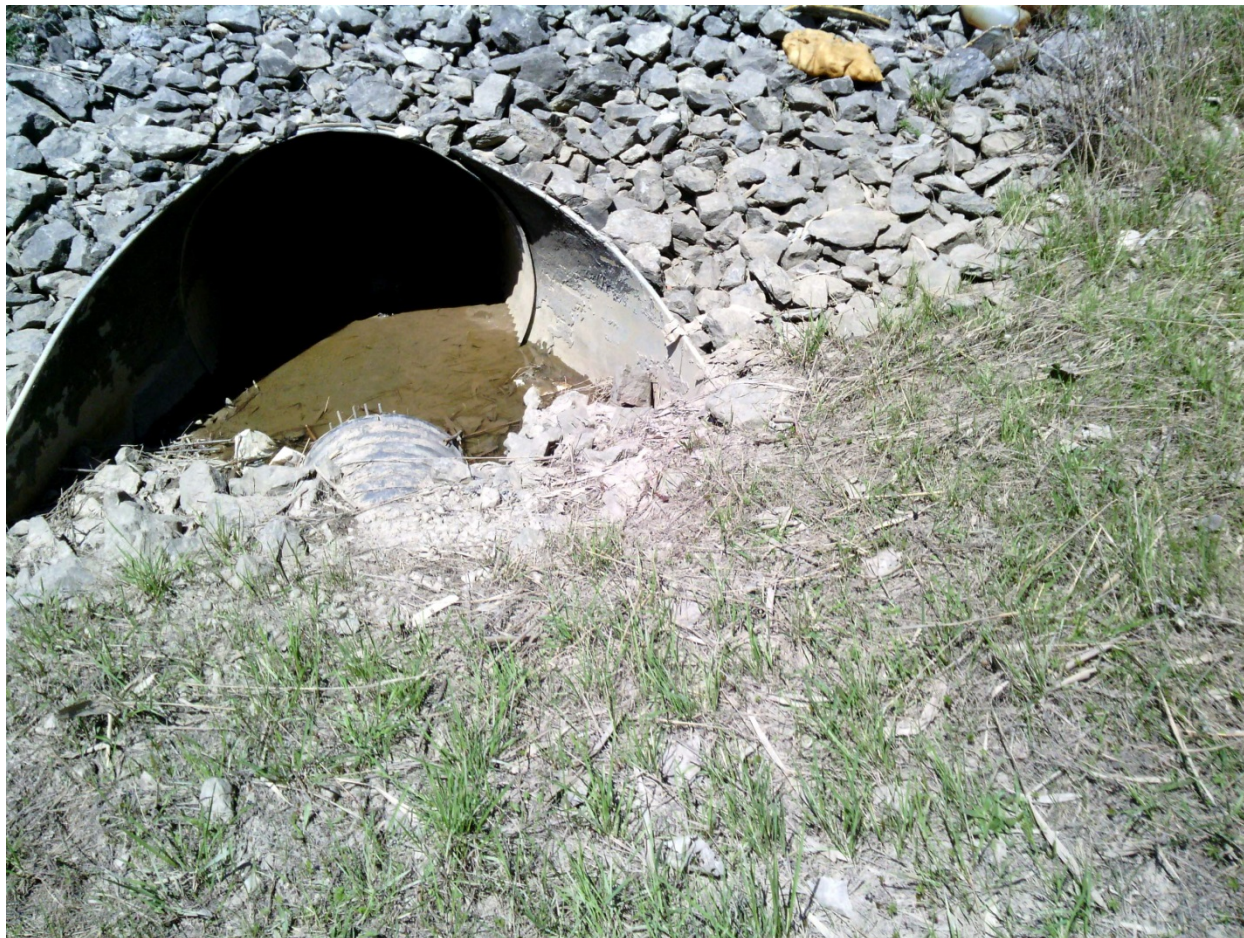
The outlet to the north culvert to the mid-section (HDPE cap) of the Eastern Drainage Ditch (EDD).
