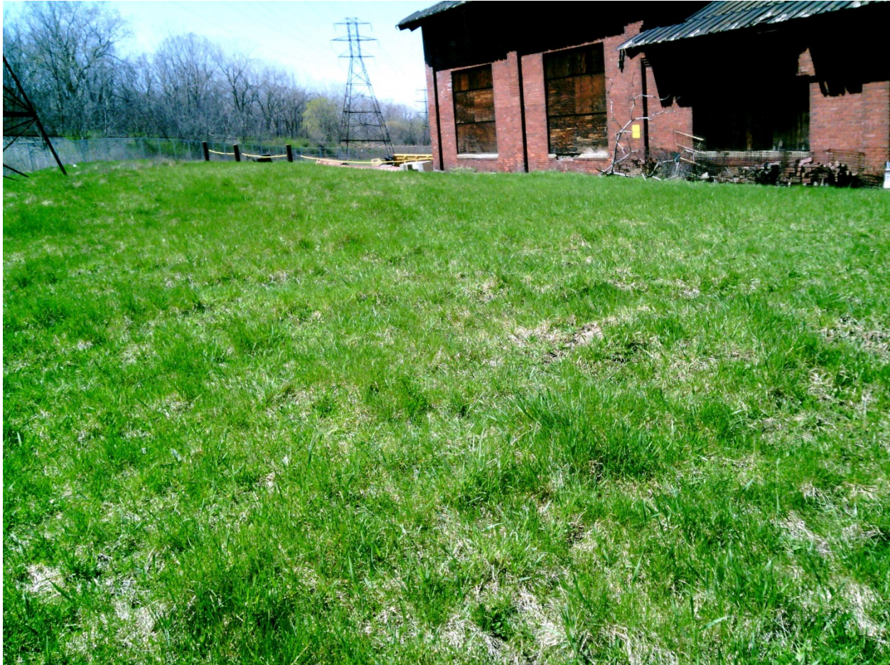
Looking west at the Clay Cap (CC) area. No issues noted. Animal burrow noted last year at the foot of the electrical tower (left edge of picture) has been filled.
