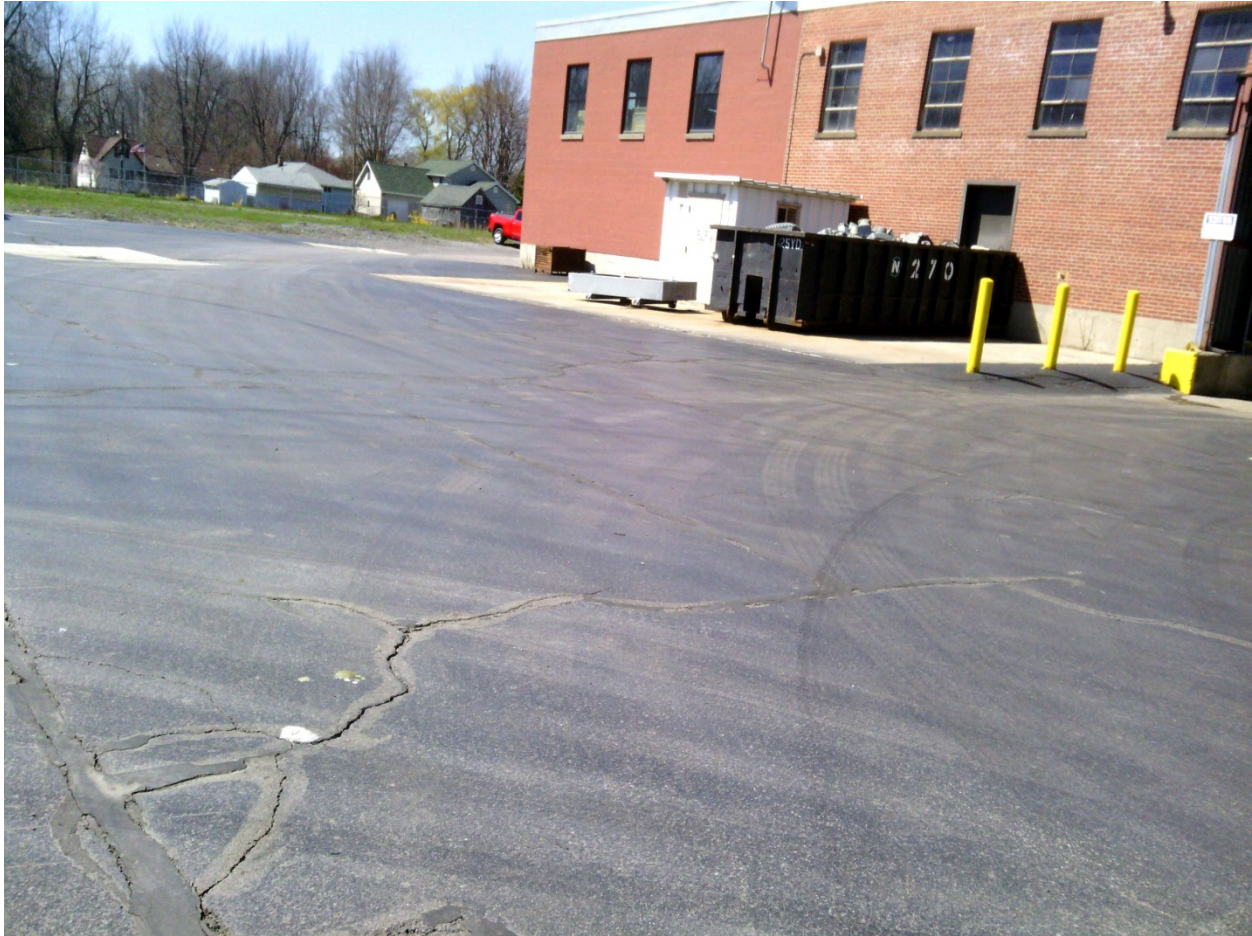
Looking northwest at a portion of the Building 3 South Asphalt Cap (B3SAC) showing an area with some significant cracking that needs to be sealed or patched.
