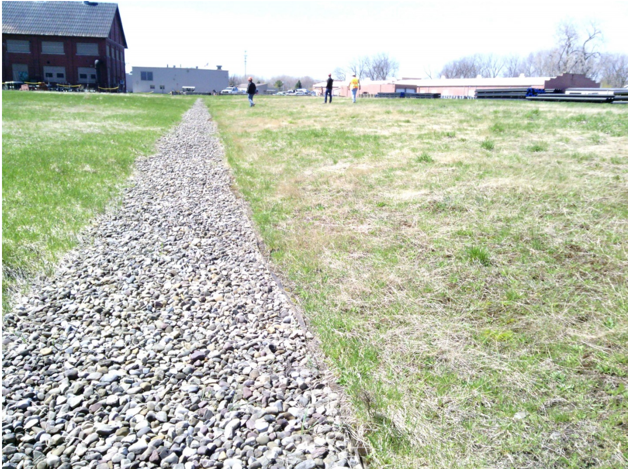
Looking west at French drain in Eastern Swale HDPE Cap (ESHC), in good condition.
