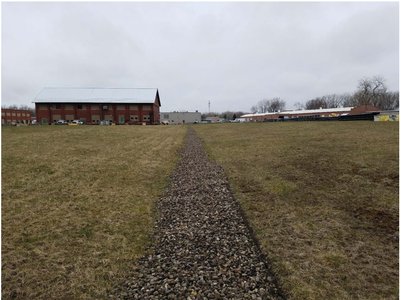
Photo 4. View looking west at French drain in Eastern Swale HDPE Cap (ESHC)
