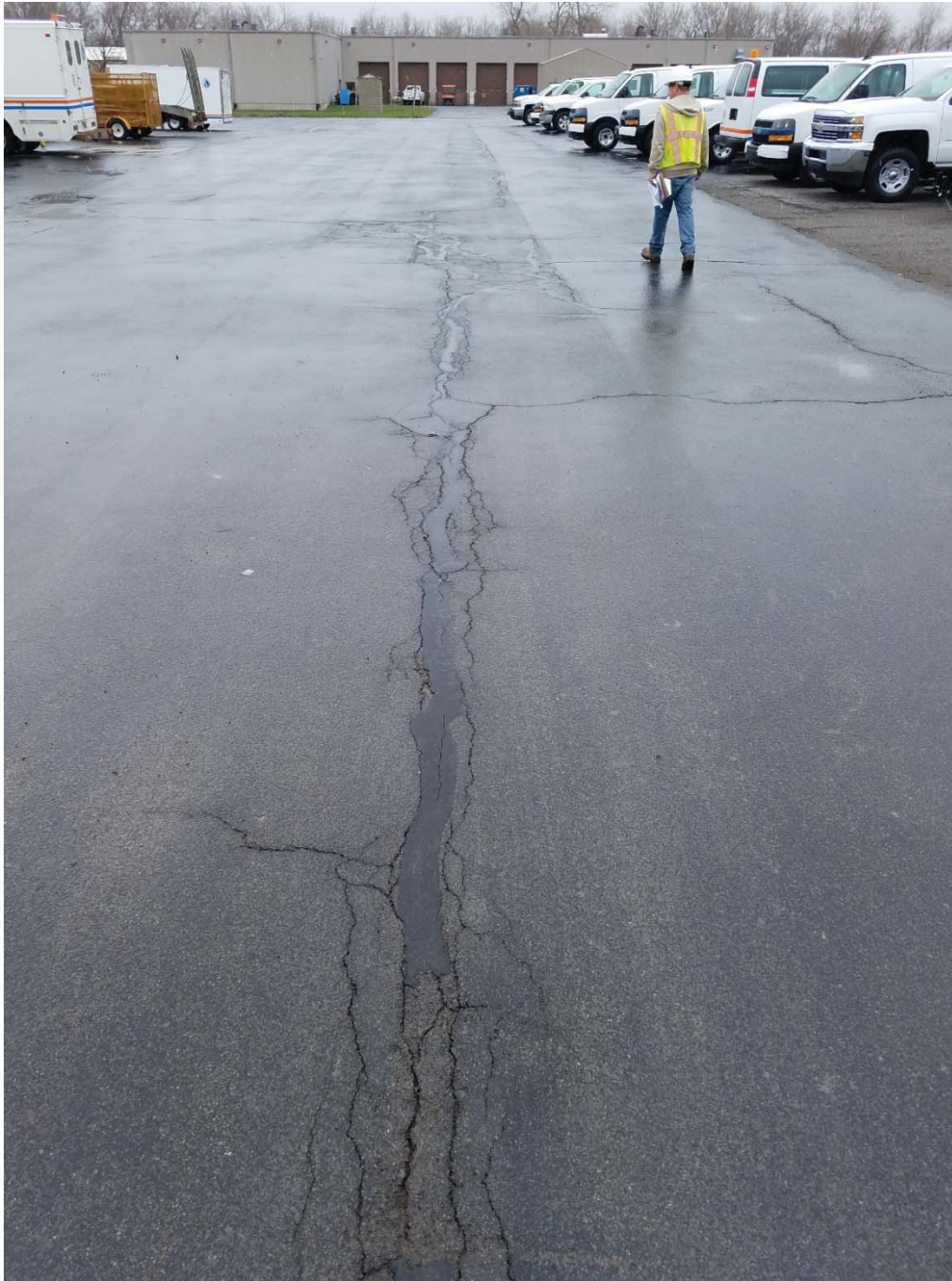
Photo 8. North view of Bldg. 3 East Asphalt Cap (B3EAC) with surface cracks and prior sealing.
