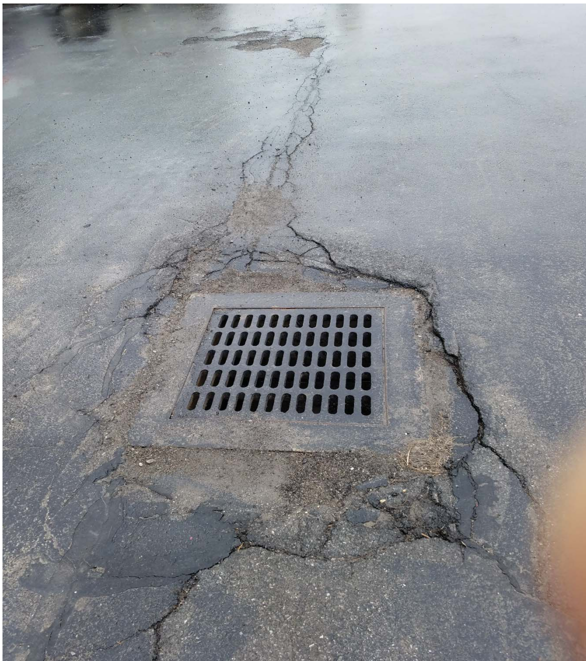
Photo 9. Building 8 West Asphalt Cap (B8WAC) cracking at storm sewer catch basin.
