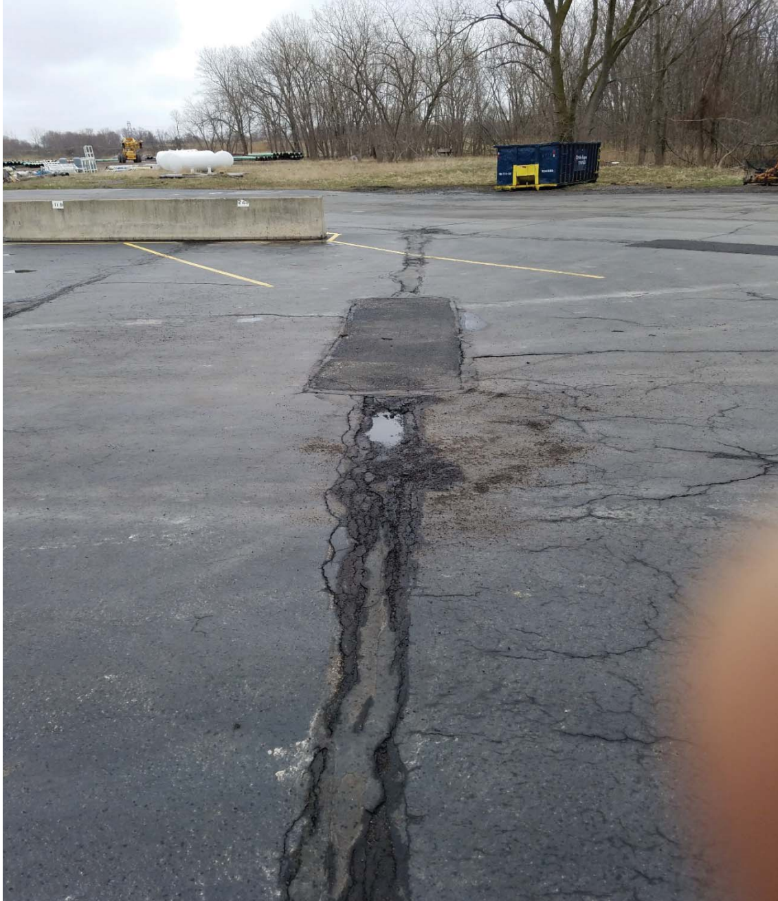
Photo 7. East view of Building 3 South Asphalt Cap (B3SAC). Surface cracks in sealant and some open to asphalt wearing course layer.
