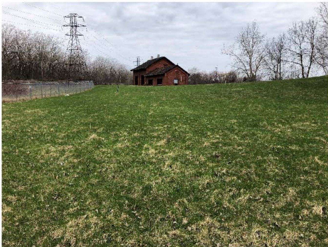
Photo 4. View looking west across clay cap in the area of Building 14.
