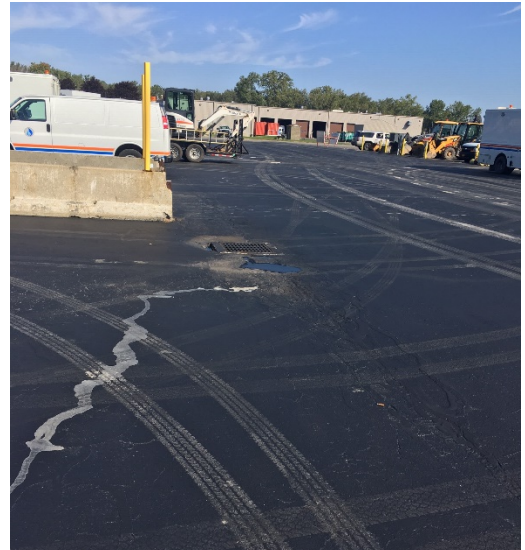
North view of repaired and resealed surface of the B3EAC.
