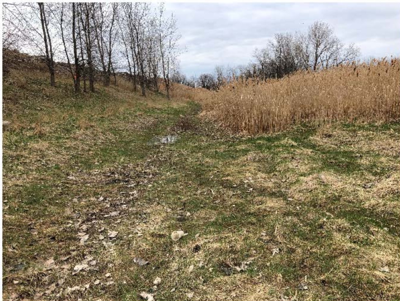
Photo 6. South view of East Drainage Ditch HDPE.
