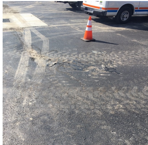
Repairs and sealing of the B8WAC near the concrete catch basin apron.
