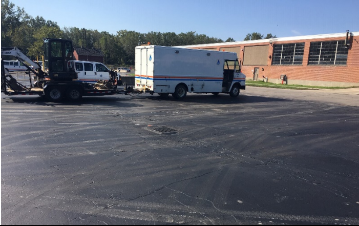
Southwest view of repaired and re-sealed surface of the B3EAC.
