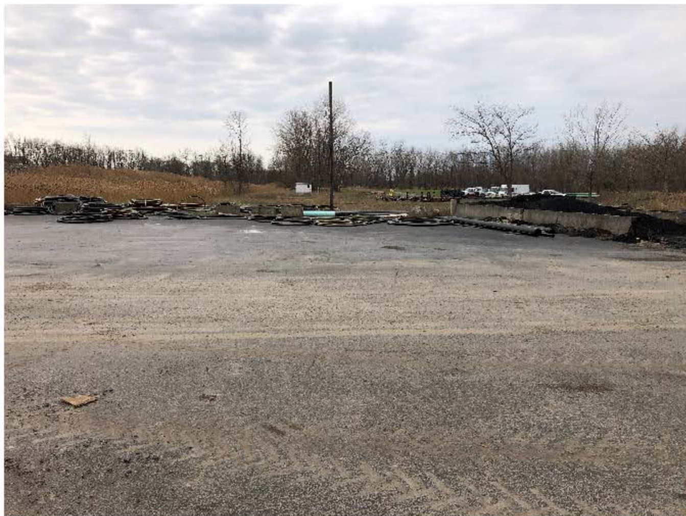
Photo 9. Southeast view at Eastern Swale South Asphalt Cap (ESSAC).
