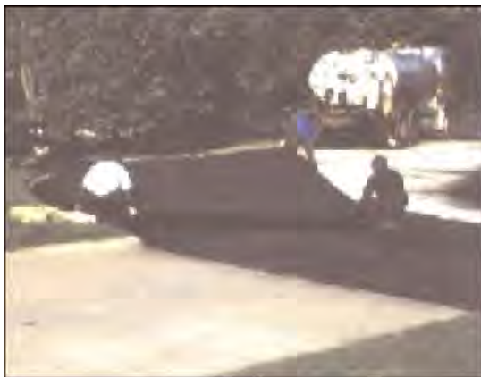
Figure 8 PETROMAT PLACEMENT AROUND CURVES
