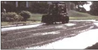
Photograph of broadcasting asphalt on Petromat.
