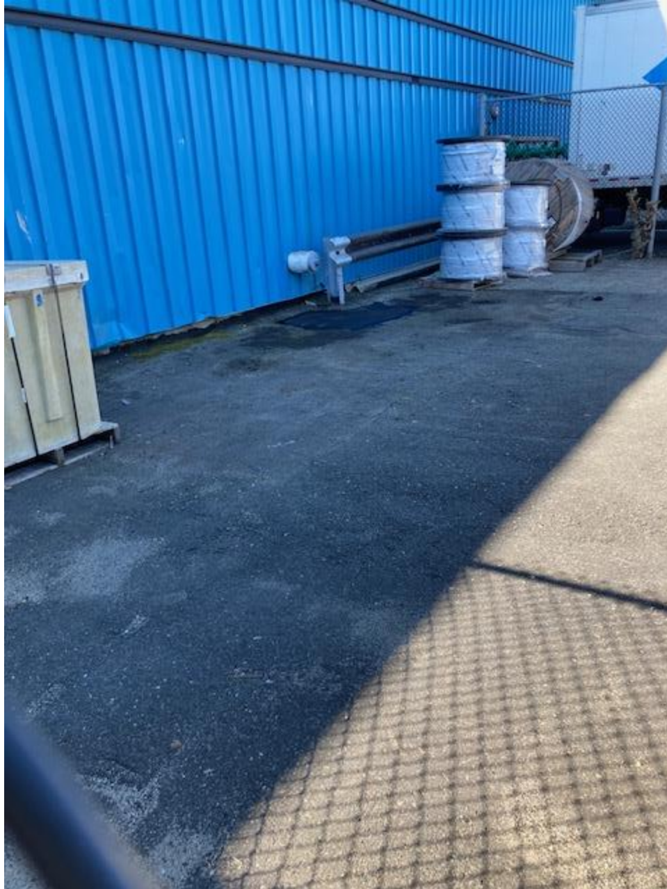
Photo 2: Former Jet Test Pads Detail
