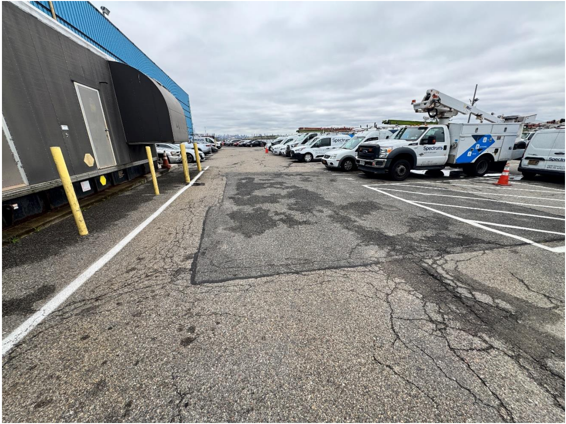
Former UST Area
