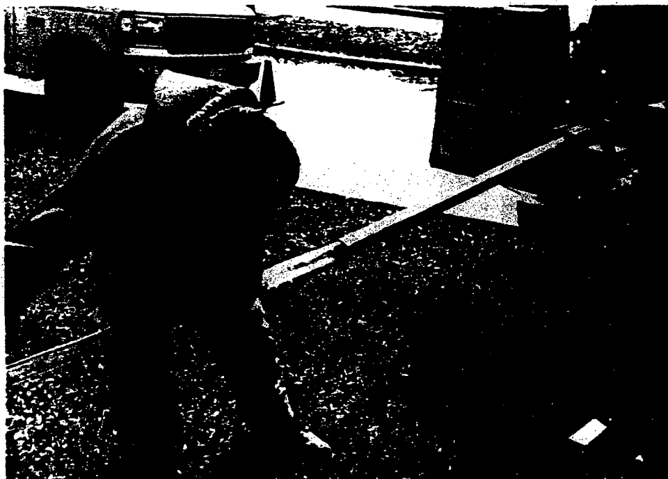
Photo #1 – Boring Location No. 43 northeast corner of Site Building (Installation of clean plastic sampling sleeve into Geoprobe MacroCore).
