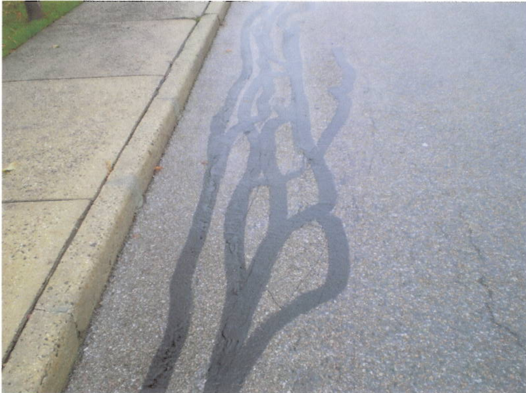
Sealed Pavement Cracks, Western Driveway, Repaired Spring 2008.
