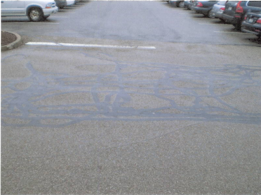
Sealed Pavement Cracks, Southwest Driveway, Repaired Spring 2008.
