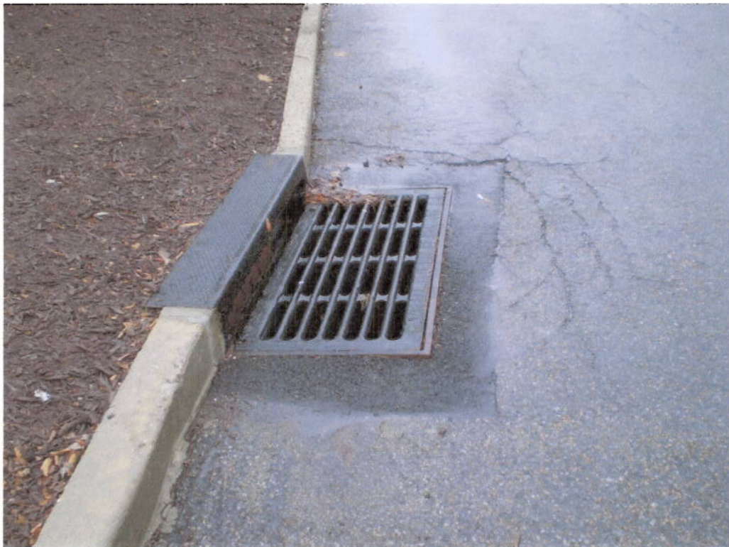
Catch Basin Repaired, Northern Parking Lot.
