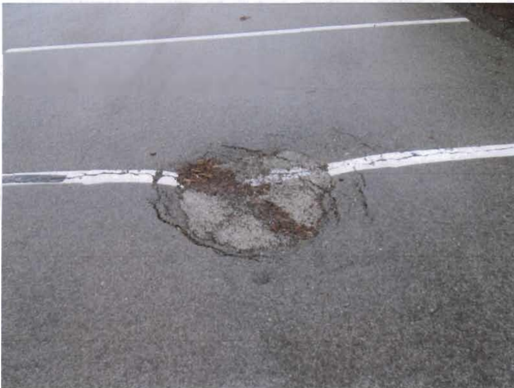
Parking Lane 1, south side building, approximately 2-foot diameter sink-hole, base layer intact, repair in Spring 2014.
