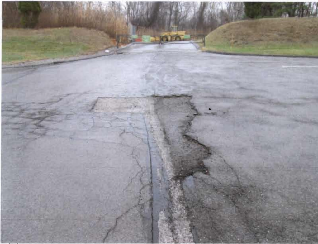
Southeast corner of parking lot, top layer peeling (10-feet by 18-inches), base layer intact, to be repaired in Spring 2014.
