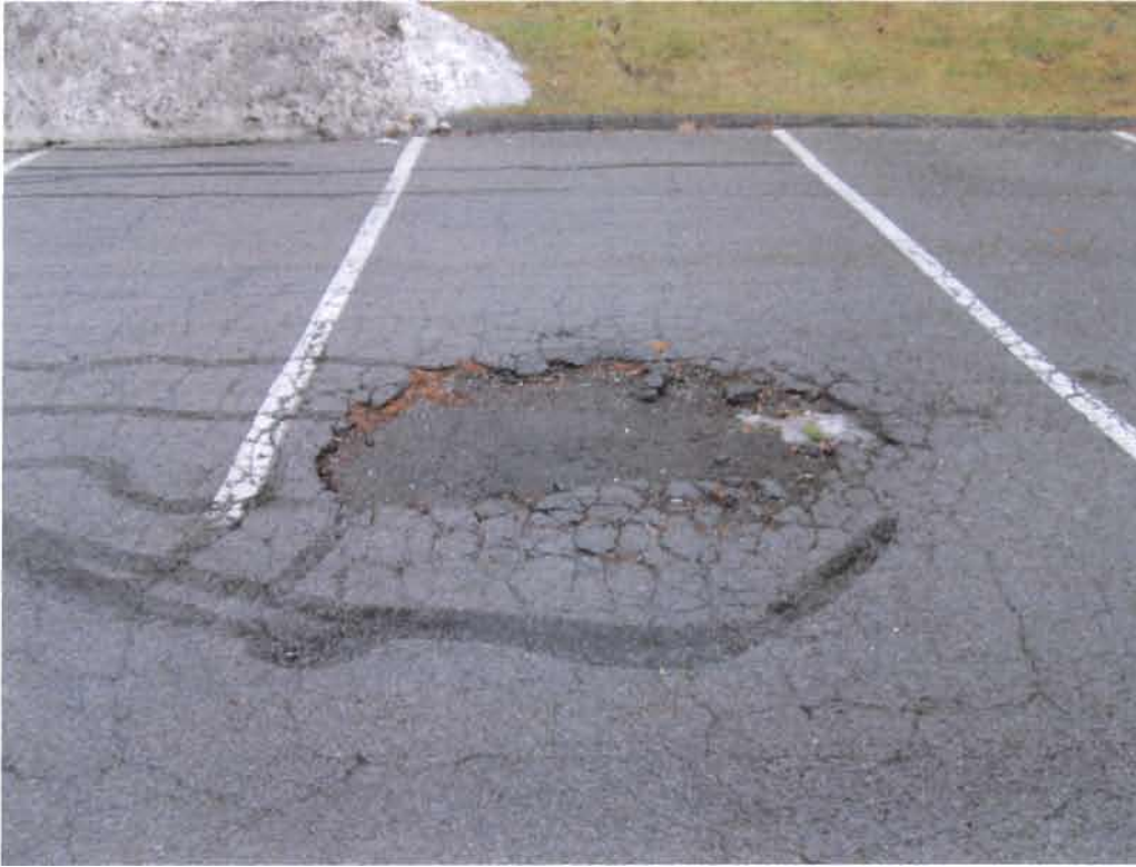
3-foot diameter repair area at south end Parking Lane 6, south side building, to be repaired in Spring 2014. Base layer intact.
