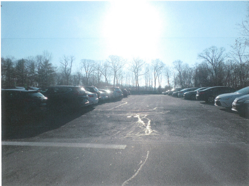
1 st row of asphalt paved parking South, small cracks in asphalt, none below top course.
