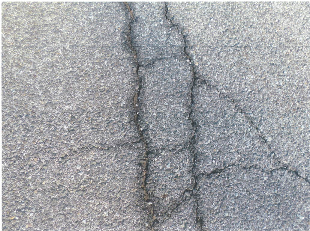
Typical crack in top layer of asphalt.
