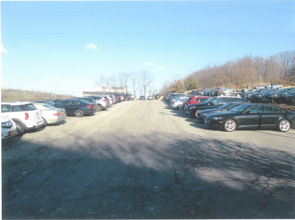
2 nd row of asphalt paved parking North, small cracks in asphalt, none below top course.
