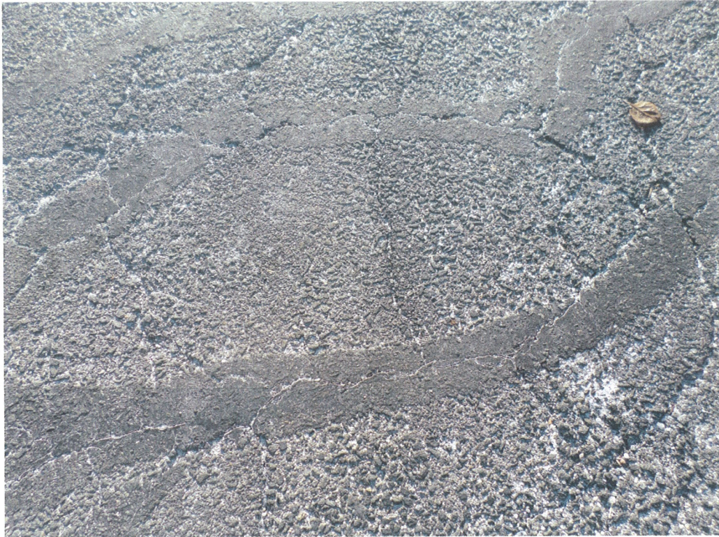
Typical small cracks in 1 st course of asphalt, none in 2 nd course of asphalt pavement.
