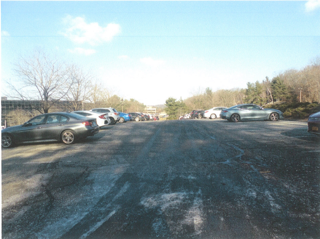
6 th row of asphalt paved parking South, small cracks in asphalt, none below top course.
