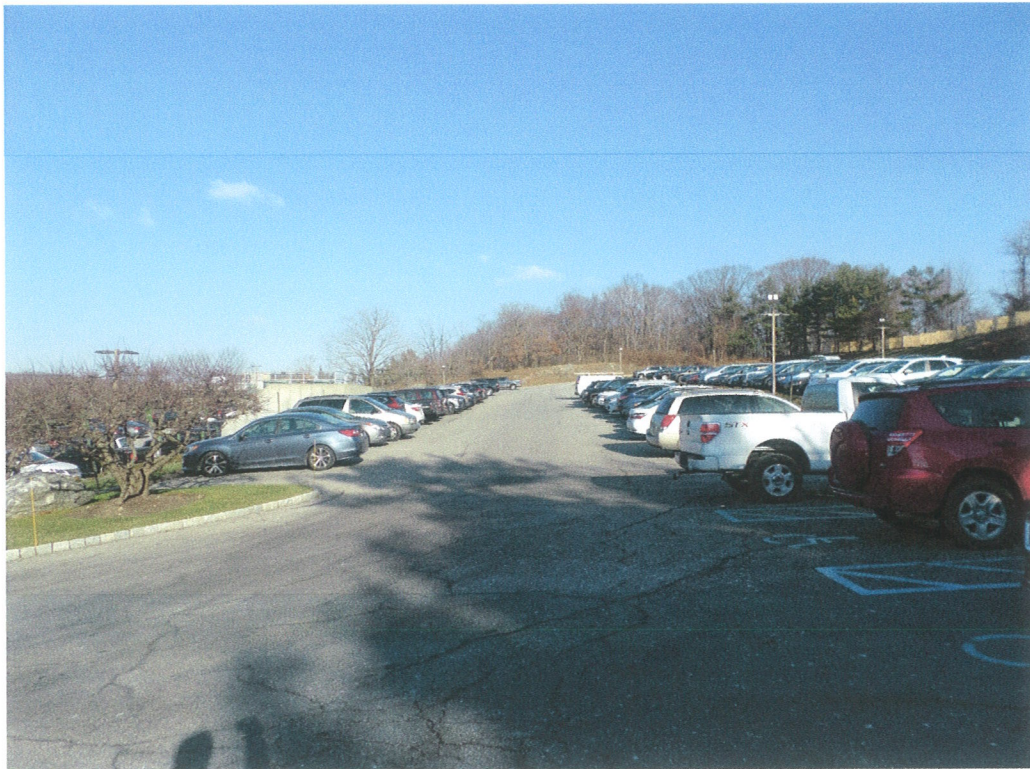
4 th row of asphalt paved parking North, several cracks in asphalt, none below top course.
