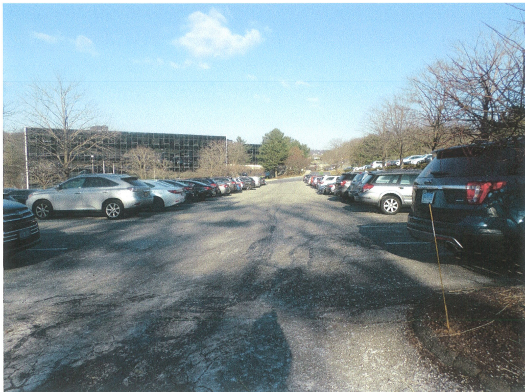
5 th row of asphalt paved parking South, small cracks in asphalt, none below top course.
