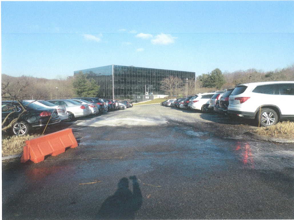
3 rd row of asphalt paved parking South, small cracks in asphalt, none below top course.
