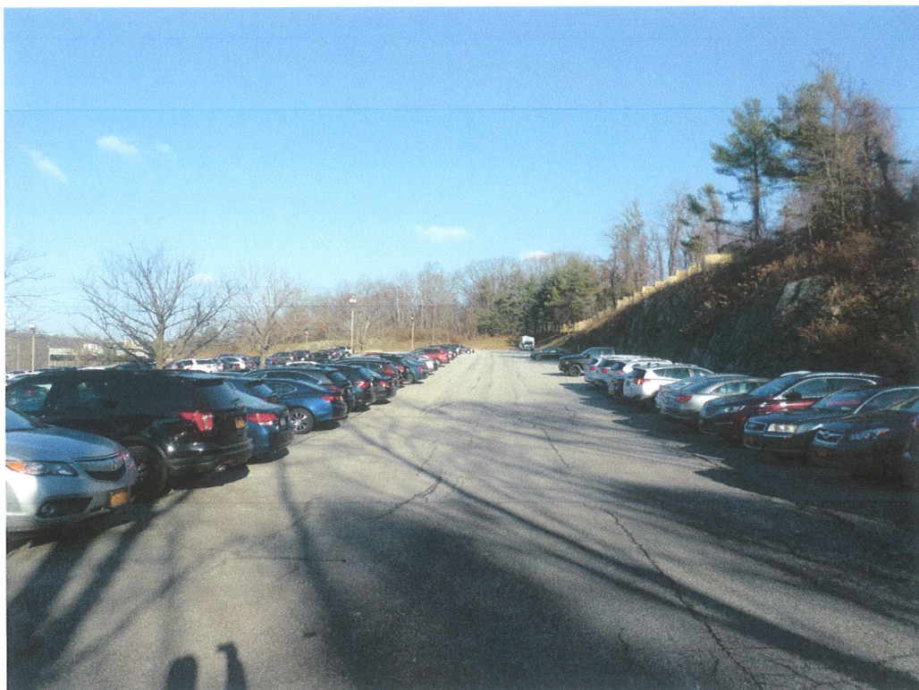
6 th row asphalt paved parking North, small cracks in asphalt, none below top course.
