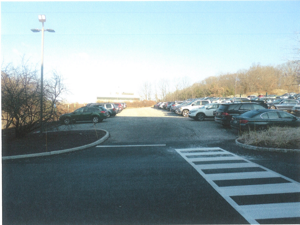
1 st row of asphalt paved parking North, small cracks in asphalt, none below top course.
