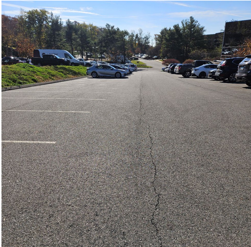
Photograph 9: Typical parking lot crack, facing south
