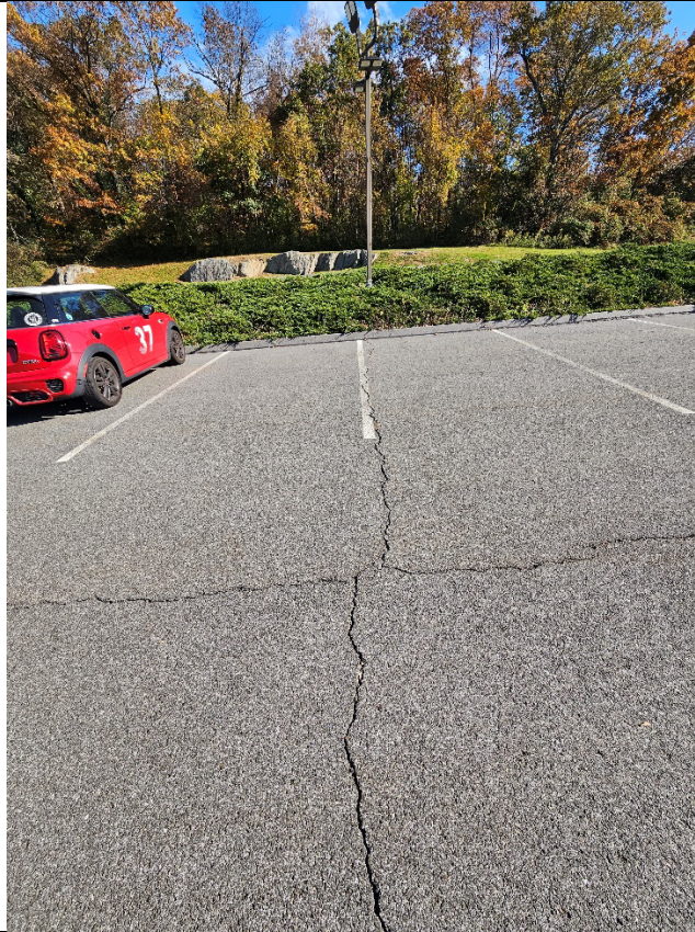
Photograph 11: Typical parking lot crack, facing east
