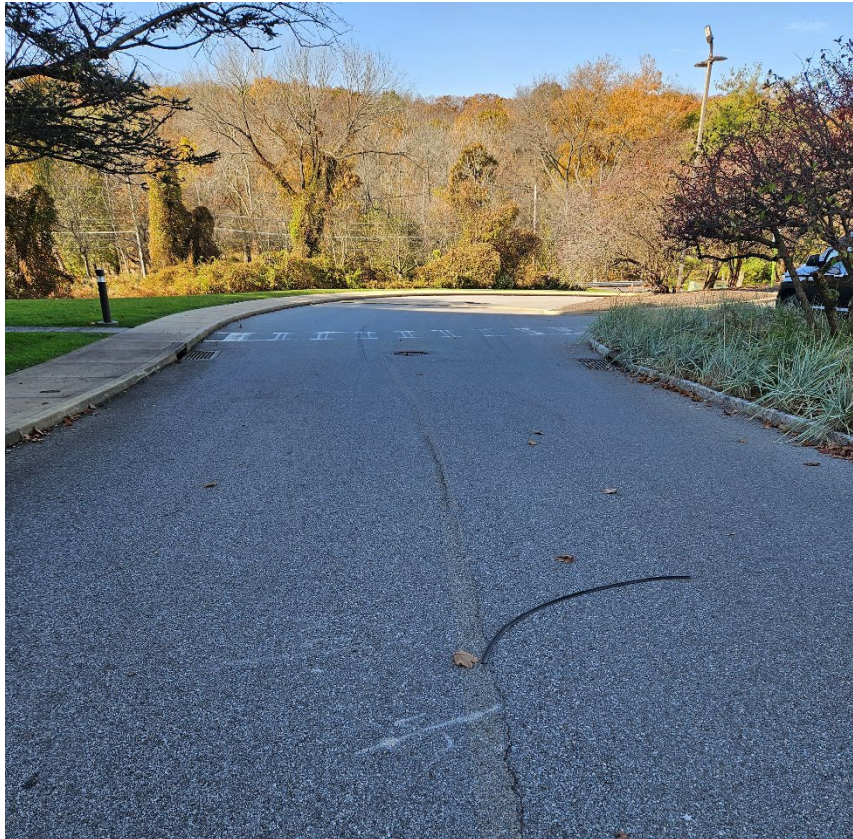
Photograph 7: Typical driveway shallow cracking, facing west
