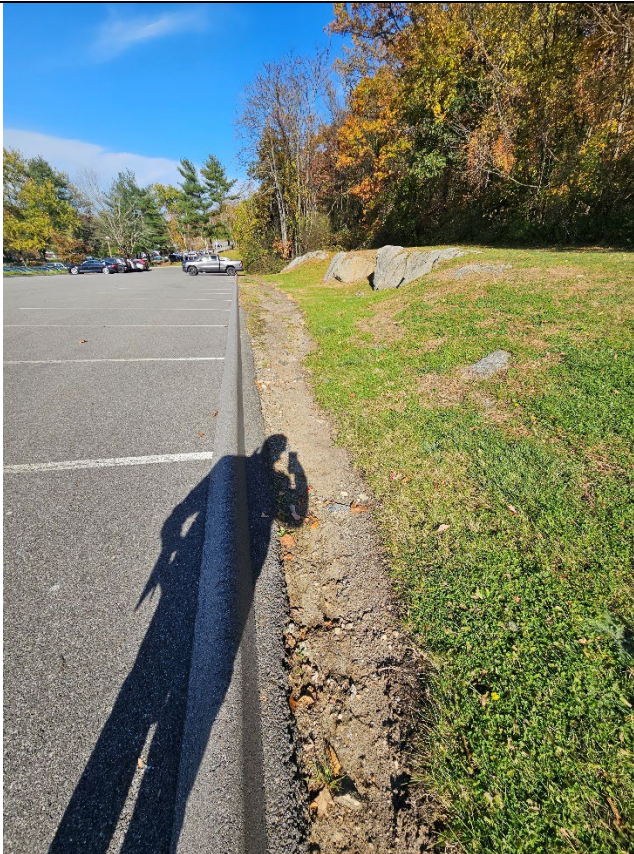
Photograph 12: Erosion and washout, facing north
