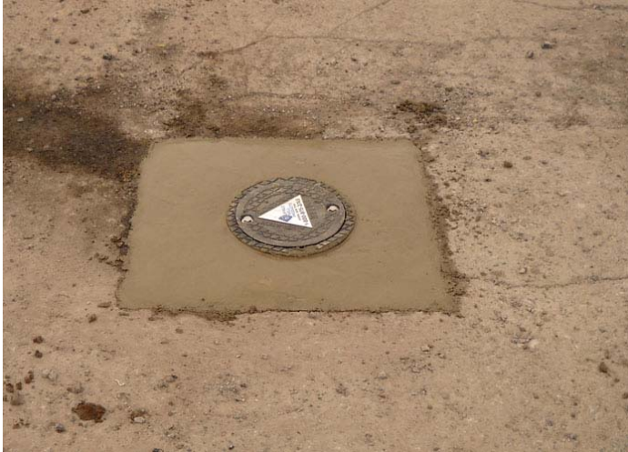
Repaired Monitoring Well Casing – MW-1
