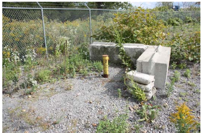
Monitoring Well MW-4
