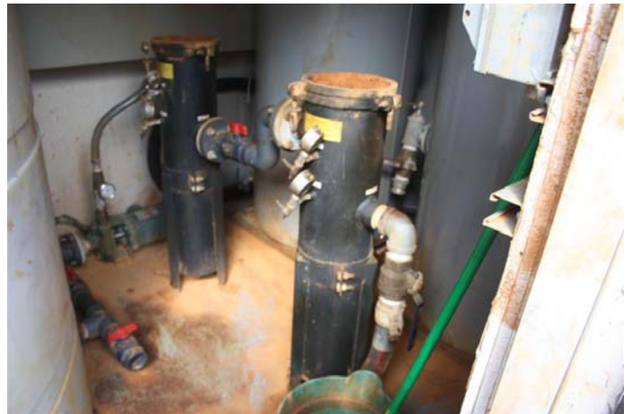
Interior of HVE Shed
