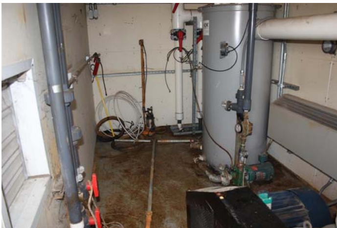
Interior of HVE Shed
