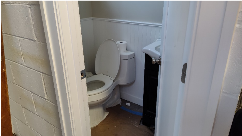
Photograph #104 – View of plumbing warehouse bathroom.
