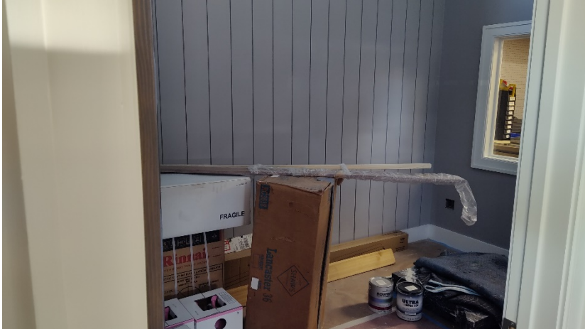
Photograph #101 – View of plumbing warehouse side room (future office space).
