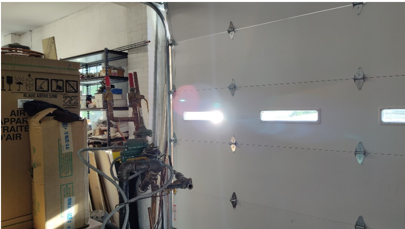
Photograph #99 – View of plumbing warehouse garage door.
