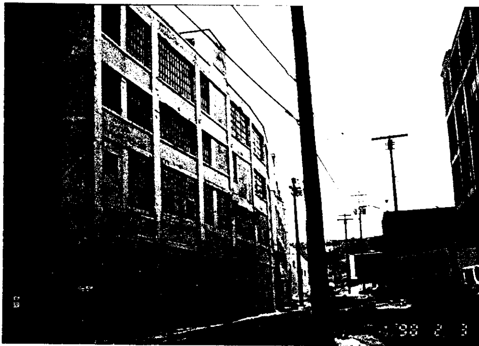
Photograph of the northeast corner of the main facility building, taken looking west. February 3, 1998.
