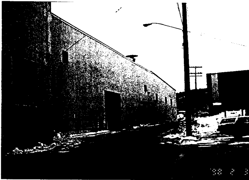
Photograph of the northwest portion of the north side of the main facility building, taken looking west. February 3, 1998.
