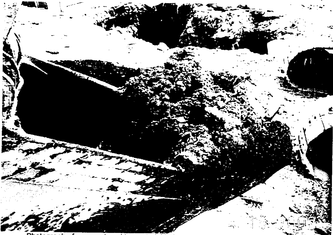
Photograph of apparent coal tar material being separated for later off-site disposal.
