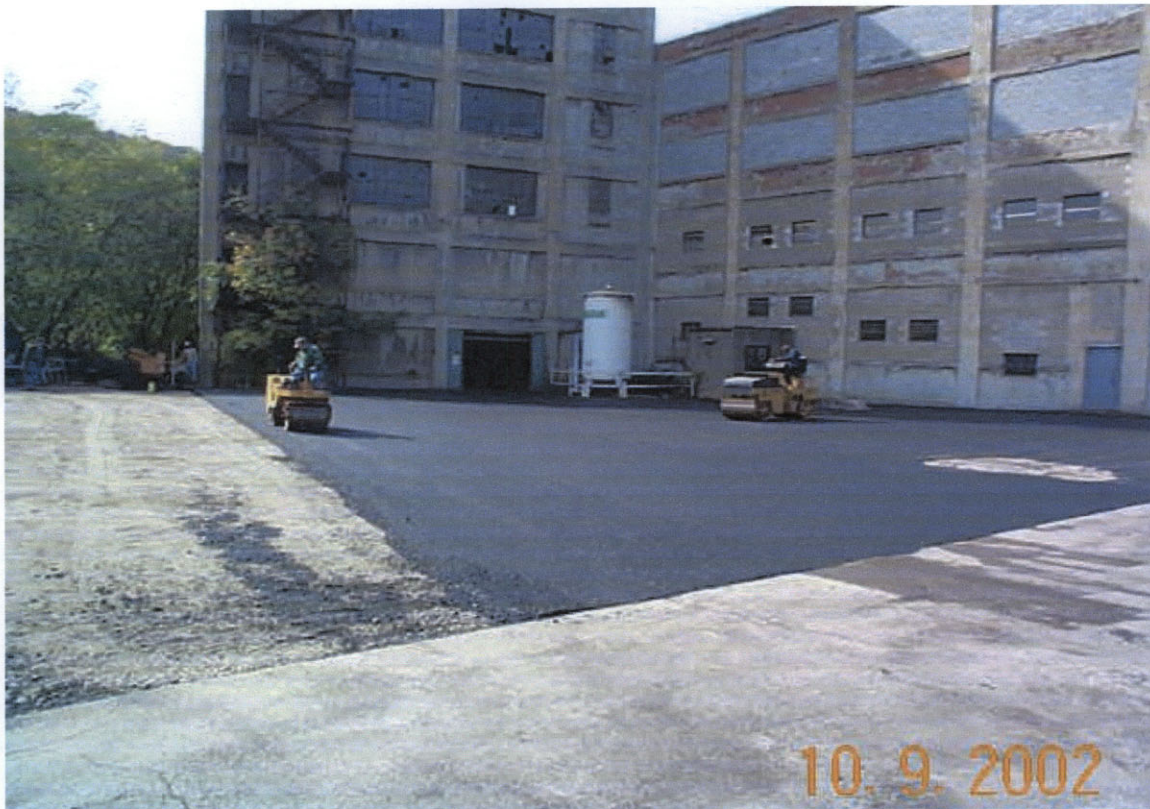
Photograph of paving activities in northeast portion of SPX property over chromium-contaminated soils.
