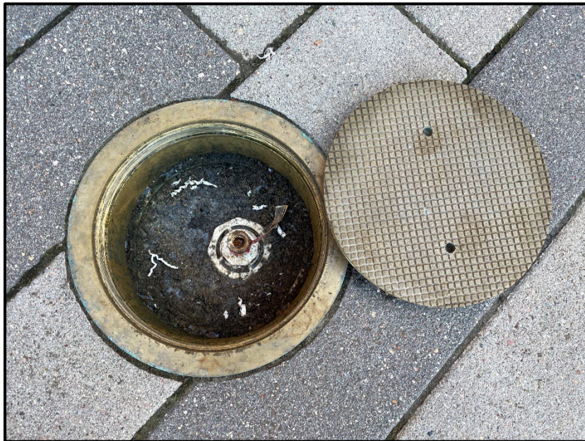
Photo 36. SSDS inspection: vapor monitoring point MP-2.
