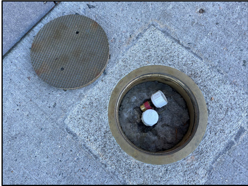
Photo 35. SSDS inspection: vapor monitoring point MP-1.
