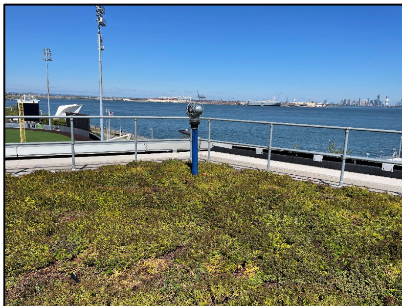
Photo 40. SSDS inspection: roof vent VR-1.
