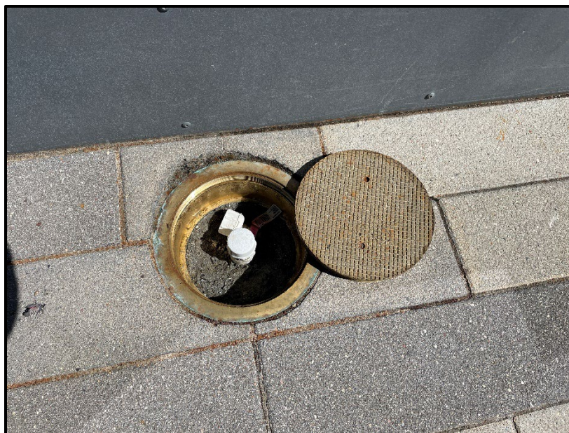
Photo 39. SSDS inspection: vapor monitoring point MP-6.
