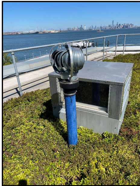
Photo 41. SSDS inspection: roof vent VR-2.
