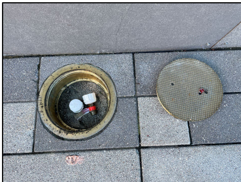
Photo 38. SSDS inspection: vapor monitoring point MP-5.
