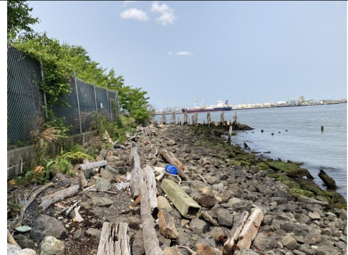
Photo 30: Remains of a former timber sheet pile wall supported by large quarry stones along western wooded Site area. Retains shoreline stone/gravel covered area and protecting shoreline.
