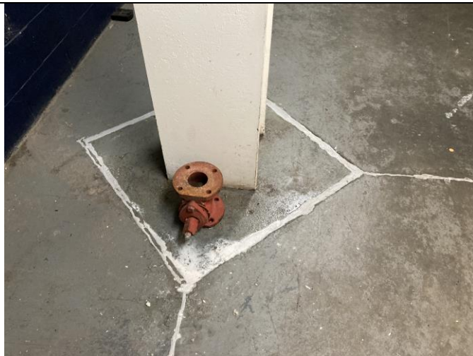
Photo 39: Resealed concrete slab floor crack in main hallway (1).
