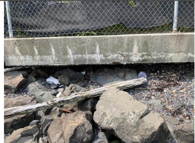
Photo 24: Undermined shoreline bulkhead wall at western end of NY Wheel construction Site.
