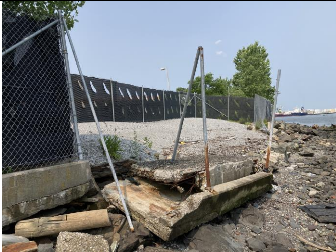
Photo 25: Collapsed shoreline bulkhead wall at western end of NY Wheel construction Site (1).
