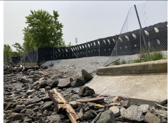
Photo 26: Collapsed shoreline bulkhead wall at western end of NY Wheel construction Site (2).
