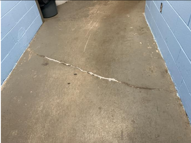
Photo 41: Resealed concrete slab floor crack in main hallway (3).
