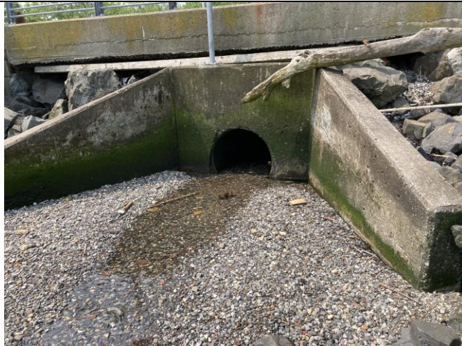
Photo 19: Site stormwater outfall from the central retention basin. Outlet is partially blocked with gravel.
