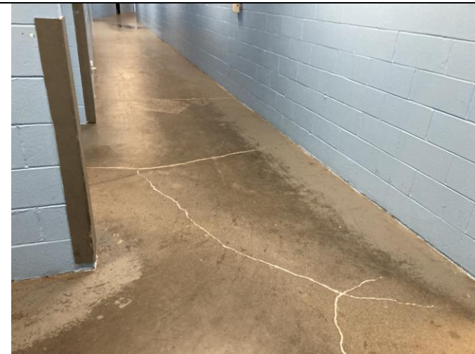
Photo 40: Resealed concrete slab floor crack in main hallway (2).
