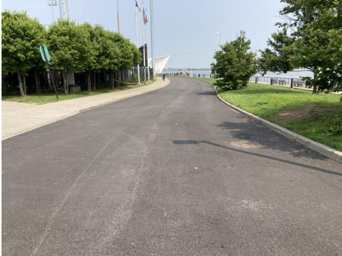
Photo 9: Repaved roadway to repair surface cracking between right field stadium wall and shoreline (looking northwest).
