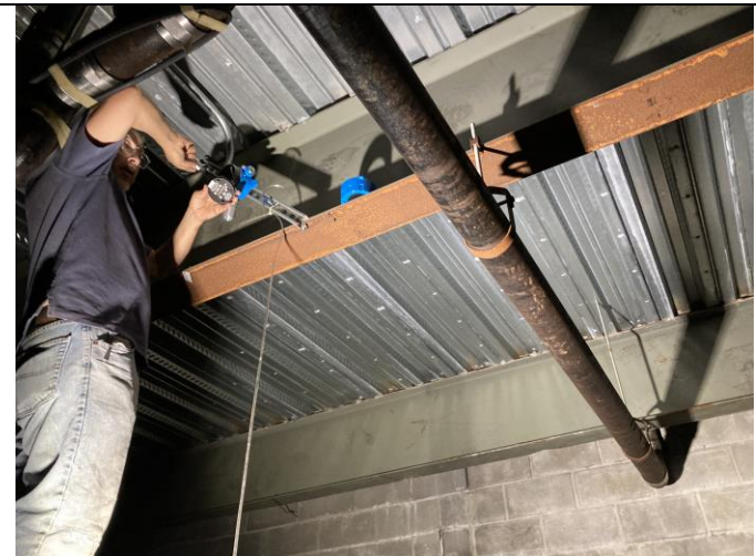
Photo 44: Replacement of gas survey sensor in right field storage area.
