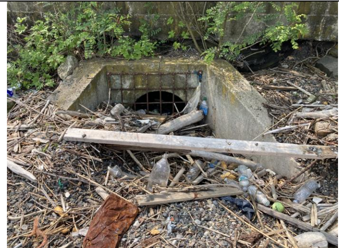
Photo 28: Partially blocked NYCDEP sewer outfall along shoreline at western end of NY Wheel construction Site.
