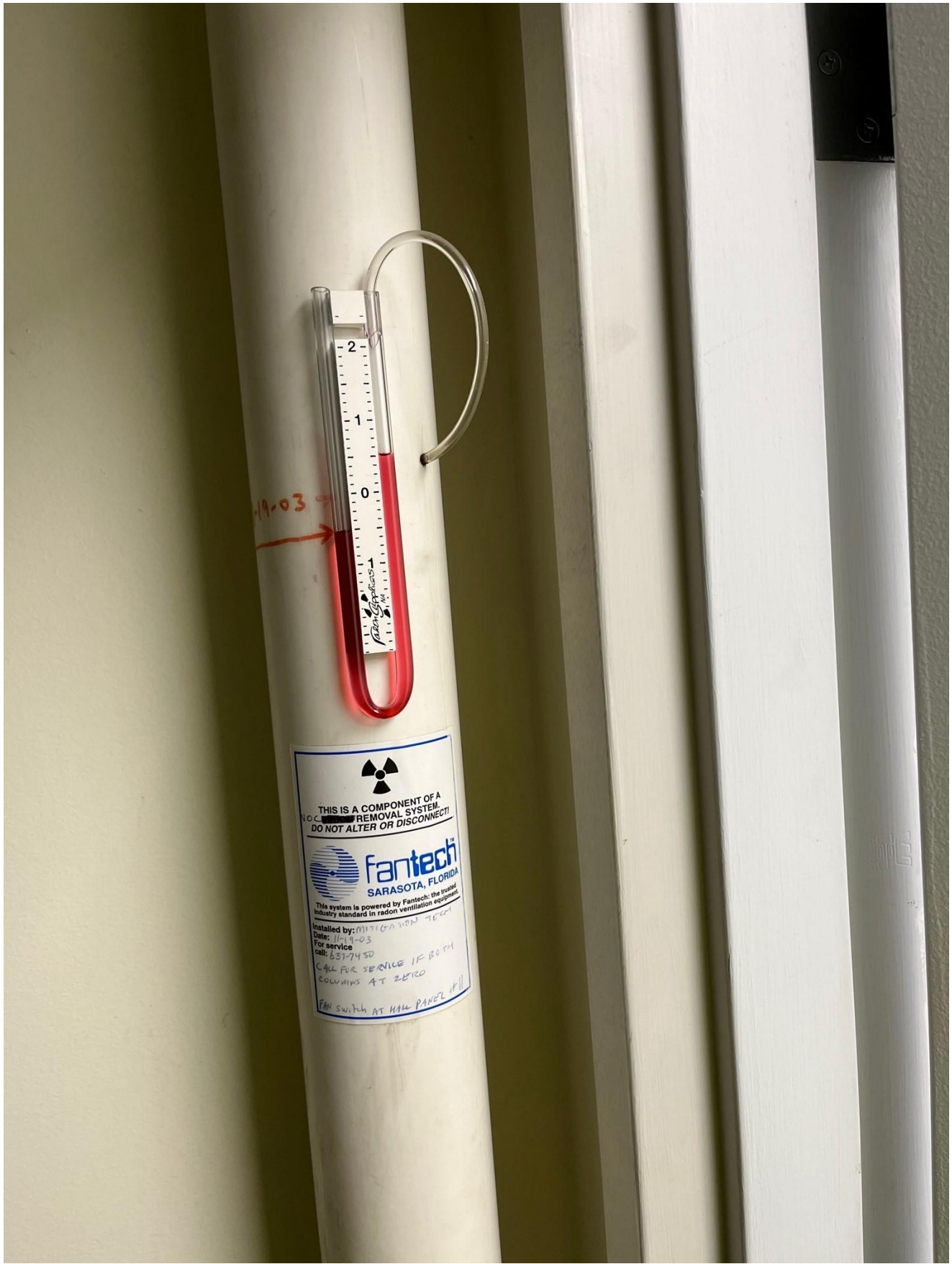
Sub-Slab Depressurization System April 29, 2022
