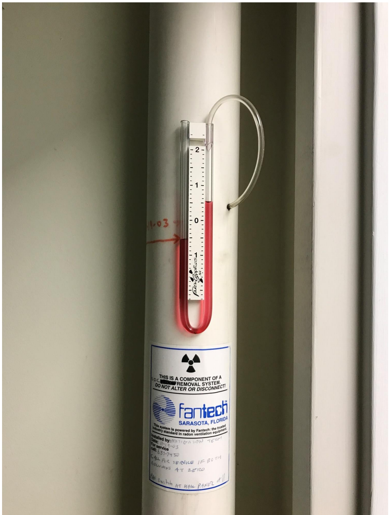
Sub-Slab Depressurization System September 10, 2021
